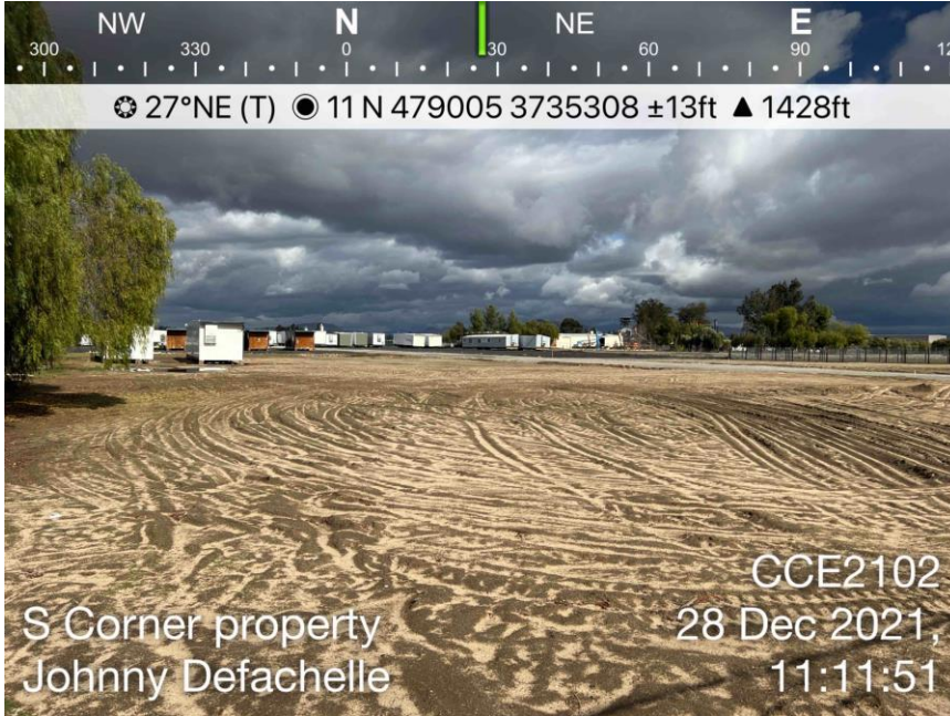
Photo 1: Overview of Project Site (View Northeast)
