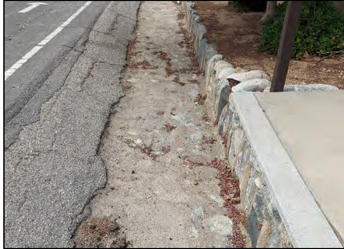
Figure 8. Overview of NB-004 (view west; August 18, 2022).
