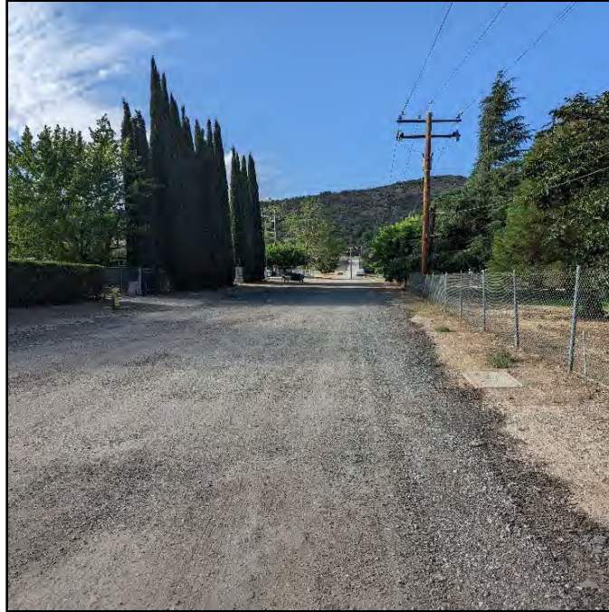
Figure 11. Overview of NB-007 (view south; August 18, 2022).
