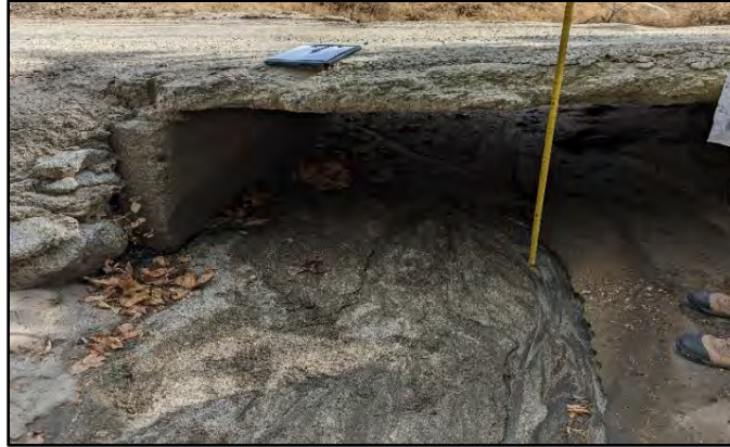
Figure 5. Overview of NB-002 (view northeast; August 18, 2022).
