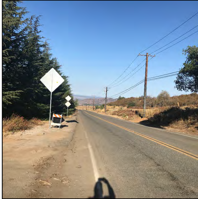
Figure 9. Overview of NB-005 (view southwest; August 18,2022).
