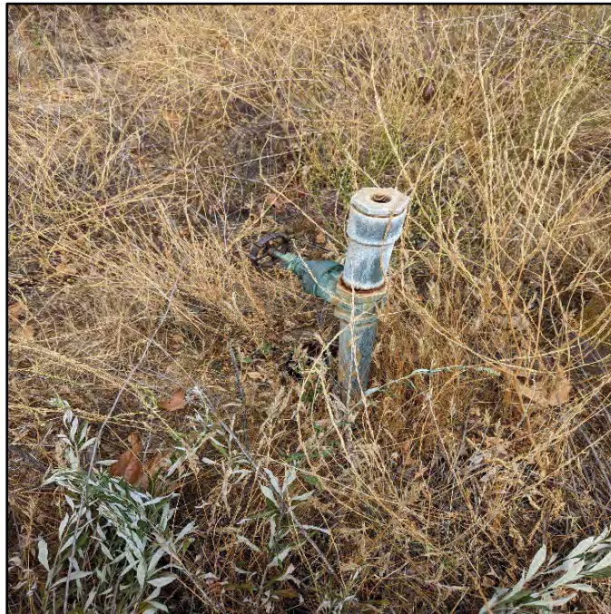
Figure 7. Feature 3 of NB-003 (view detail; August 18, 2022).
