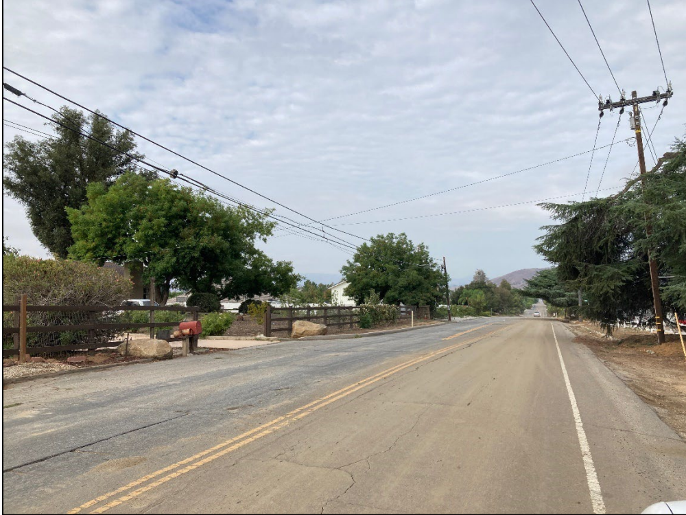
Photo 3. Project site with developed land cover along western end of the alignment on Oak Glen Road between Cherry Croft Drive and Pendleton Road, facing southwest.
