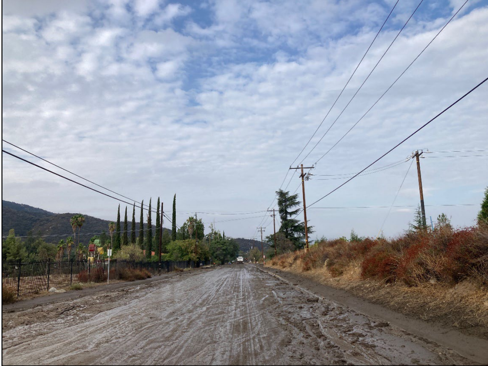
Photo 7. Project site along the public ROW (Oak Glen Road) with evidence of recent mudslide at the time of survey; photo taken northeast of Chagall Road, facing southwest.
