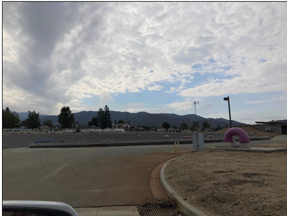
Photo 2. Existing YVWD water facility at the proposed location of 14.1 booster site; facing east.
