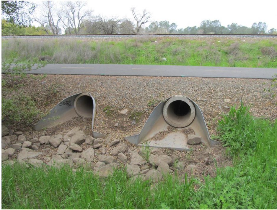
Photo 5: The storm drain culvert in the Bike Path alignment.
