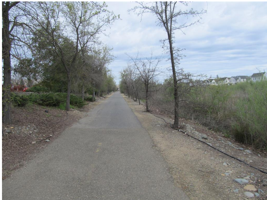
Photo 6: The Bike Path alignment looking north from Parkshore Road.
