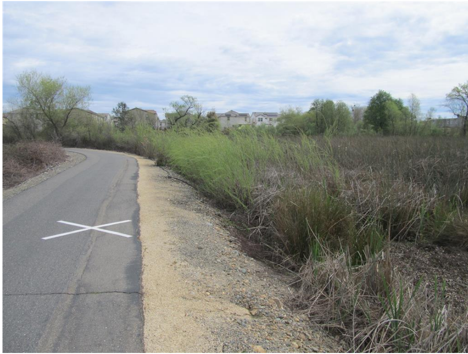
Photo 7: The Bike Path alignment south of Parkshore Road.
