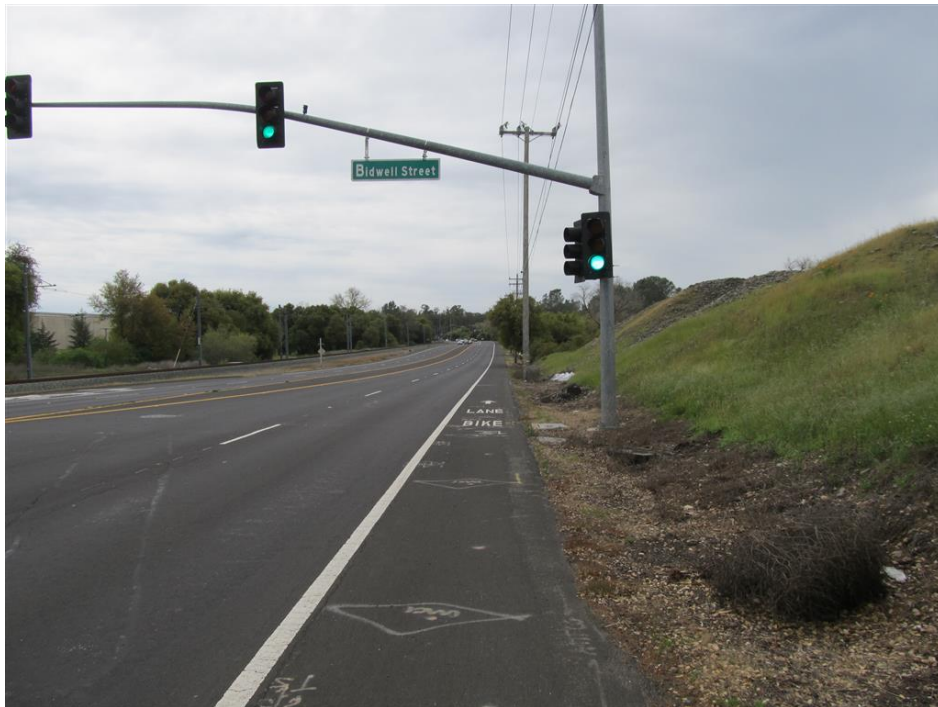
Photo 1: The north end of the Folsom Boulevard alignment, looking south.
