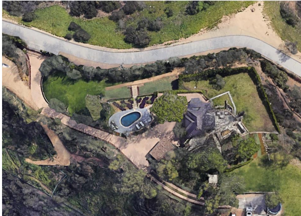
Figure 3 – Location of Pool To Be Removed, Retaining Wall #3 and Fill-Sites (DEIR Figure II-1 Detail) In Relation to Historic Residence
