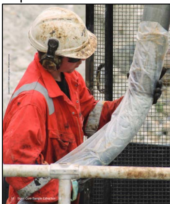
Figure 7. Sonic Core Sampling Extraction (Boart Longyear, 2017)
