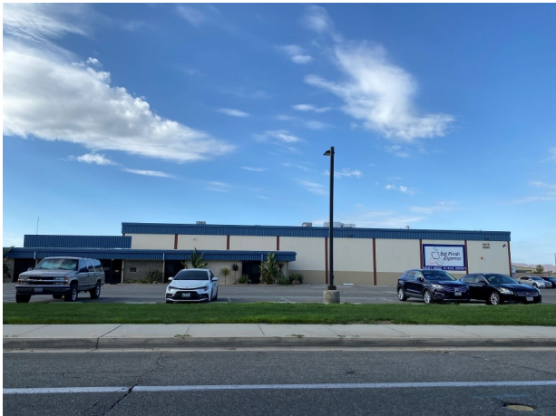
17. View of the adjoining property to the north.
