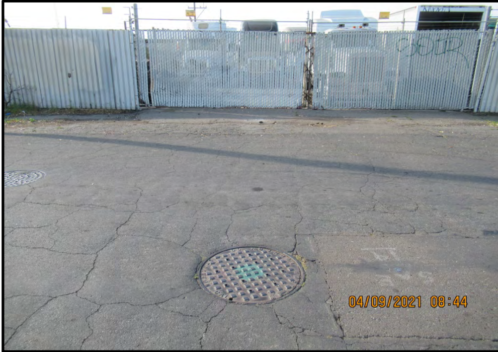
Man hole within Anderson Street, looking south; 04/09/21.
