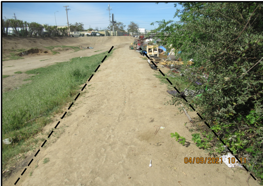
Top of the underground culvert system shown in the photo above, looking west from just downstream of the culvert inlet; 04/09/21.
