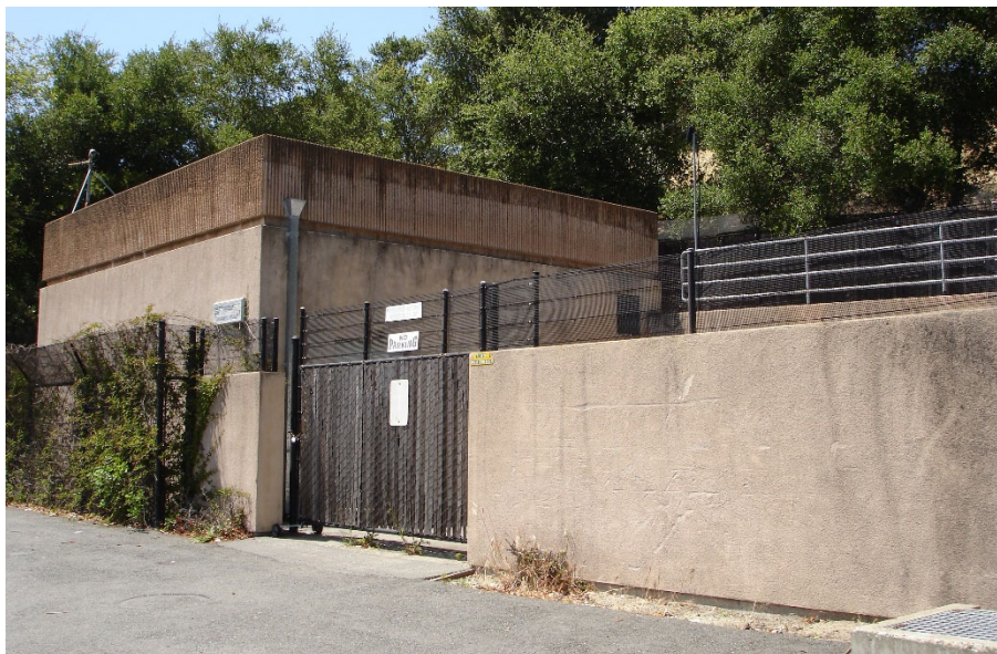
Example Installation of CMU Wall
