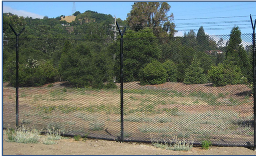
Example Installation of Security Chain Link Fence
