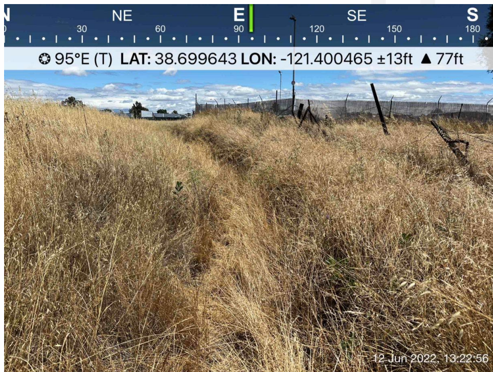
Figure 4 – Stormwater drainage along southern boundary
