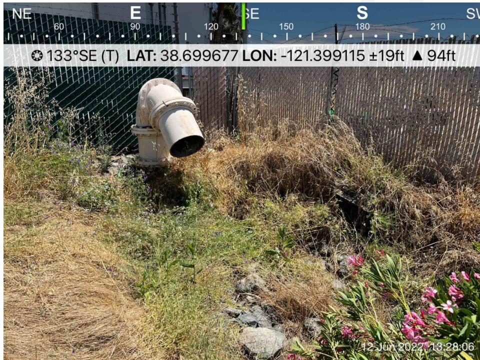
Figure 6 – Stormwater drainage pipe in SE corner of Project boundary
