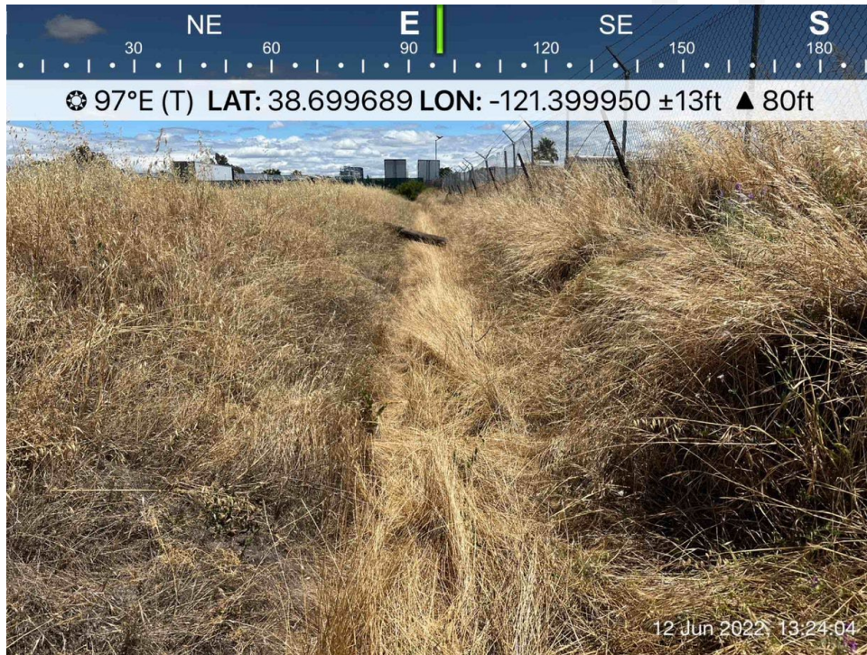
Figure 5 – Stormwater drainage view east
