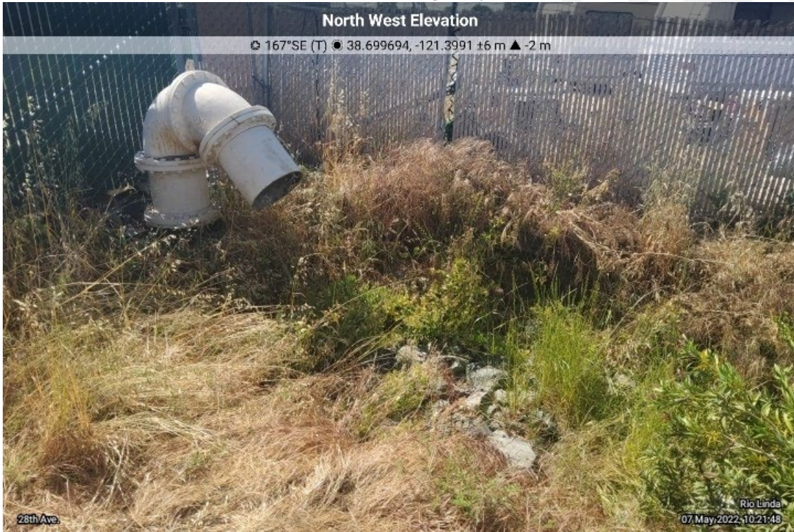
Photo 10 – Stormwater Drainage Pipe (View Southeast)
