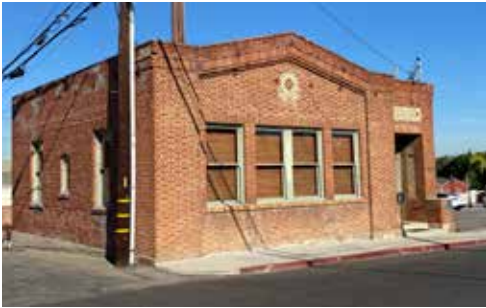
203 Richmond Street was the former location of the first El Segundo City Hall and Library
