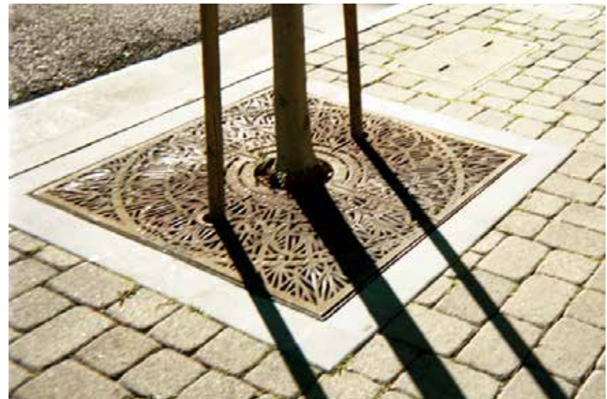
Tree grates should be used to expand the usable pedestrian space and create a distinct sense of place and urban character
