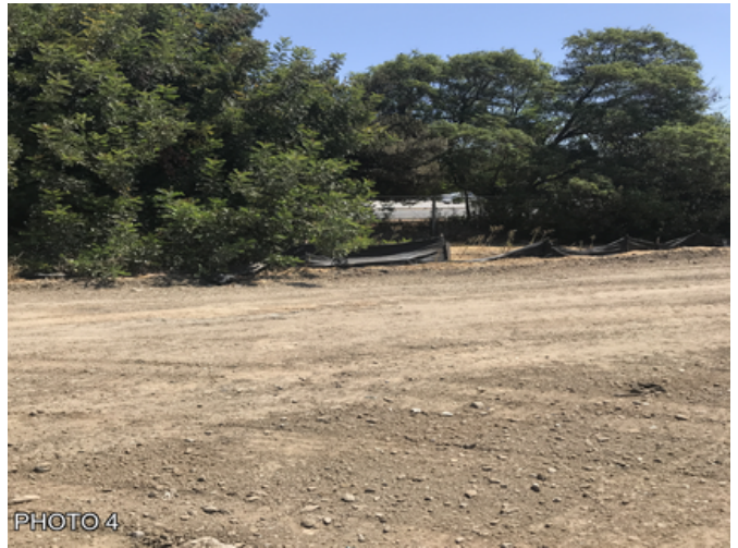
SILT FENCE ALONG WESTERN PROPERTY BOUNDARY
