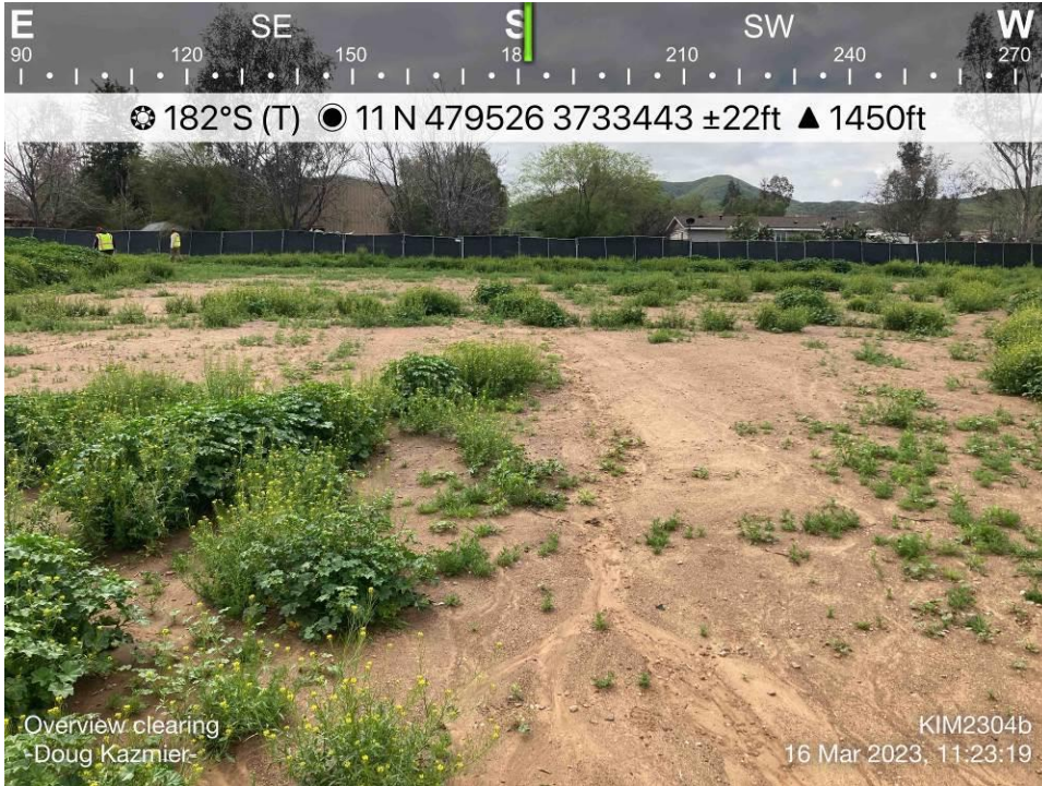
Photo 3: Project Site Overview from Near Southern Boundary
