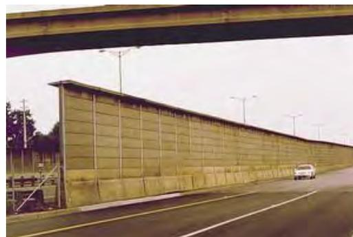
Figure 25. T-profile top barrier photo #1312
