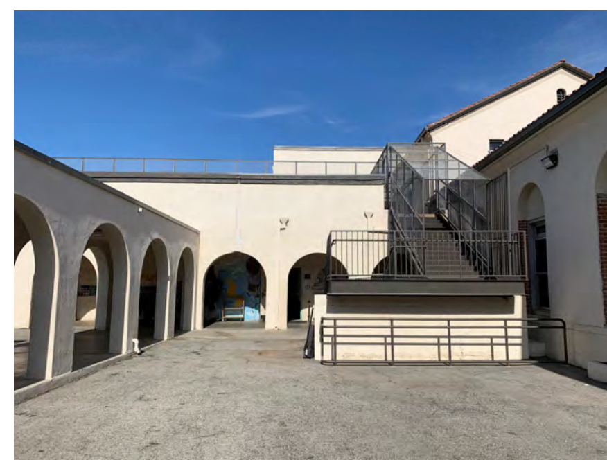
WEST EXIT STAIR
