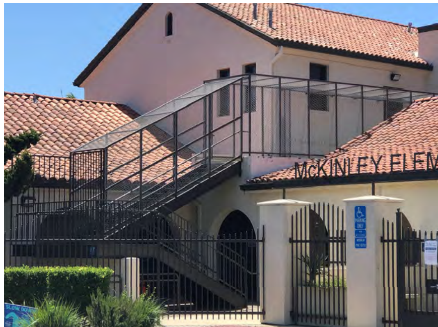
EAST EXIT STAIR
