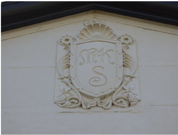
Detail, Building C. Northwest view.
