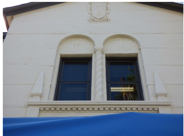
Building C. Northwest view.
