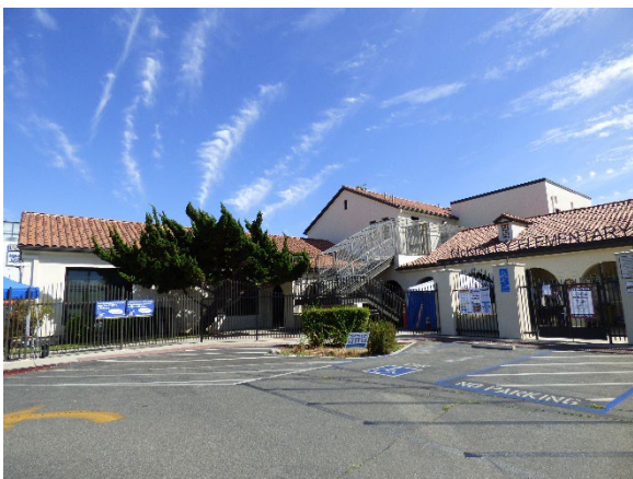
Building C. South view.
