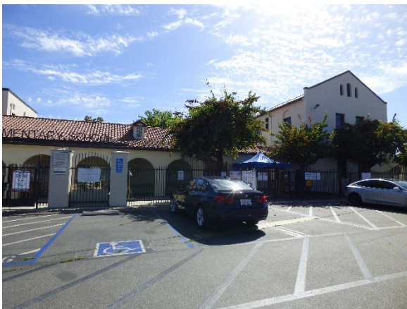
Building C. West view.
