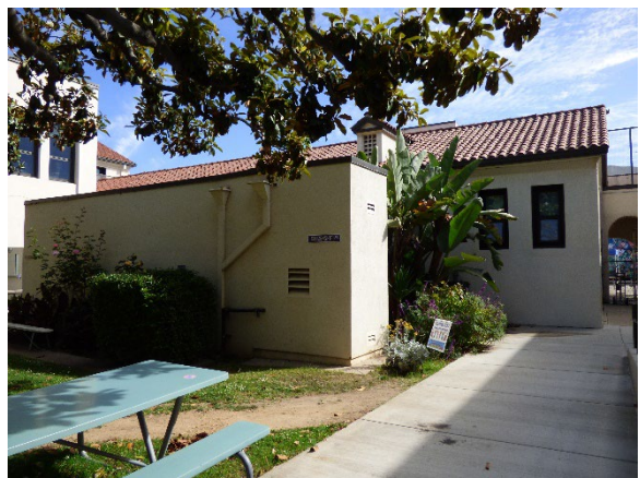
Building C. West view.
