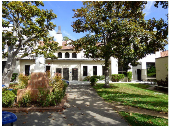
Building C. Southwest view.
