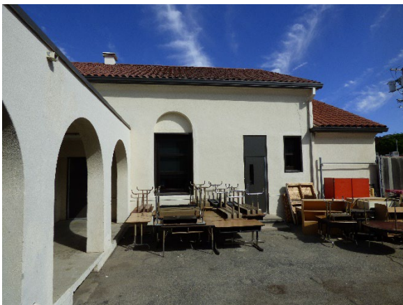
Building C. South view.
