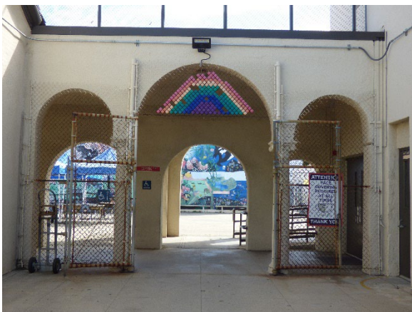
Arcade, Building C. East view.
