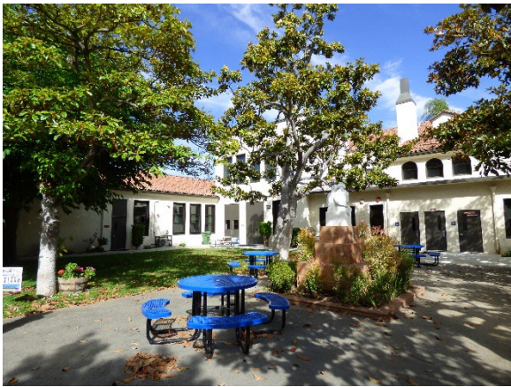
Building C. Southeast view.
