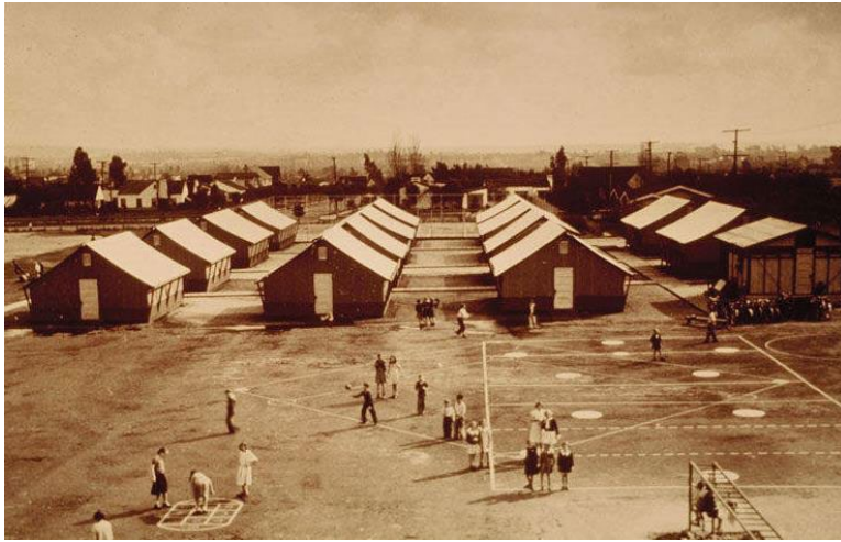
Tents on the Santa Monica High School campus after the 1933 Long Beach Earthquake. Source: Santa Monica Public Library.
