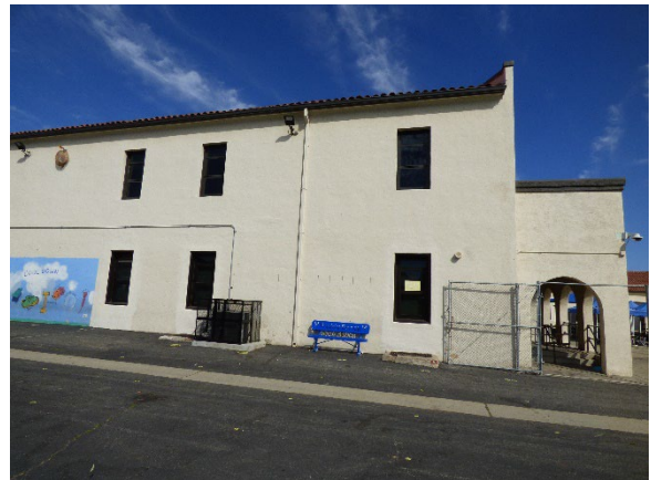
Building B. South view.
