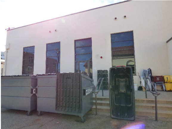
Building A. Northwest view.
