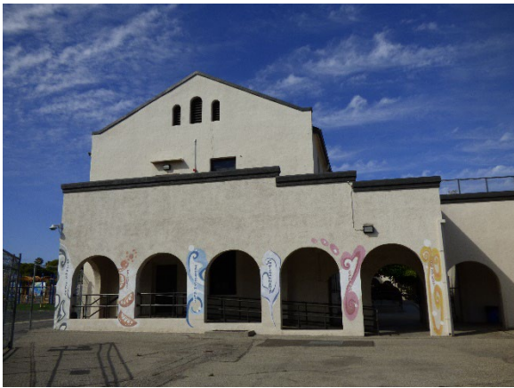
Building B. East view.
