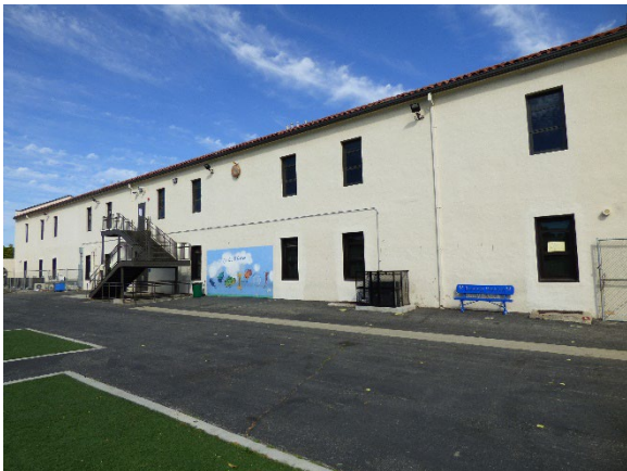
Building B. Southwest view.
