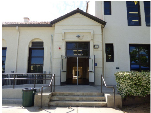
Building C. Northwest view.
