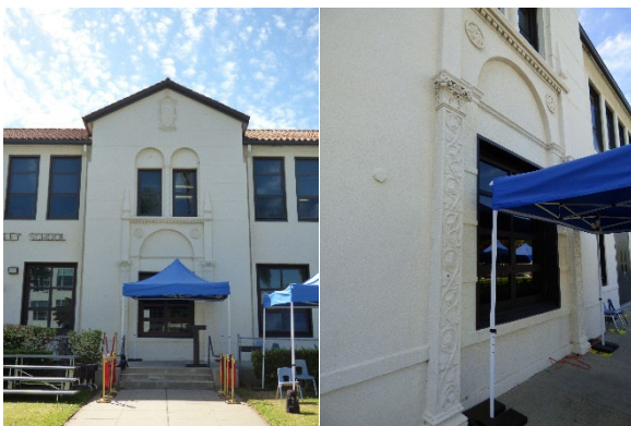
Entrance, Building C. Northwest and North view.
