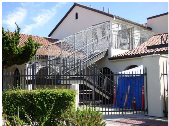
Detail, staircase. Building C. South view.
