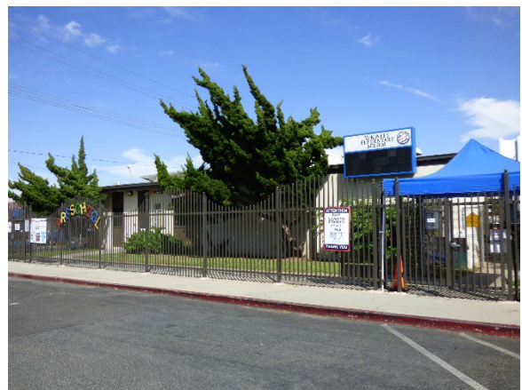
Building D Southeast view.
