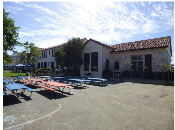
Building C. Northwest view.
