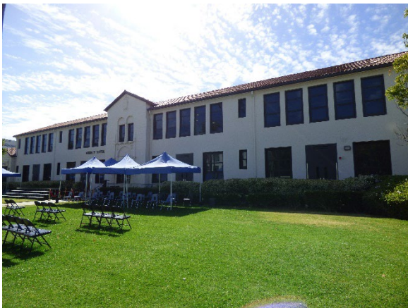
Building C. Northwest view.
