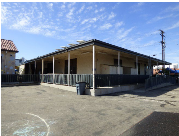
Building D. North view.
