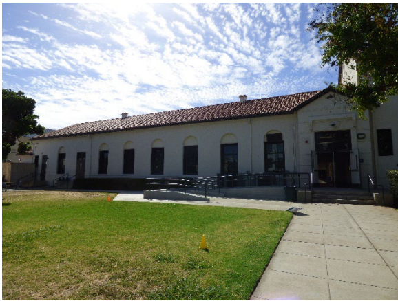
Building C. West view.
