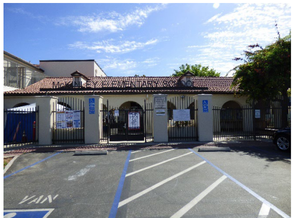
Building C. Southwest view.
