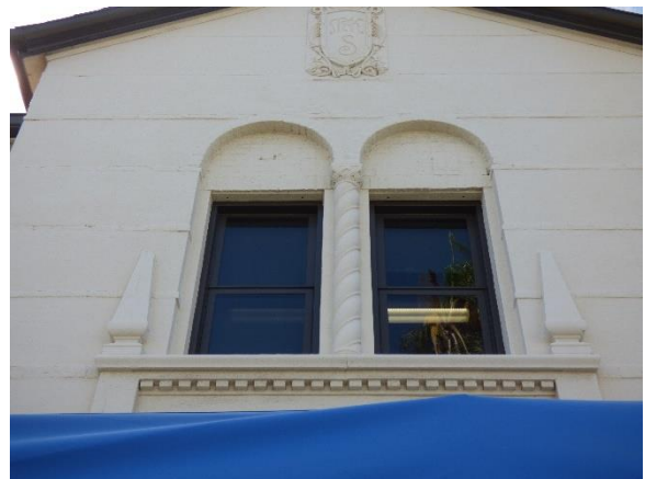
Building C. Northwest view.
