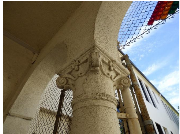
Detail, Building C. South view.
