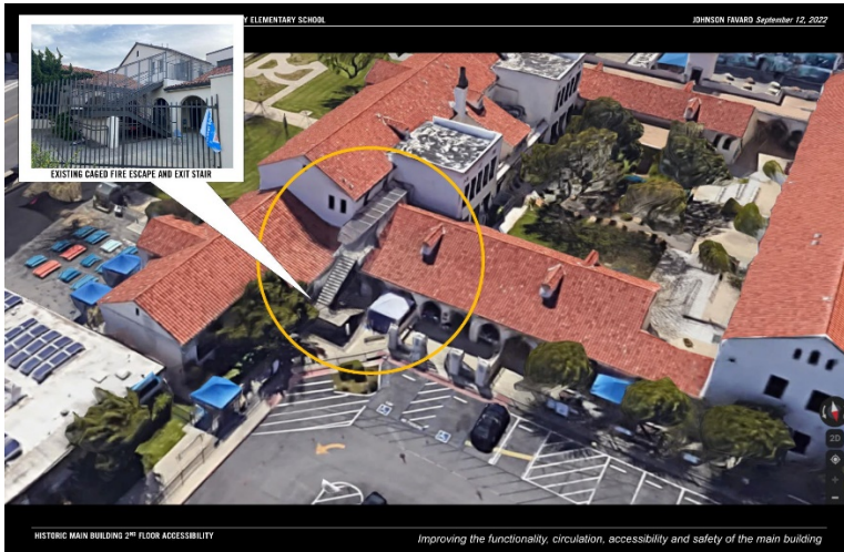
Main building south wing east fire escape/exit stair
