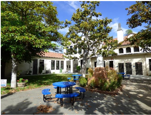
Building C. Southeast view.
