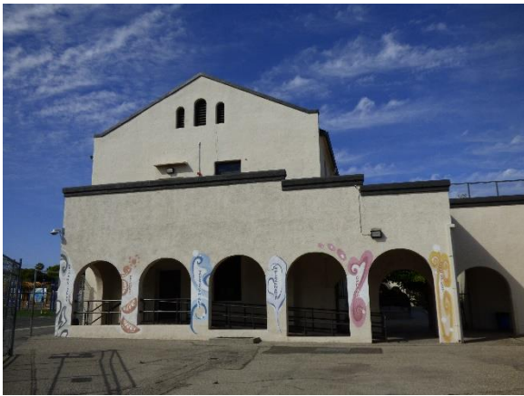
Building B. East view.
