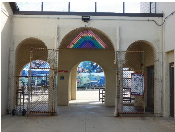
Arcade, Building C. East view.
