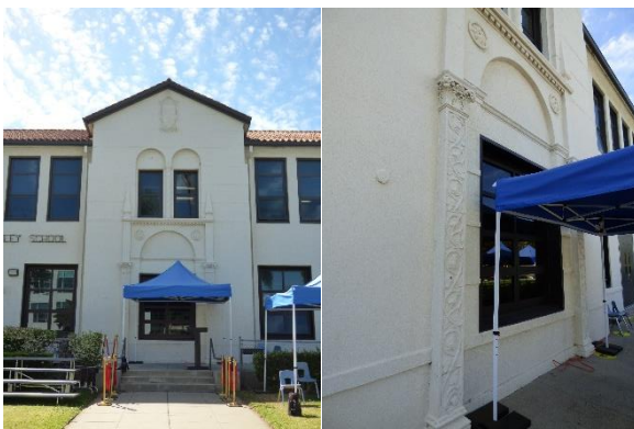
Entrance, Building C. Northwest and North view.
