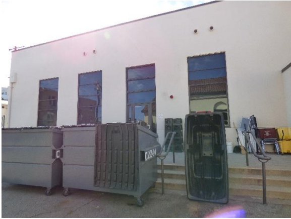
Building A. Northwest view.
