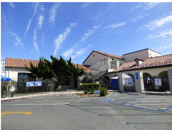
Building C. South view.
