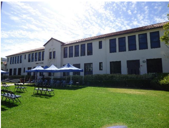
Building C. Northwest view.
