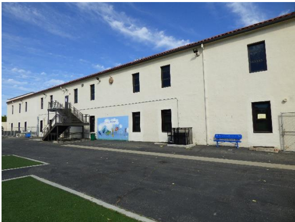
Building B. Southwest view.
