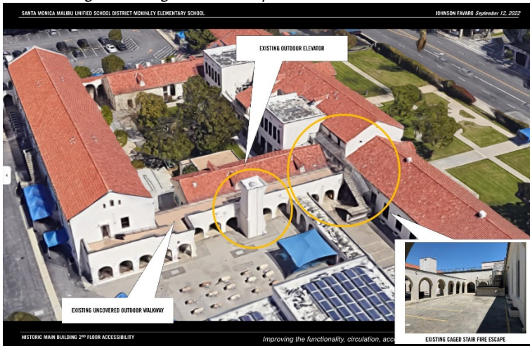
South wing west fire escape/exit stair, outdoor elevator, and rooftop walkway
