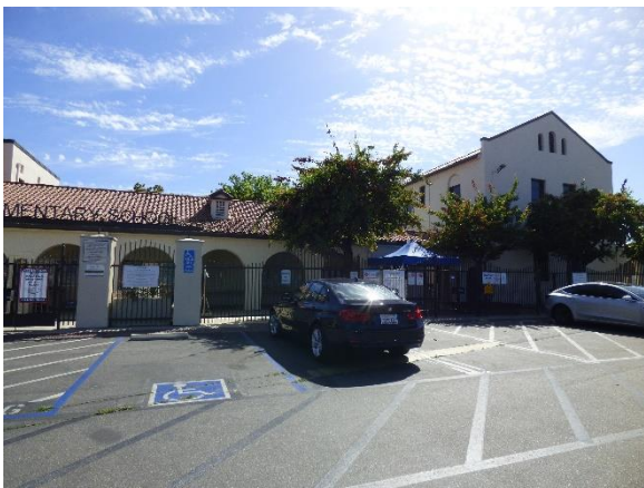
Building C. West view.
