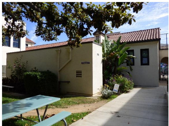
Building C. West view.
