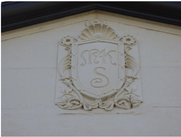
Detail, Building C. Northwest view.
