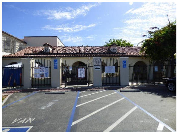
Building C. Southwest view.
