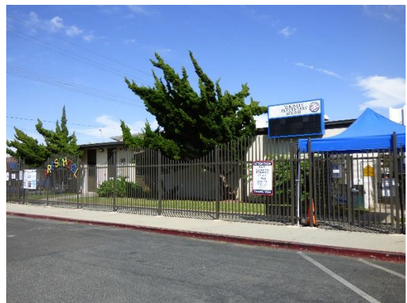
Building D Southeast view.
