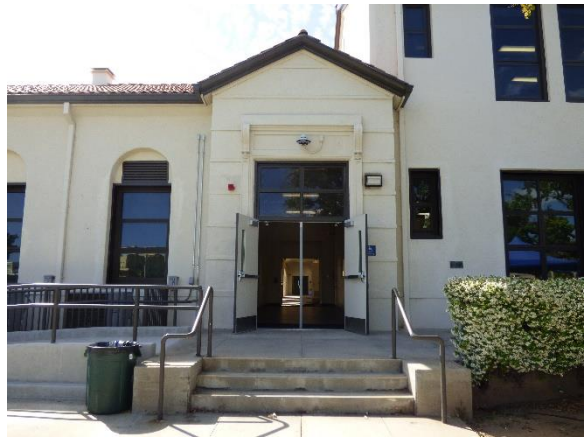
Building C. Northwest view.
