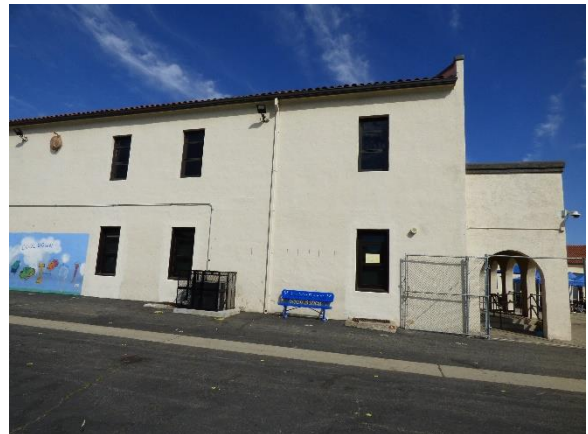
Building B. South view.
