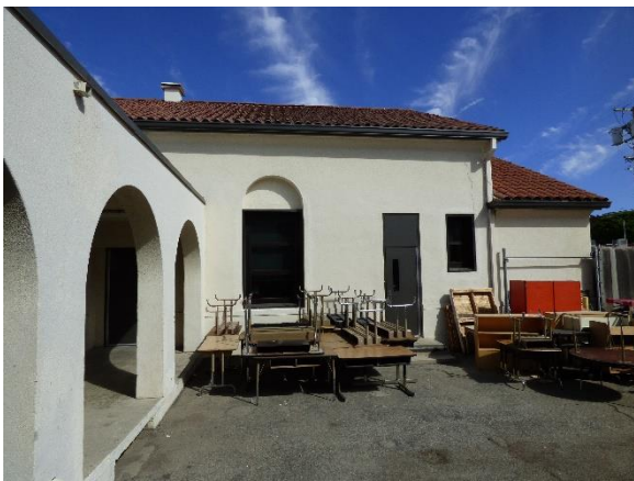
Building C. South view.
