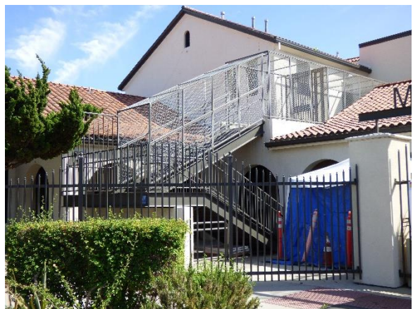
Detail, staircase. Building C. South view.
