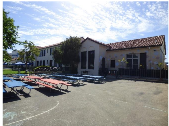
Building C. Northwest view.
