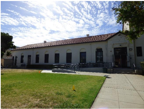
Building C. West view.
