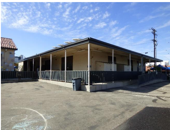
Building D. North view.
