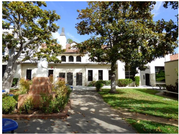
Building C. Southwest view.
