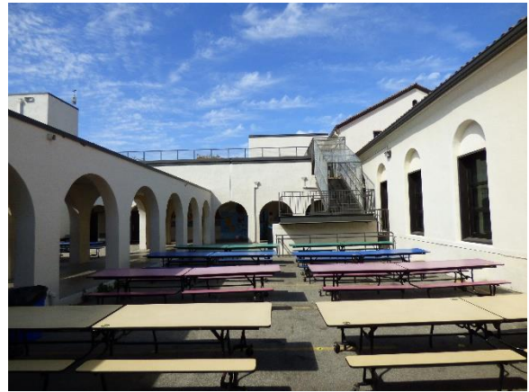
West Courtyard. Northeast view.
