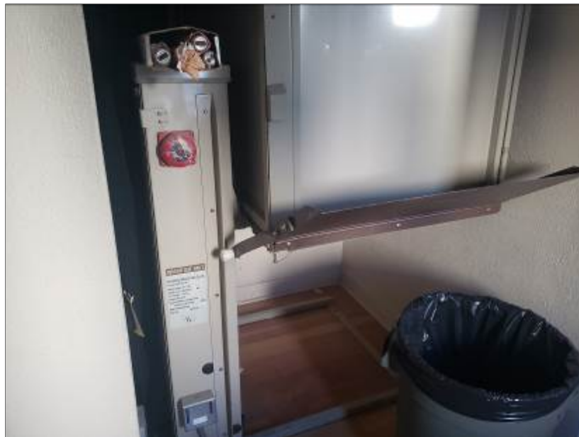
Photo 12: Typical Classroom Building Interior
