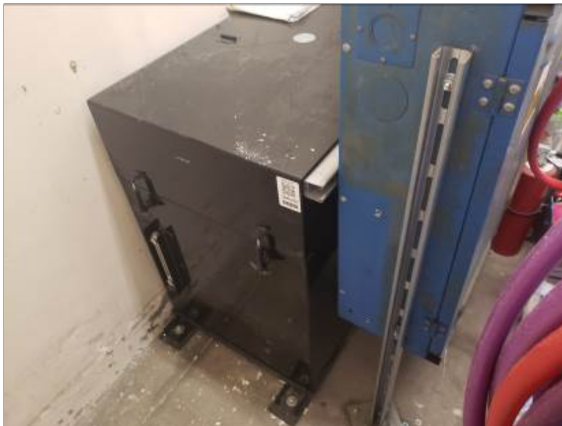
Photo 16: Passenger Elevator Equipment
