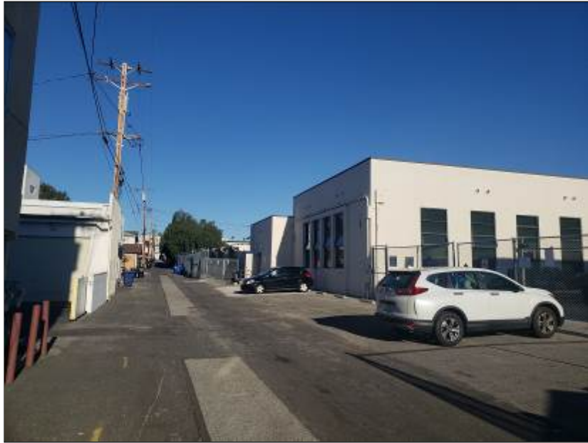
Photo 3: Southwestern Boundary of Site – 23 rd Court
