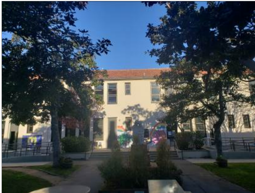
Photo 20: Classroom Building Exterior
