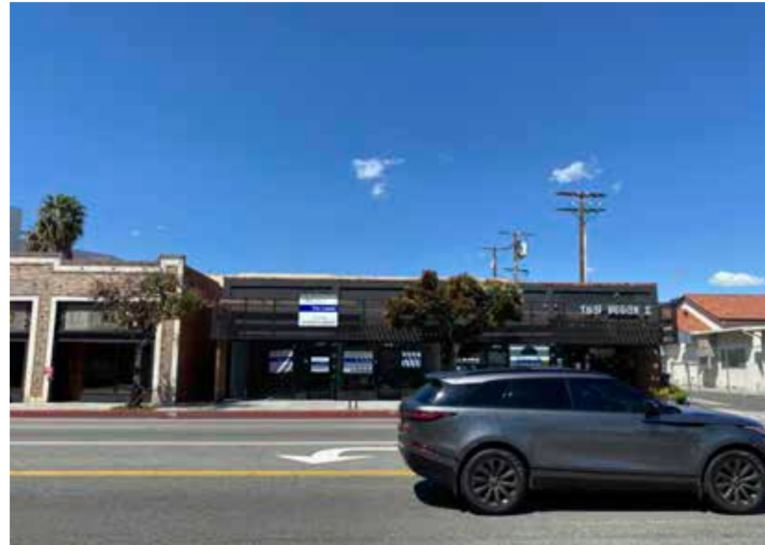
GLASS STOREFRONT RETAIL Commercial one-story buildings front the north side of Santa Monica Blvd. on the west side of McKinley Elementary School and picking up again past Chelsea Avenue to the east.
