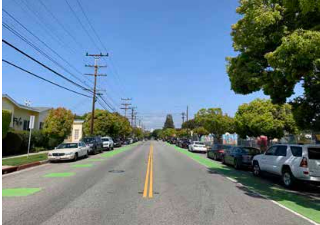
ARIZONA AVENUE LOOKING EAST Forming the northern boundary of McKinley Elementary School, this two lane street has dedicated bike lanes in either direction with curbside parking on both sides.
