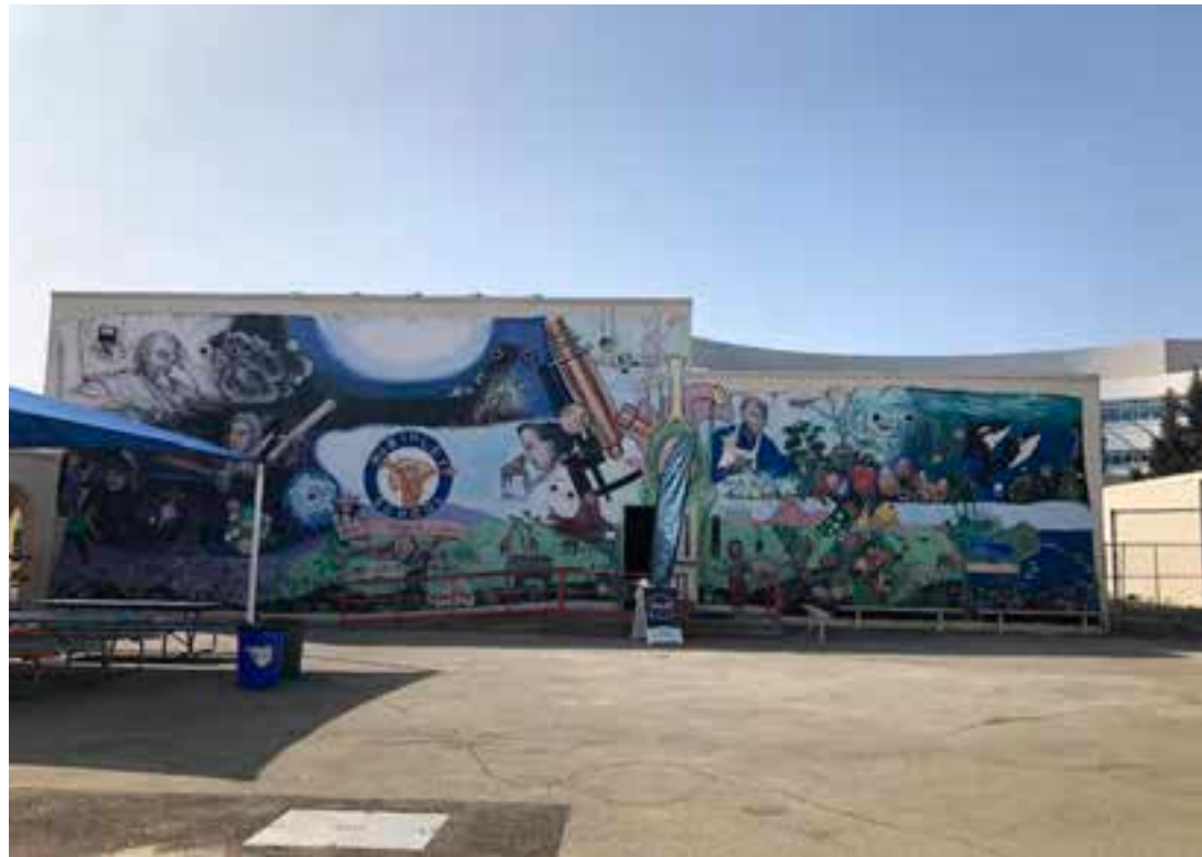
MULTIPURPOSE CAFETERIA & KITCHEN The building is located off 23rd Court and faces an empty paved interior court and houses an office for the CREST program.
