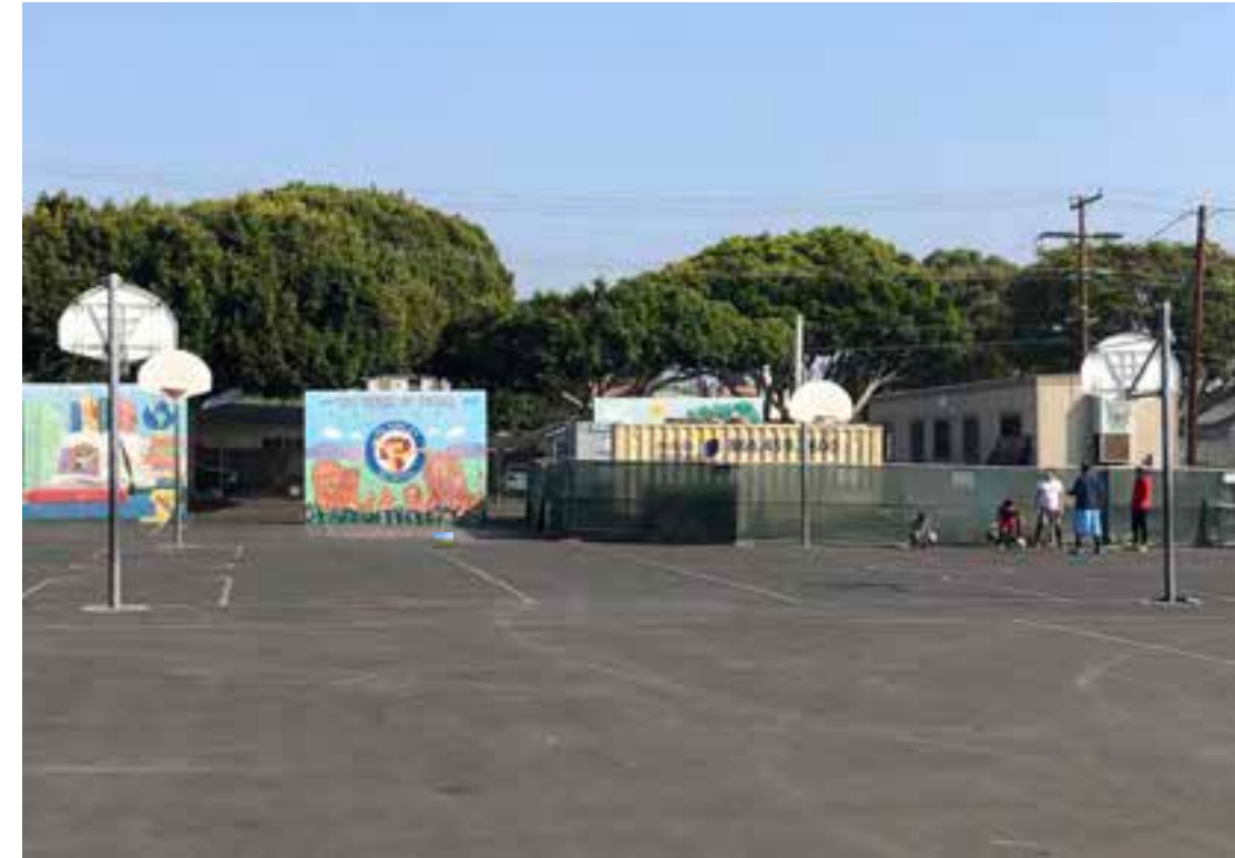
HANDBALL AND BASKETBALL COURTS A variety of courts occupy the northeast zone of the playground. Due to the large area the playground covers, the handball courts locate remotely, creating hard to surveil areas.
