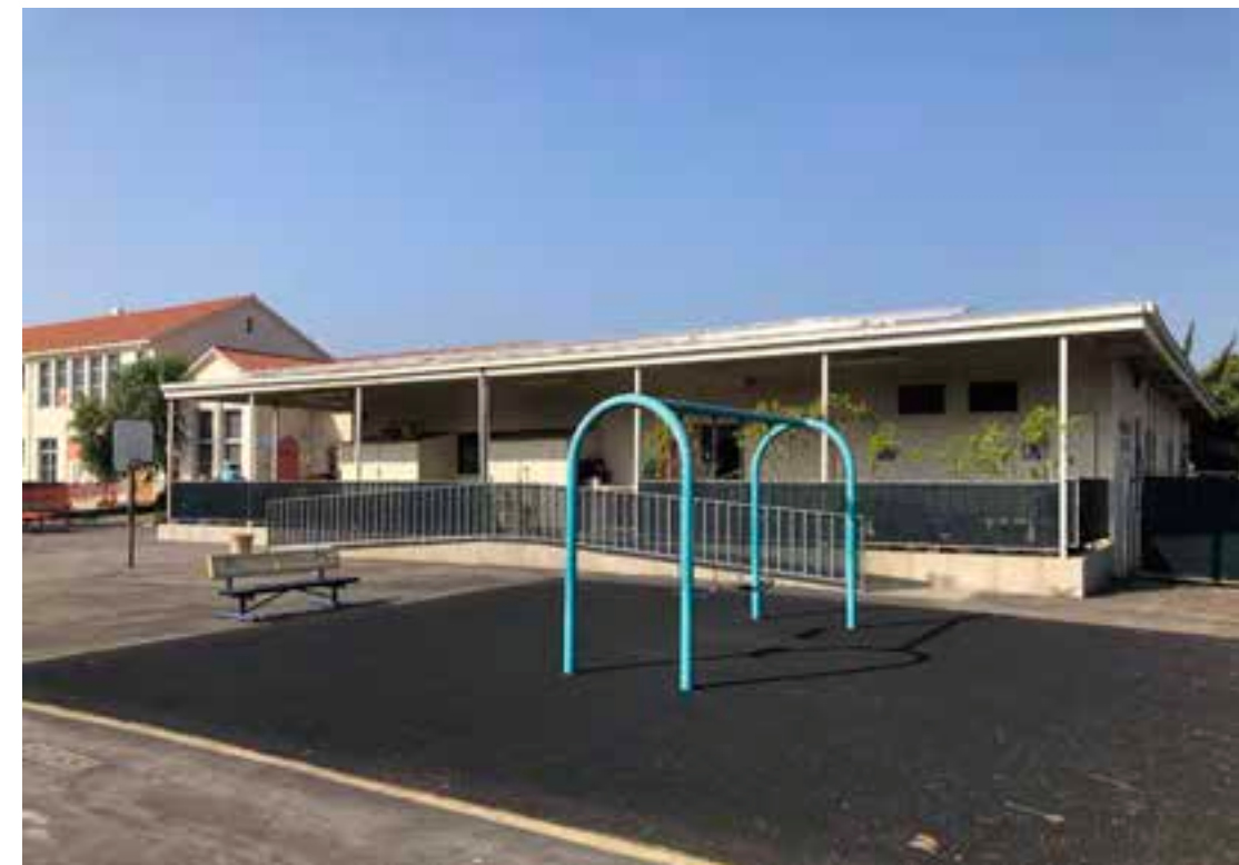
EARLY CHILDHOOD MODULAR This building is situated outside the central core of campus, occupying the southeast corner of campus at the corner of Santa Monica Boulevard and Chelsea Avenue.
