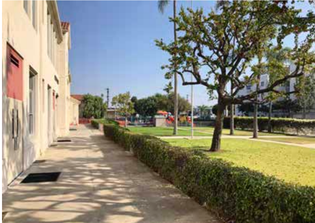
SOUTH PATIO AT BUILDING C Largely unused, the south patio connects the kindergarten classrooms with preschool building D and the relocatables at the southwestern corner of campus.
