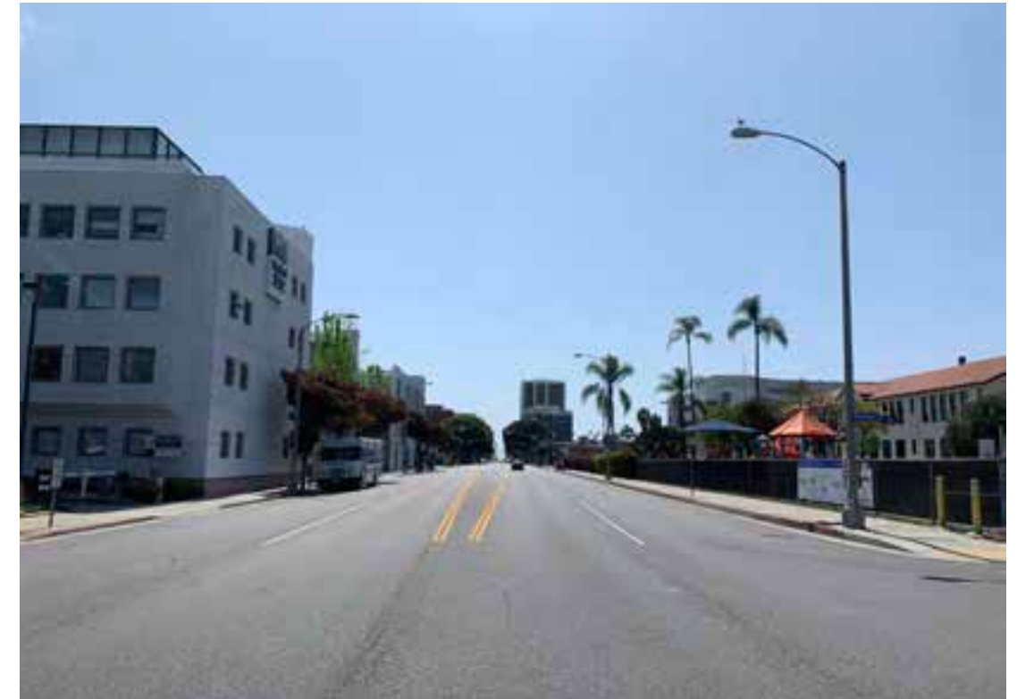
SANTA MONICA BOULEVARD LOOKING WEST The school fronts on Santa Monica Blvd, a major west-east thoroughfare connecting the Pacific Ocean to Sunset Junction in the Los Angeles neighborhood of Silverlake.
