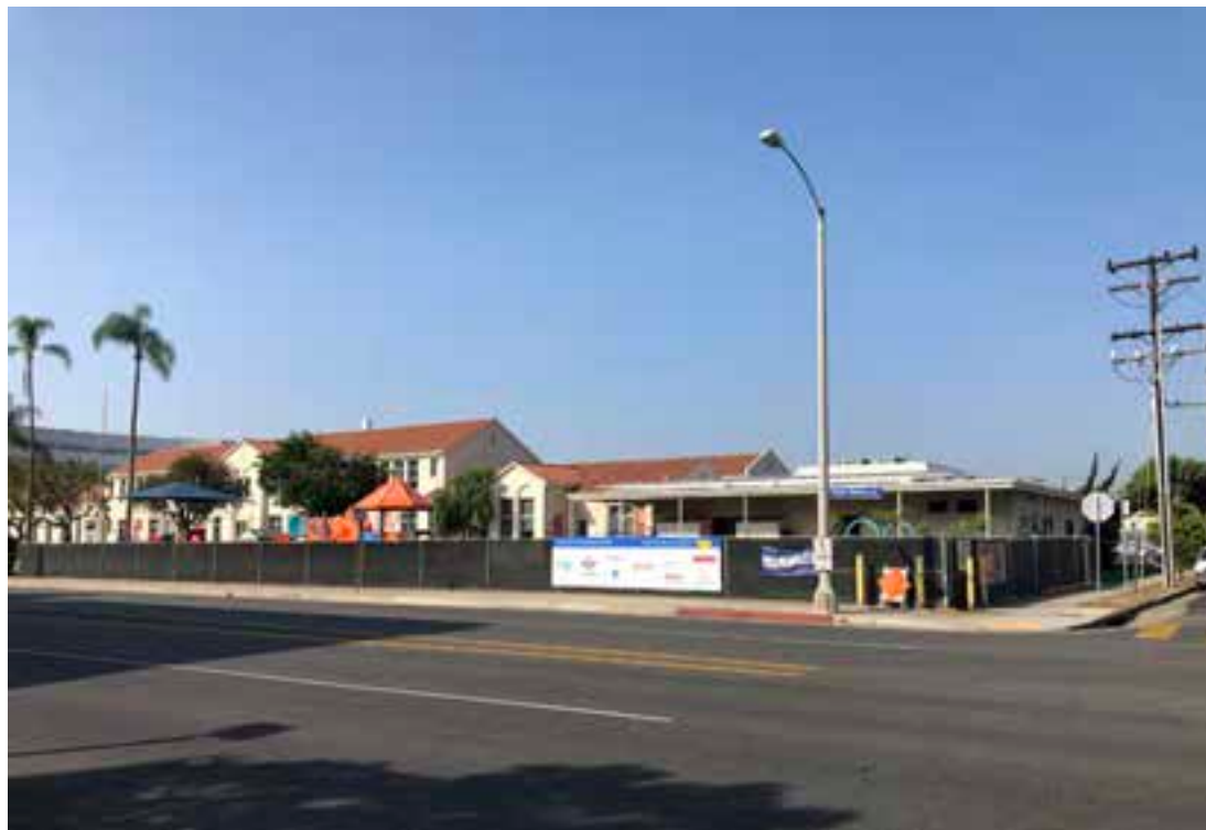
SOUTH PERIMETER Chain link fencing with fabric screening separates the early childhood play yard from Santa Monica Boulevard and Chelsea Avenue.
