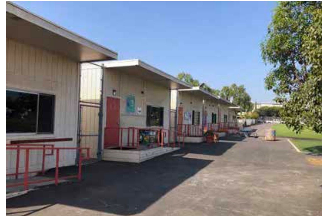
SECOND GRADE, ART & COMPUTER ROOM RELOCATABLE CLASSROOMS These buildings occupy the middle of the western perimeter of campus.
