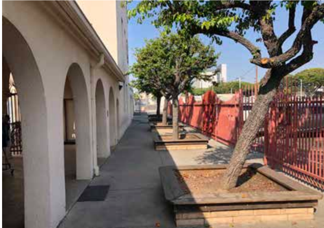
EAST PERIMETER A variable height painted vertical bar enclosure separates the interior of campus from the main parking lot off Chelsea Avenue.
