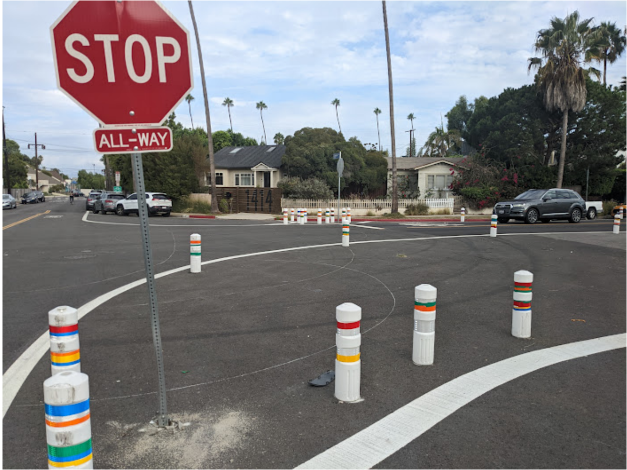
Exhibit #2: Example of safe streets design using K71 flex-post bollards in the City of Los Angeles.
