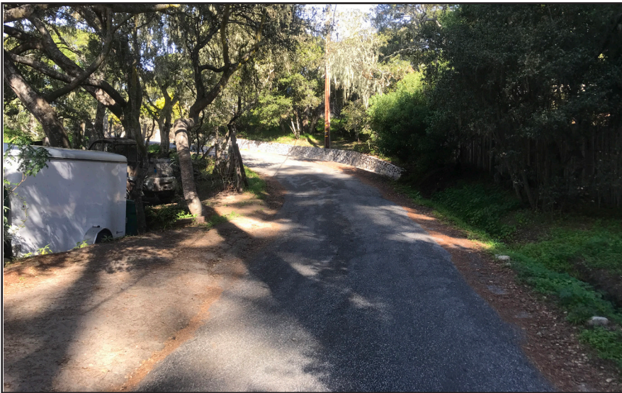
Photo #3: Pipeline alignment from Corona Way.
