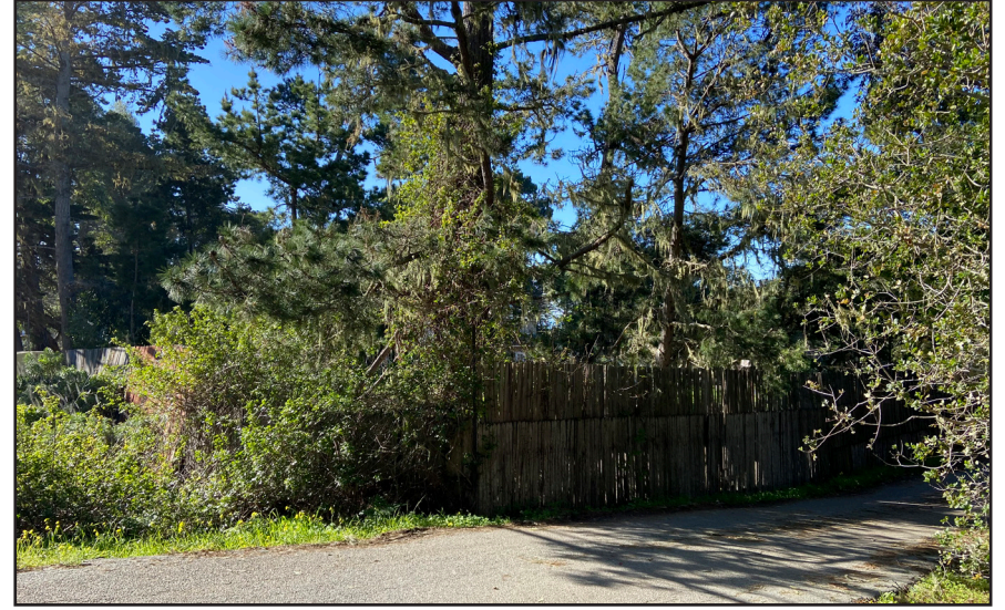
Photo #10: Location of Pump Station on the west side of State Route 1.
