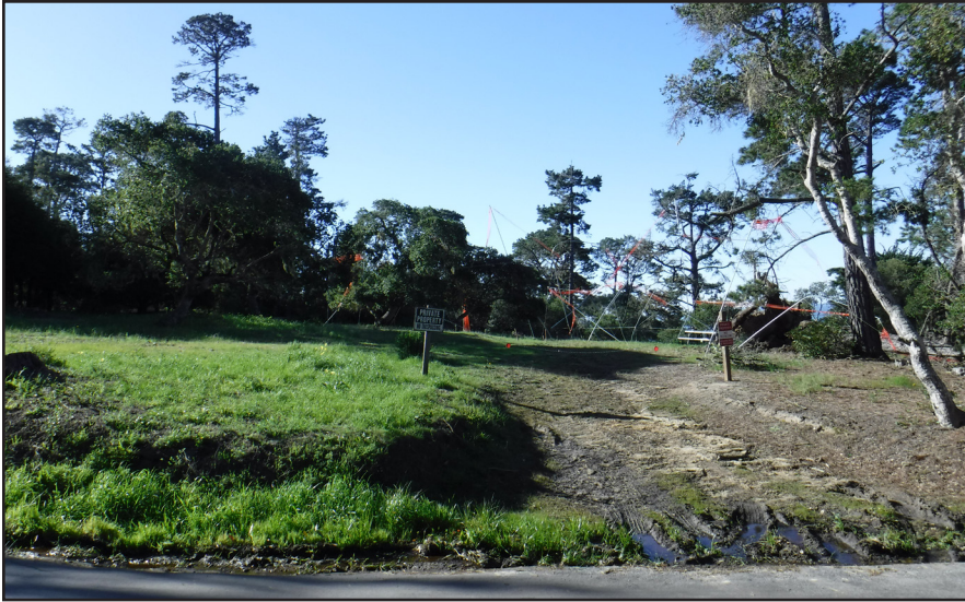
Photo #13: Staging Area from Corona Road looking south.
