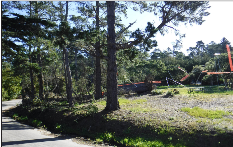
Photo #15: Staging Area from Corona Road looking east.
