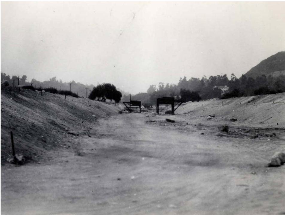
Construction of Arroyo Seco Channel, 1934.
