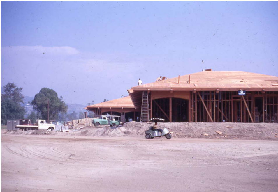
Construction of new clubhouse looking north, 1967.
