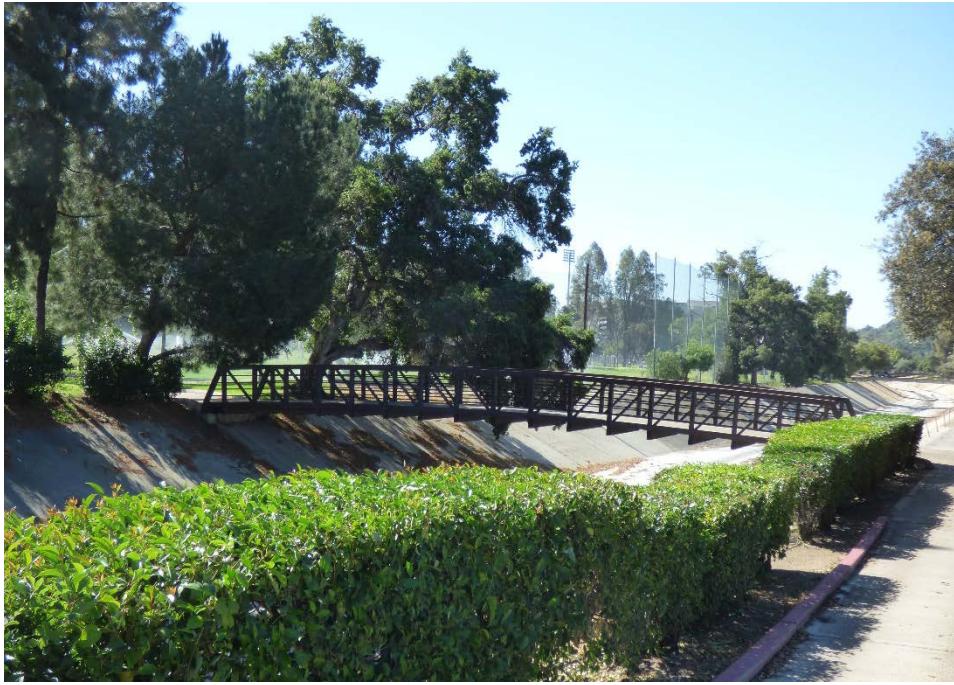
View of Arroyo Seco Channel and wood cross bridge with driving range in background looking northeast. Historic Resources Group, 2021.
