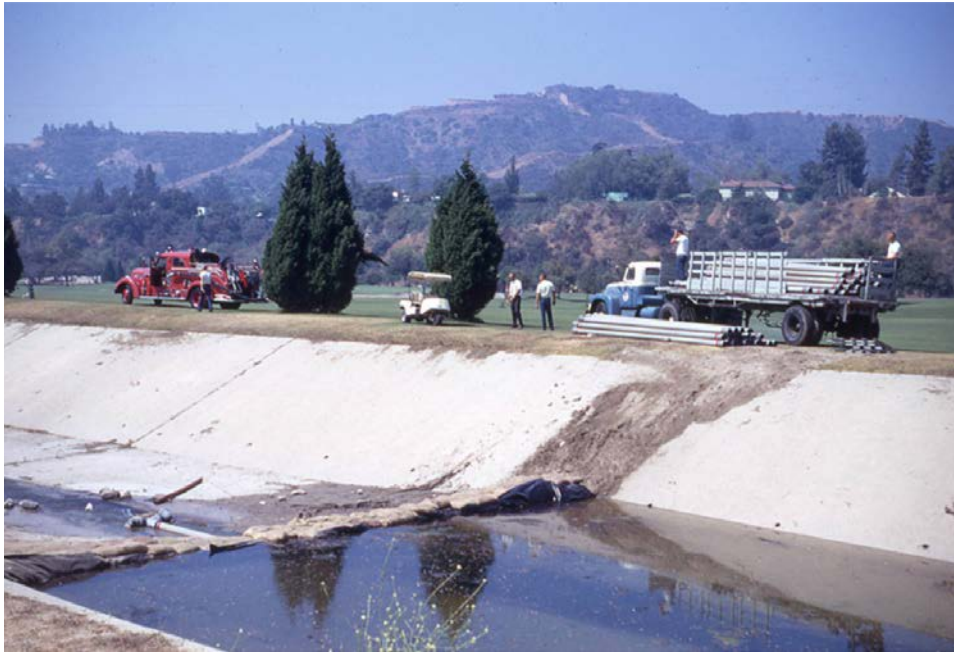
Renovation of Arroyo Seco Channel block, 1967.
