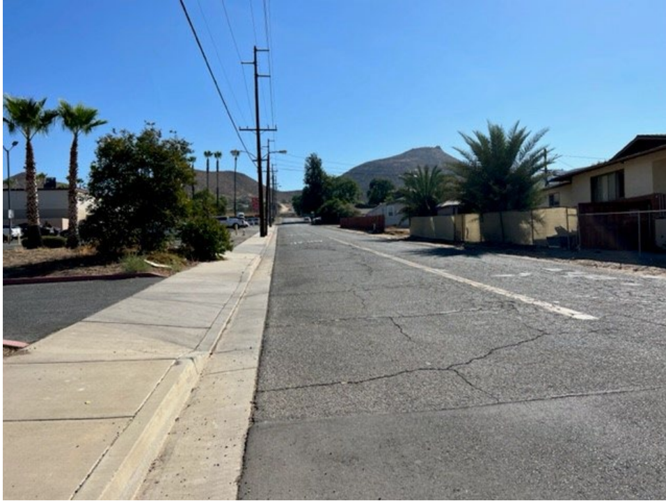
Plate 1. Malaga Road (northern project boundary), looking east; photo #2.
