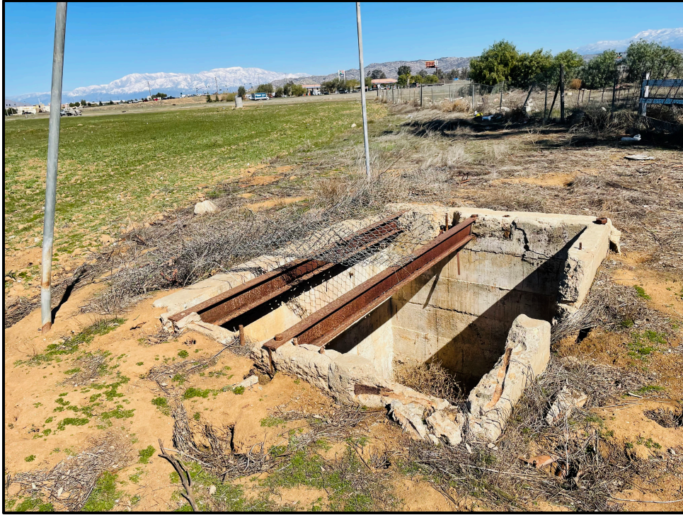
Plate 3.2–3: A concrete well (ISO-1) noted along the southern boundary of the property that is associated with the previous rural residence (now gone) located immediately south of the survey area.
