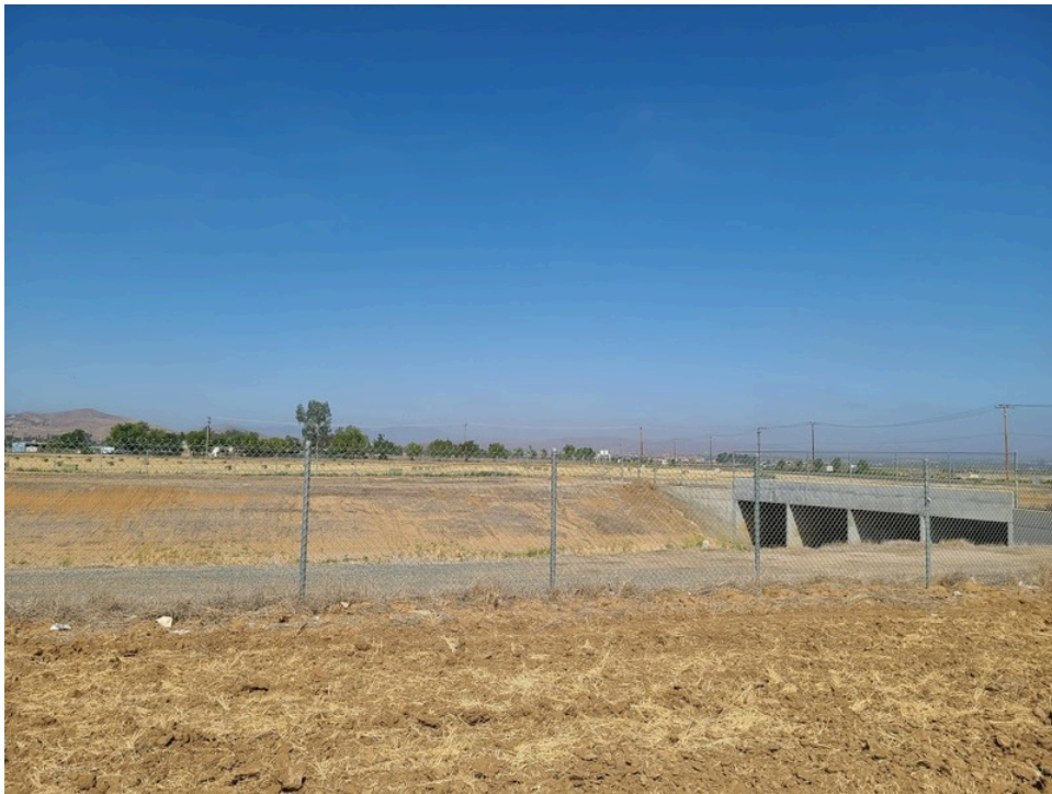
16. Dry River Bed Adjoining to the West
