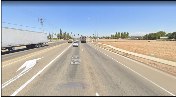
Photo 1: View of intersection looking north. Source: Google Earth, 12/20/2022
