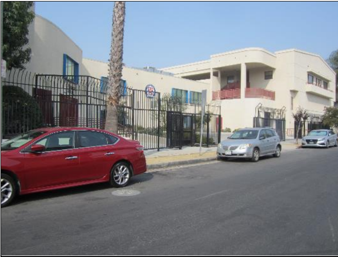
7. Southern side of the subject building.
