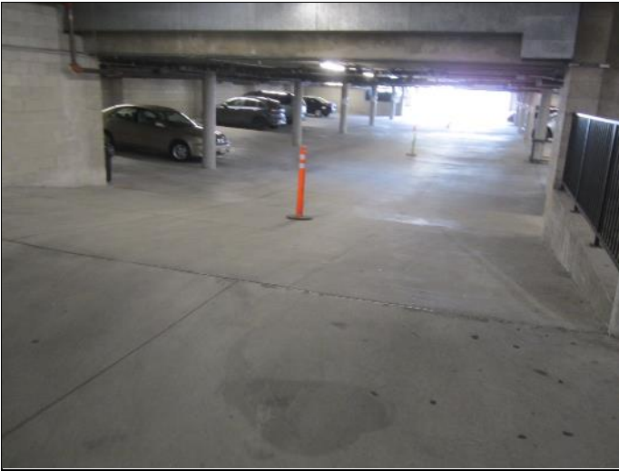
13. Parking garage at the subject property.
