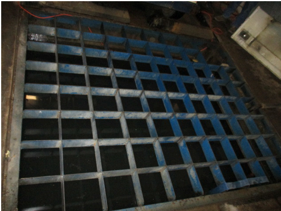
26. Concrete-lined pit with melt water in the Zamboni storage room
