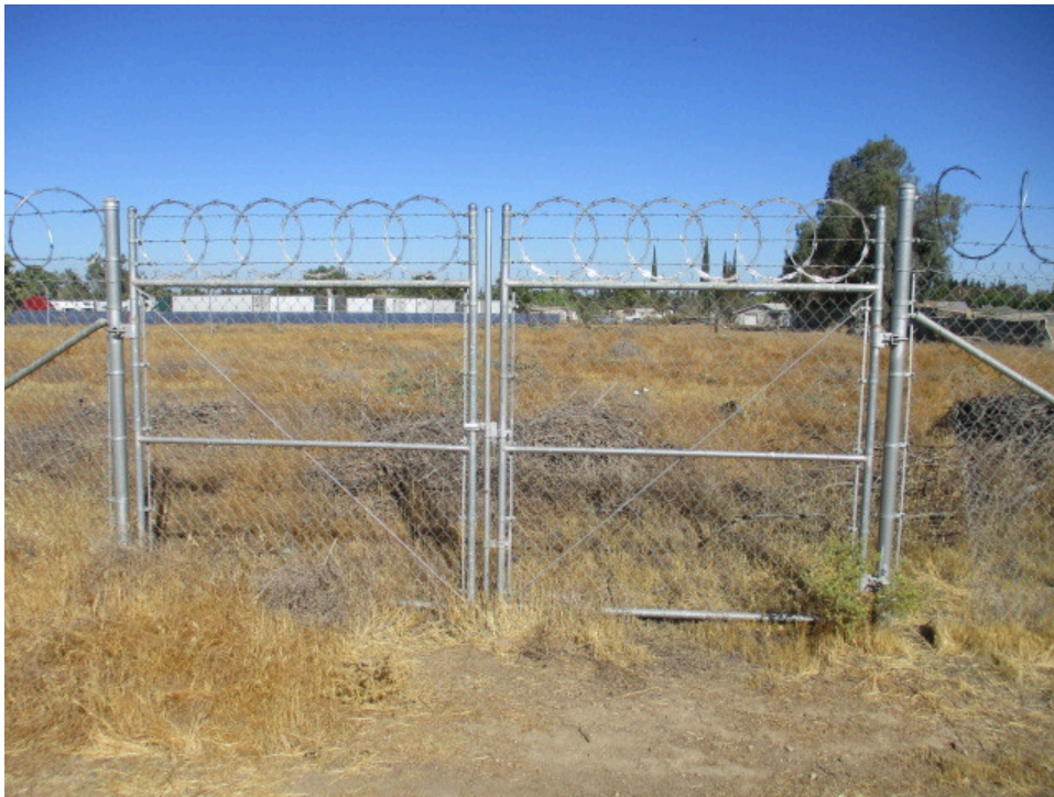
18. Gate and fence at the northwestern end of the subject property
