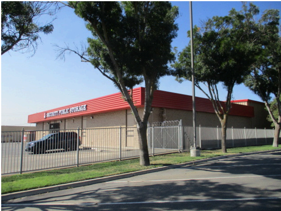
40. Security Pacific Storage adjacent to the south and east
