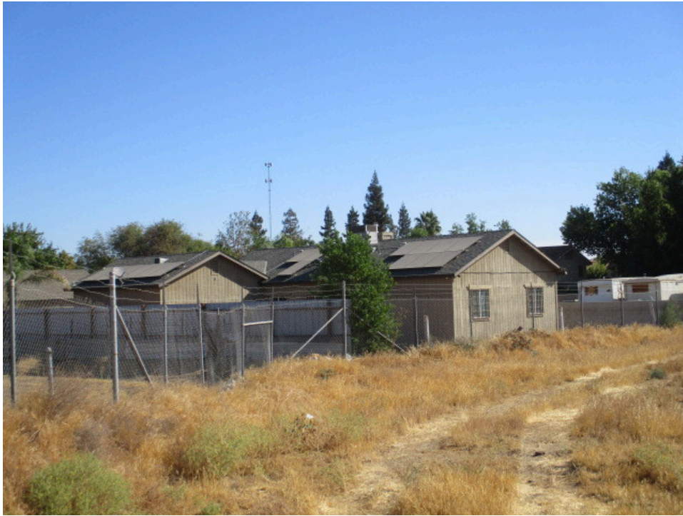
33. Residences adjacent to the north
