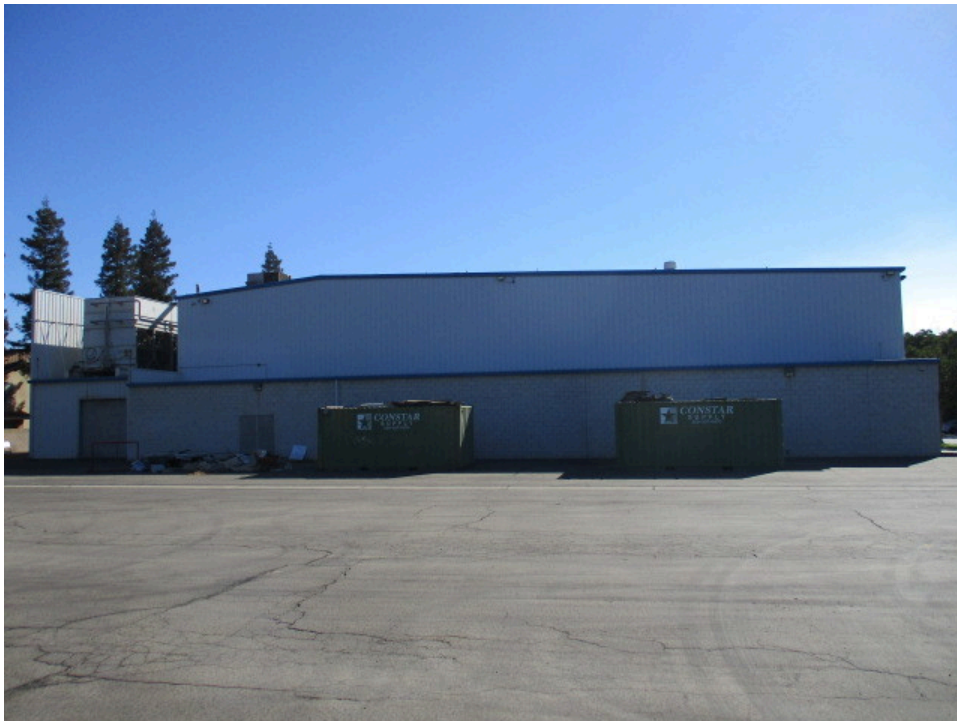
4. Western side of the Gateway Ice Center
