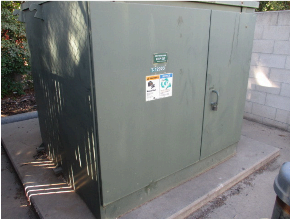
5. Pad-mounted transformer
