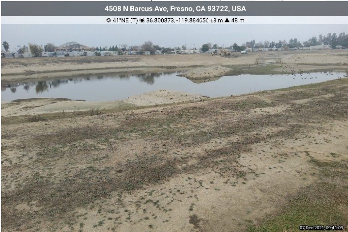
Photo 15 – City Retention Pond (View Northeast)
