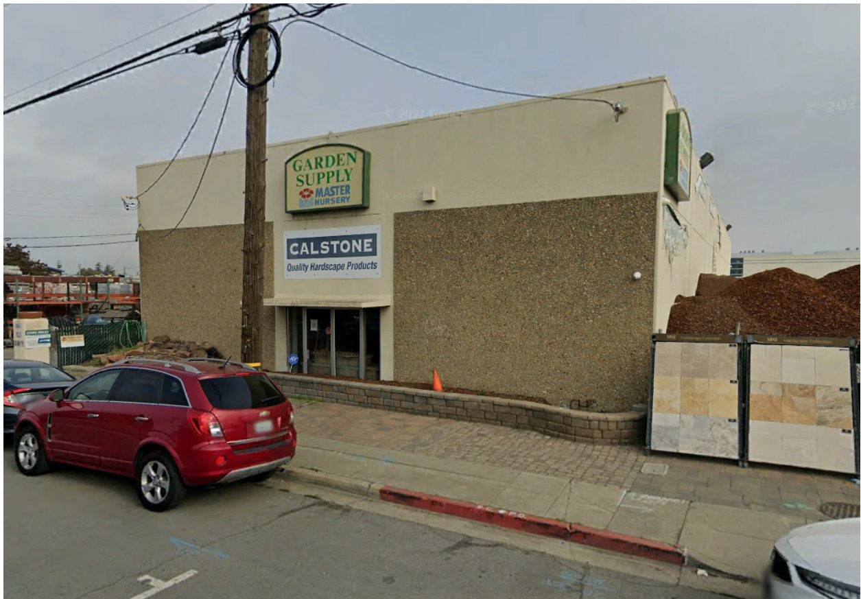
Fig.8 – 803 Old County Rd. – Front (west), from Old County Rd.
