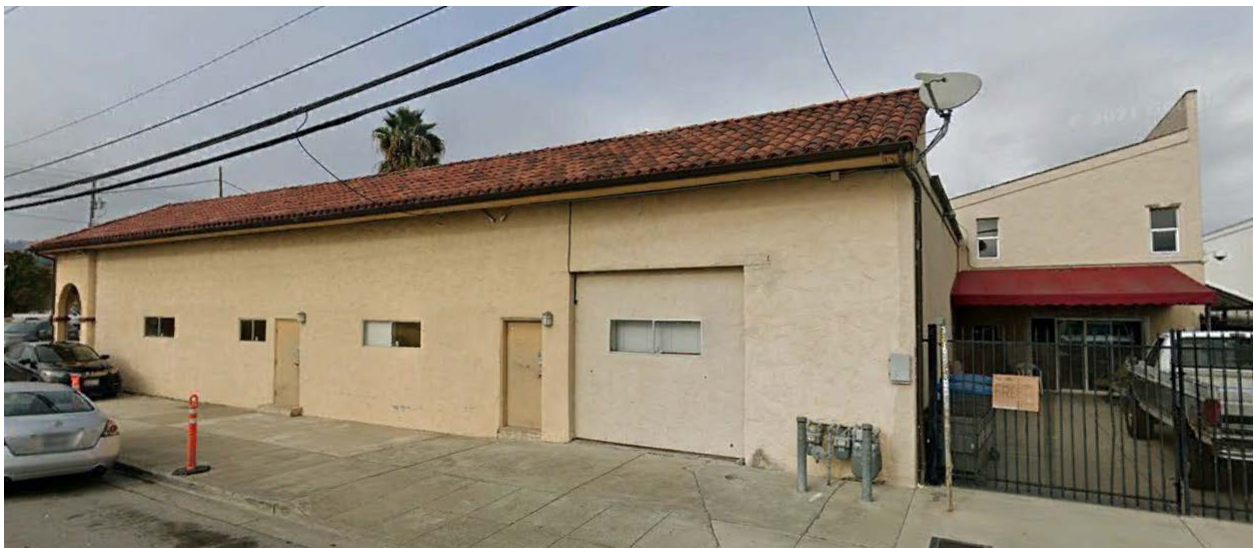
Fig.16 – 851 Old County Rd. – South side and part rear, from Commercial St.
