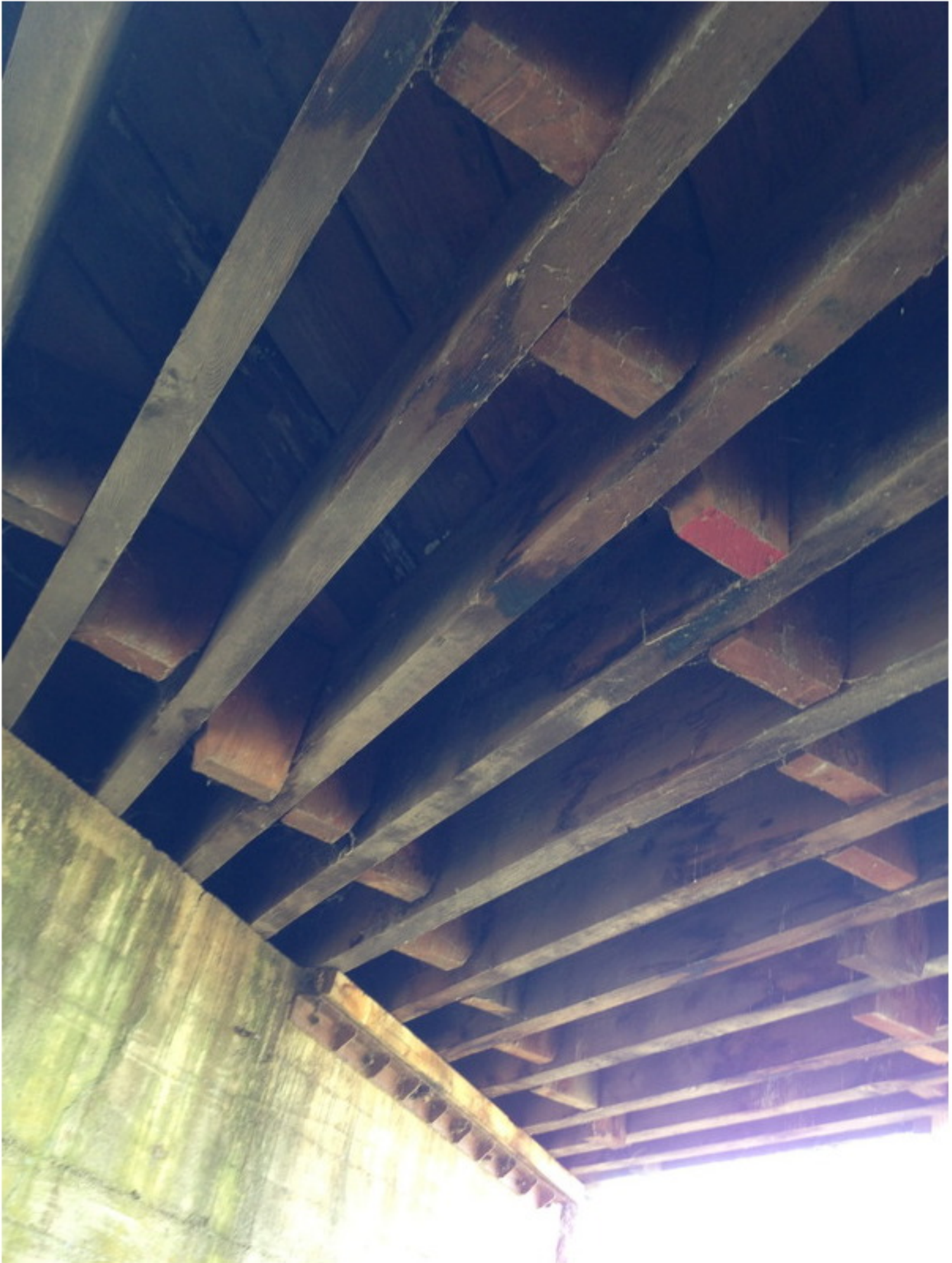
Photo No. 3 Underside Span 1.
