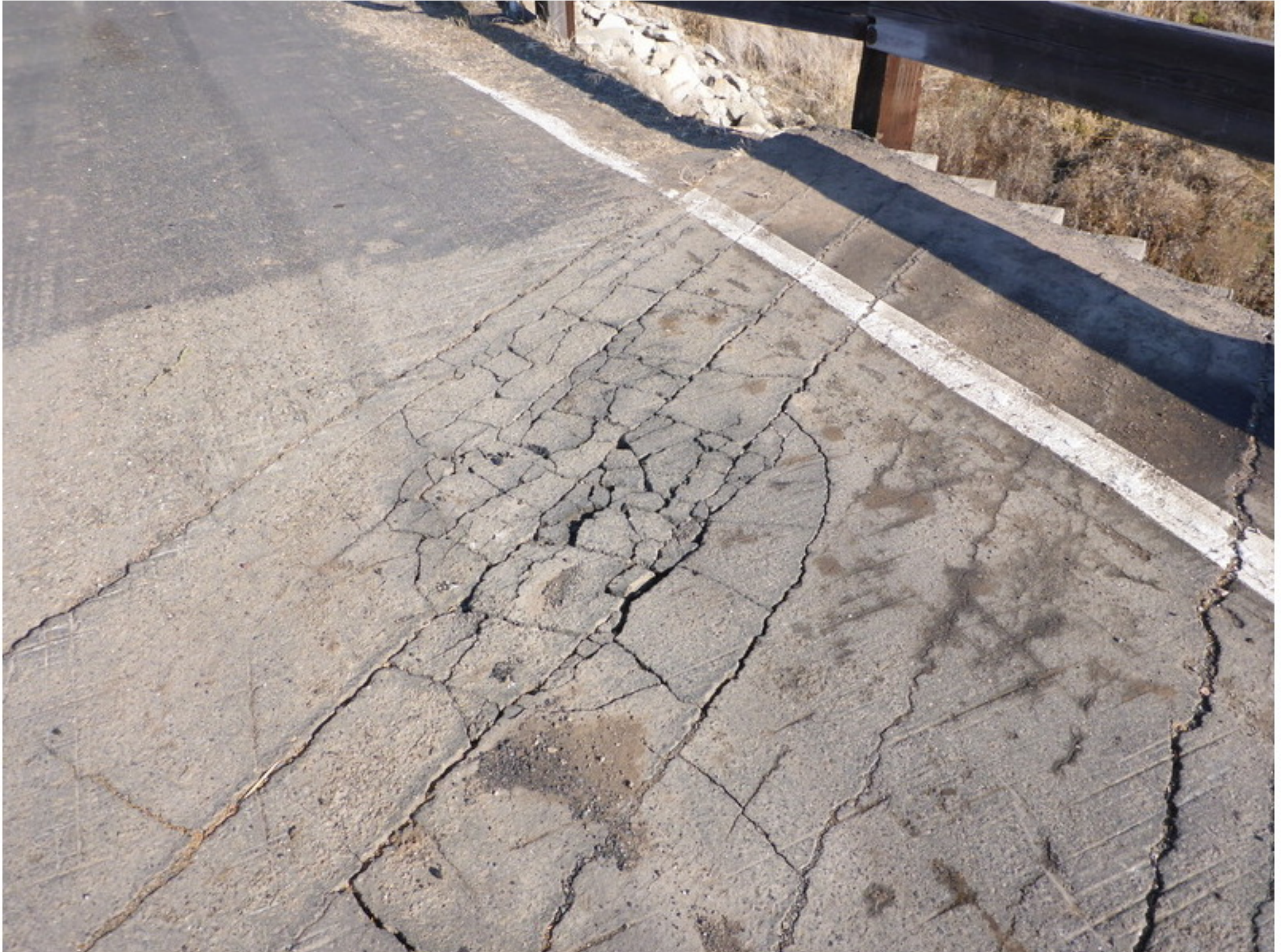
Photo No. 4 Bridge deck at Abutment 4, left side
