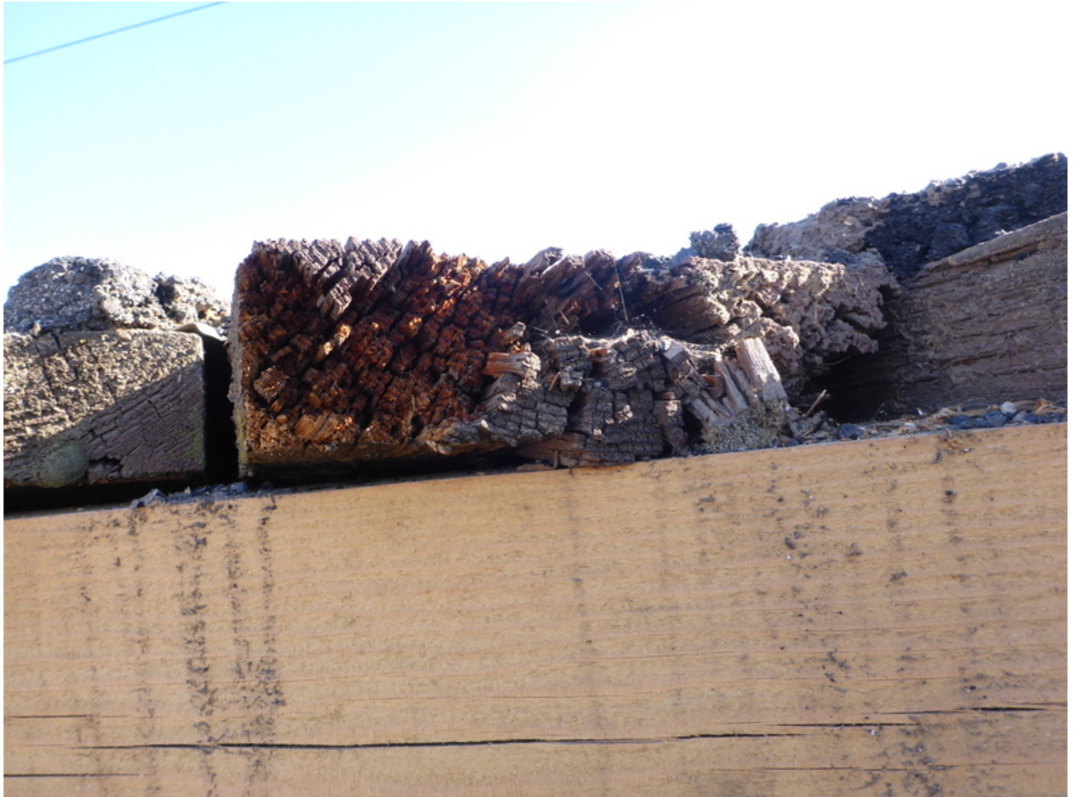
Photo No. 6 Typical condition of the deck board edges
