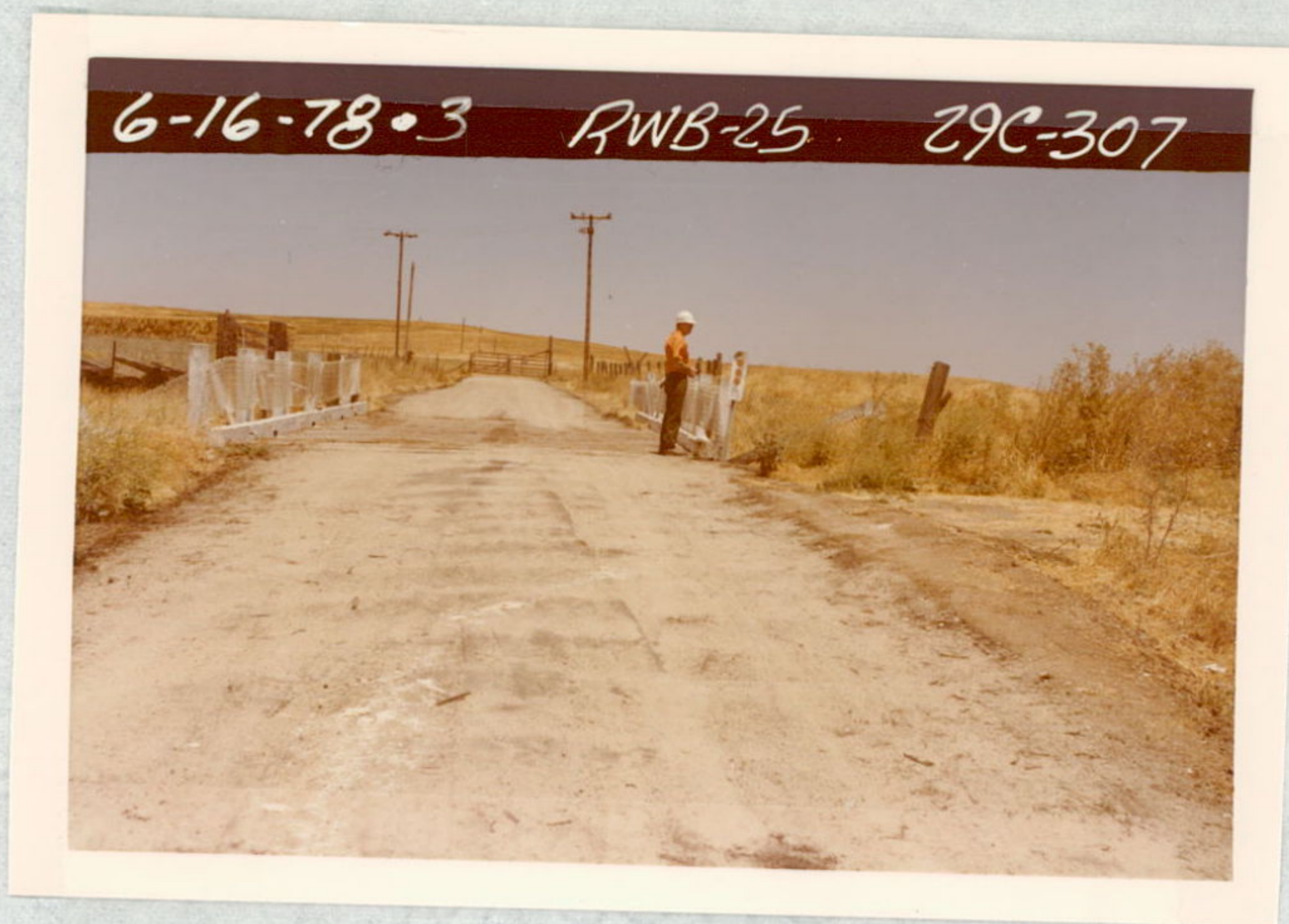
ROADWAY LOOKING NORTH
