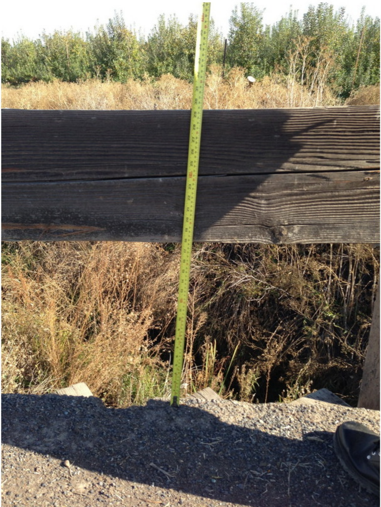
Photo No. 5 Bridge rail.
