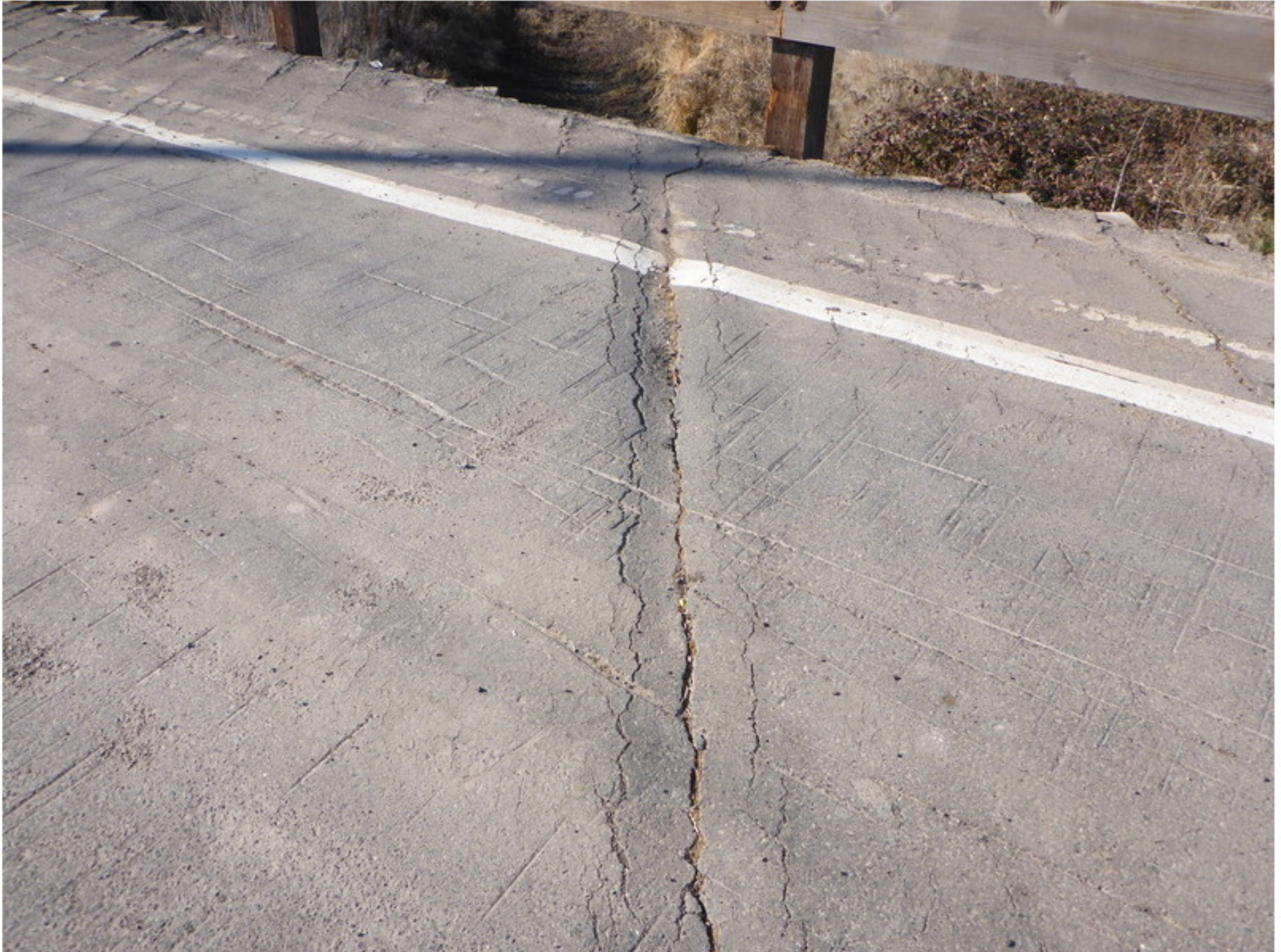
Photo No. 3 Rotten deck board in the middle of the bridge
