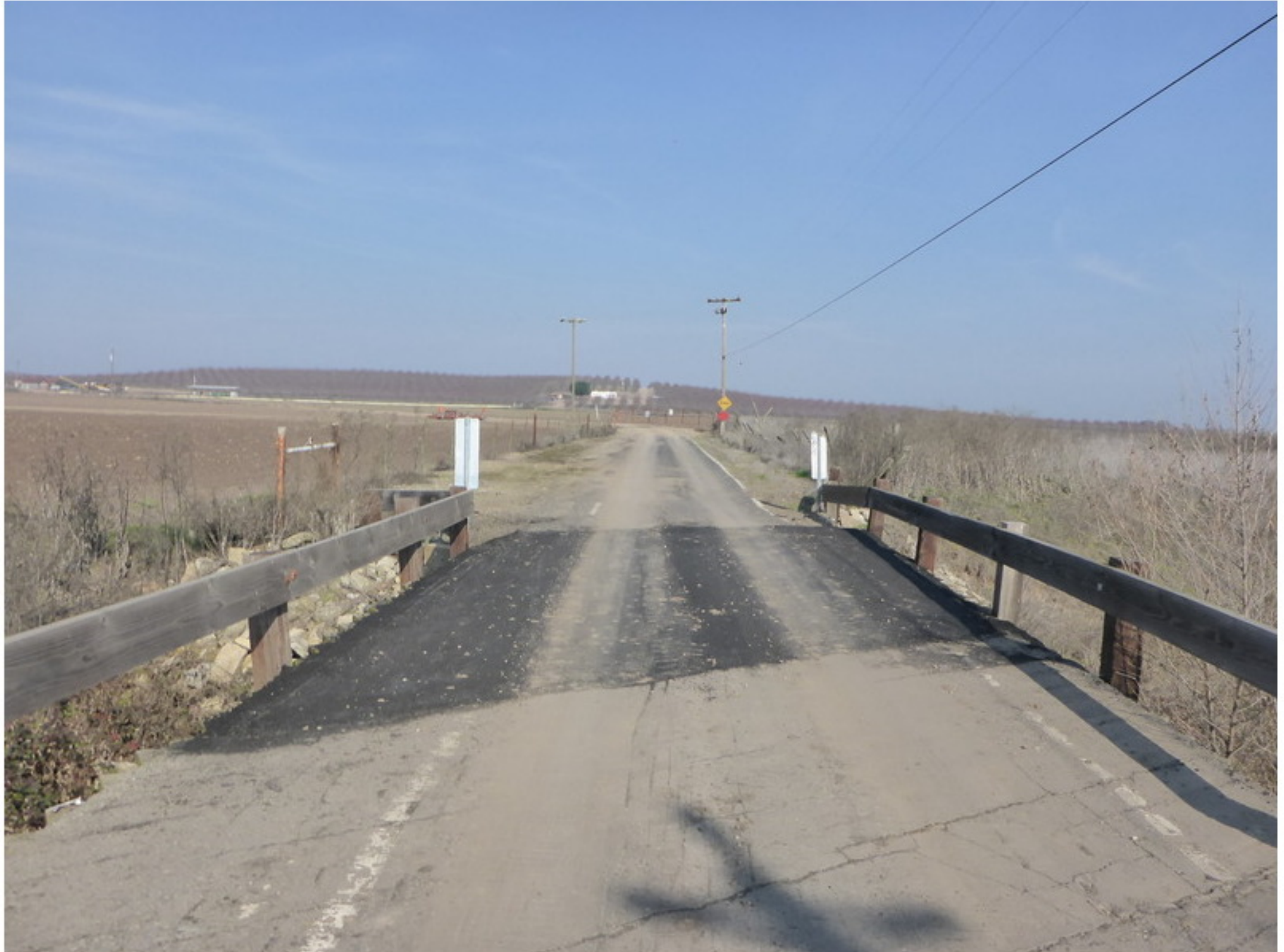
Photo No. 7 New AC overlay after repairs at Abutment 4. Looking north.
