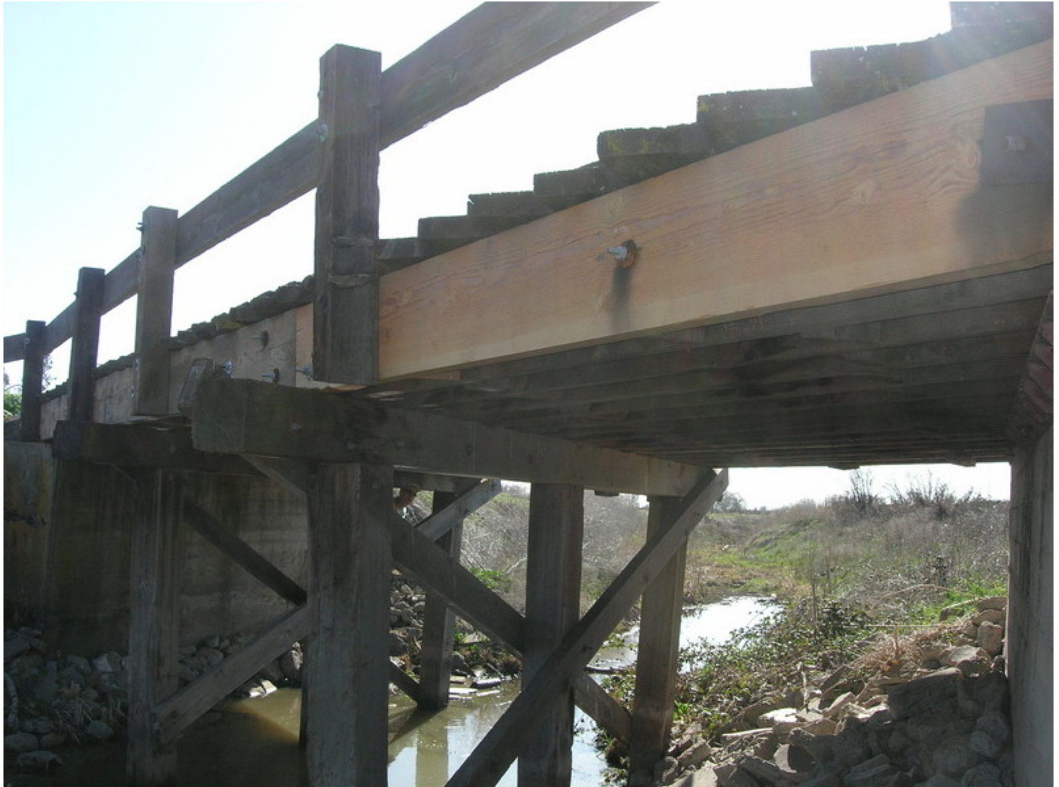
Photo No. 3 New right exterior stringers in all three spans.
