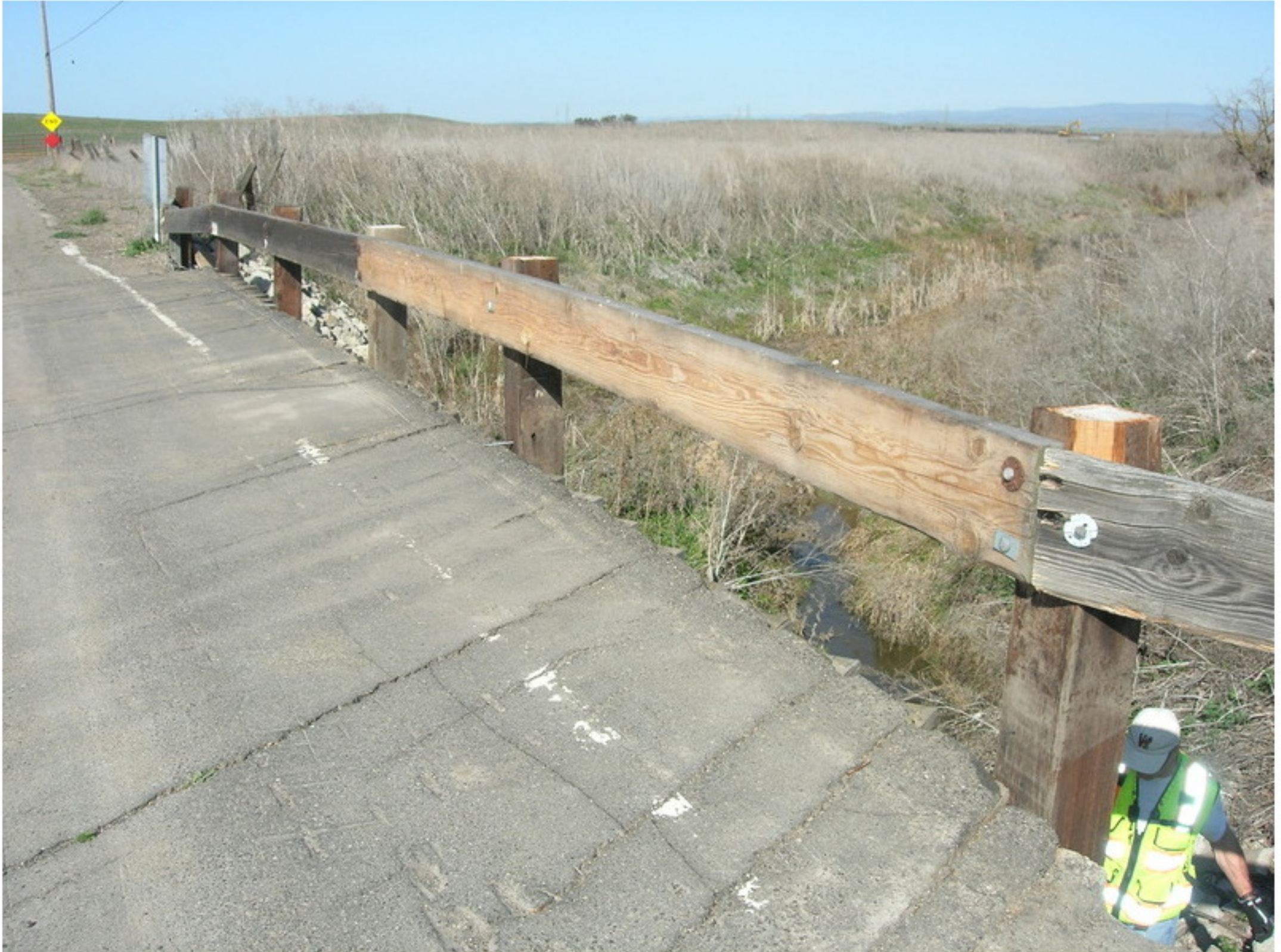
Photo No. 1 New timber rail on the right side.
