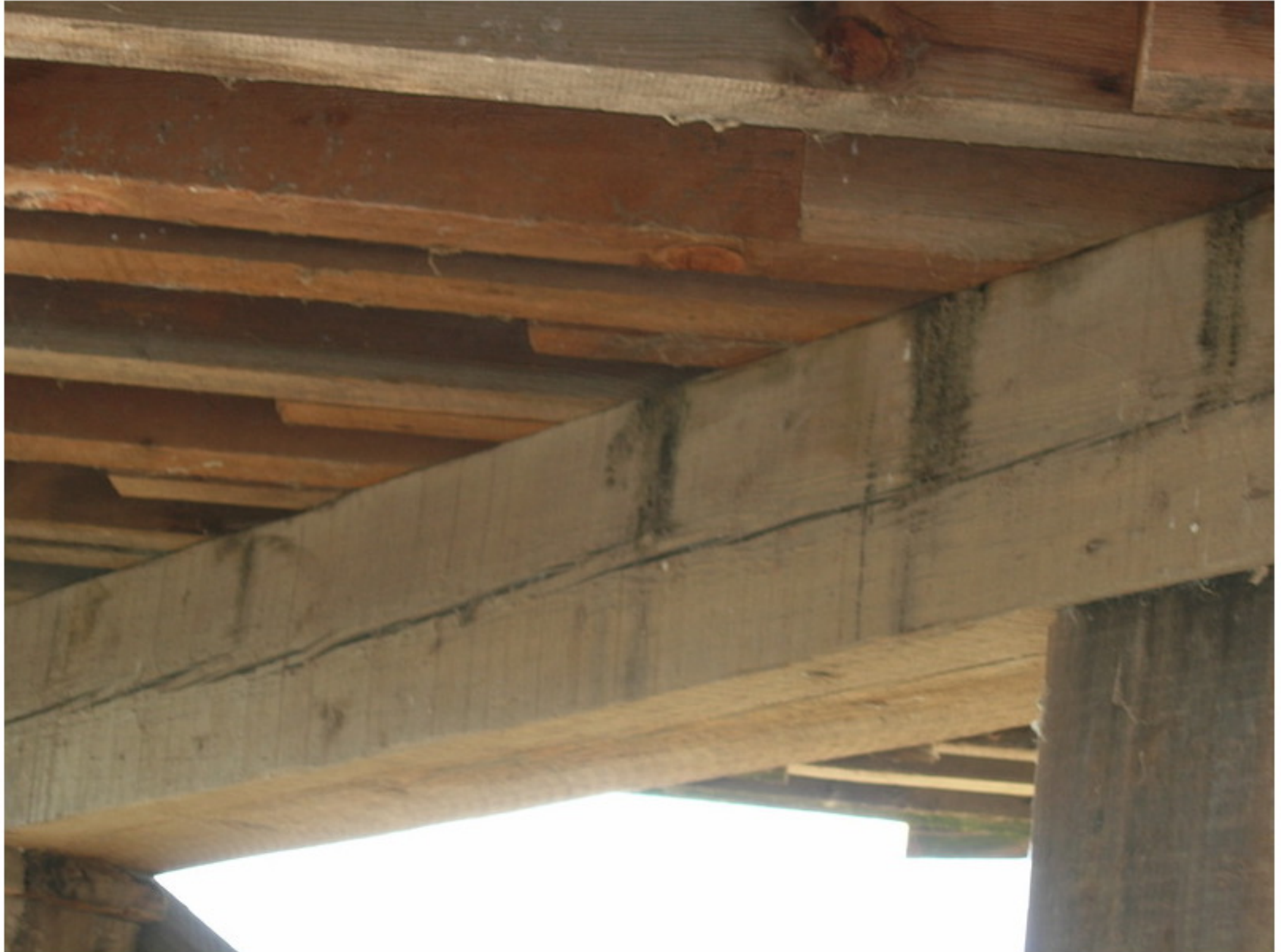
Photo No. 4 Timber cap at Bent 3.
