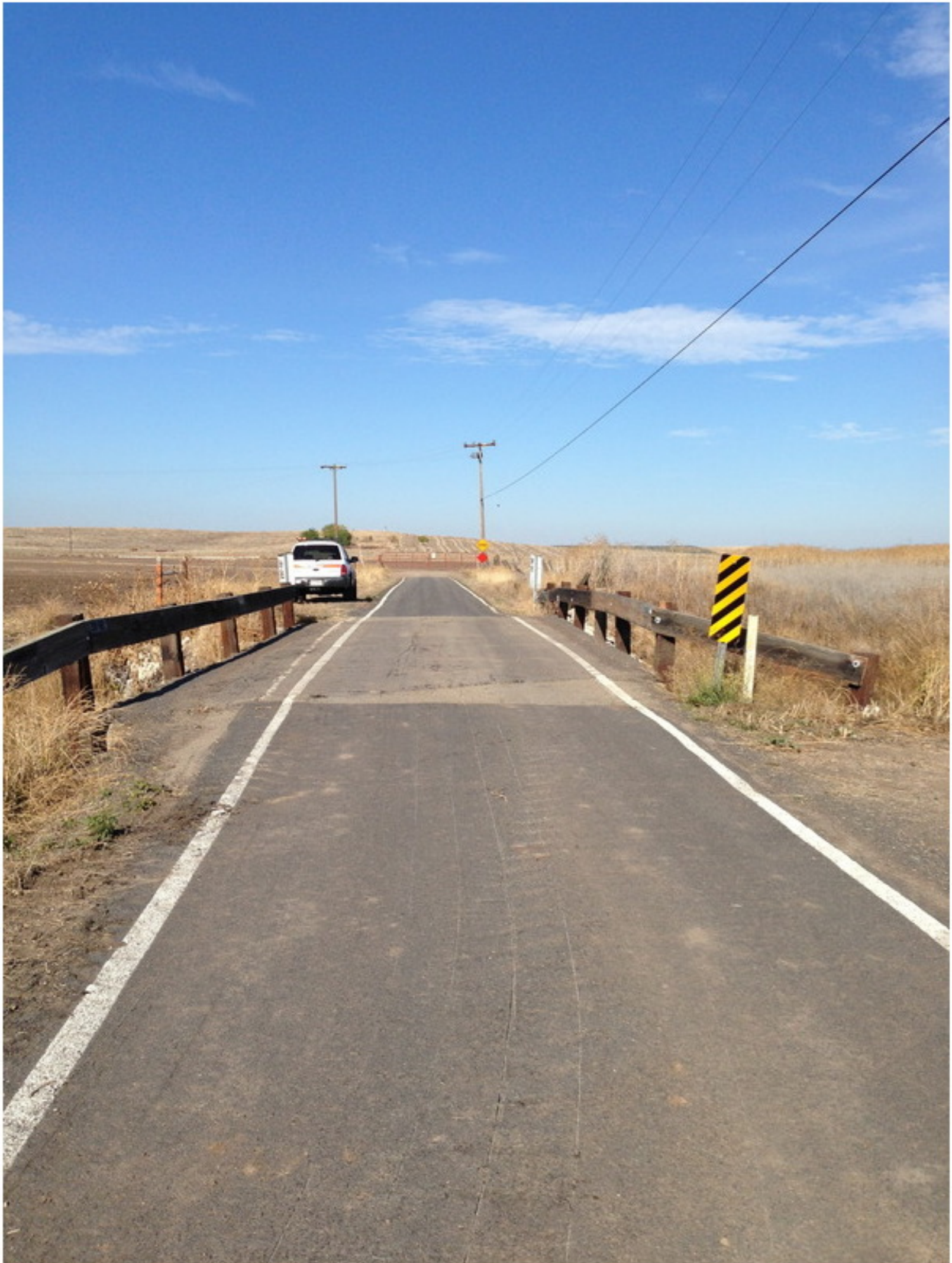
Photo No. 1 Roadway looking north.
