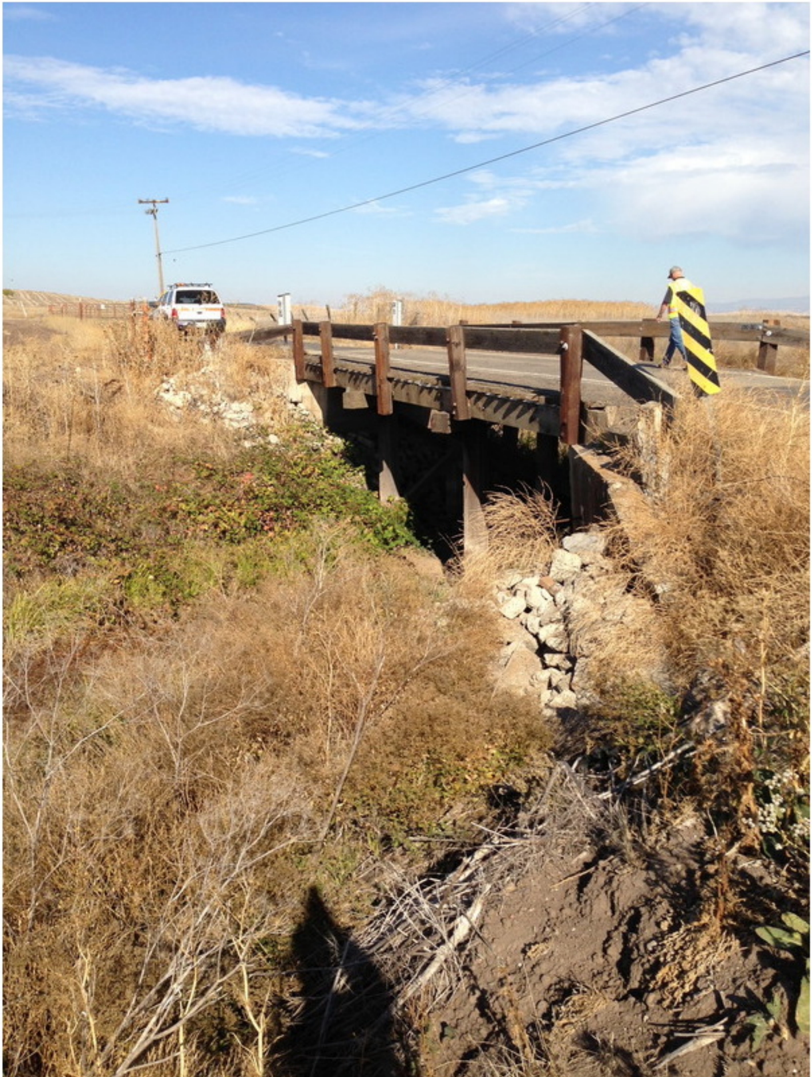
Photo No. 2 Elevation looking northeast.
