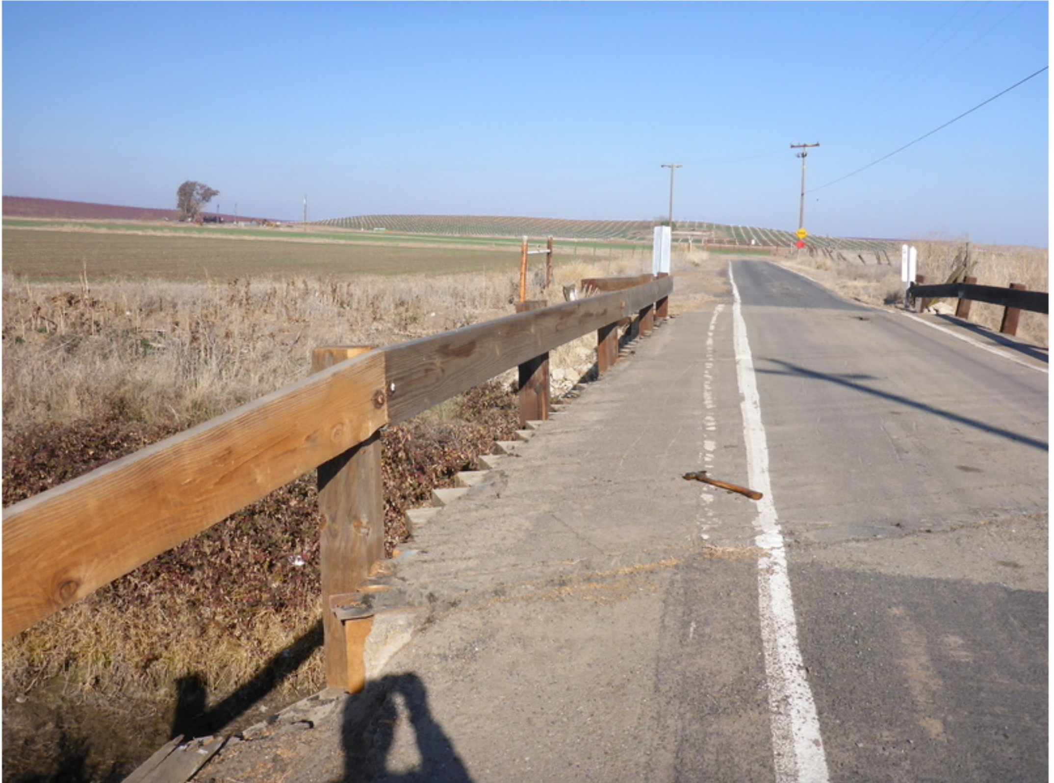
Photo No. 1 New left timber rail
