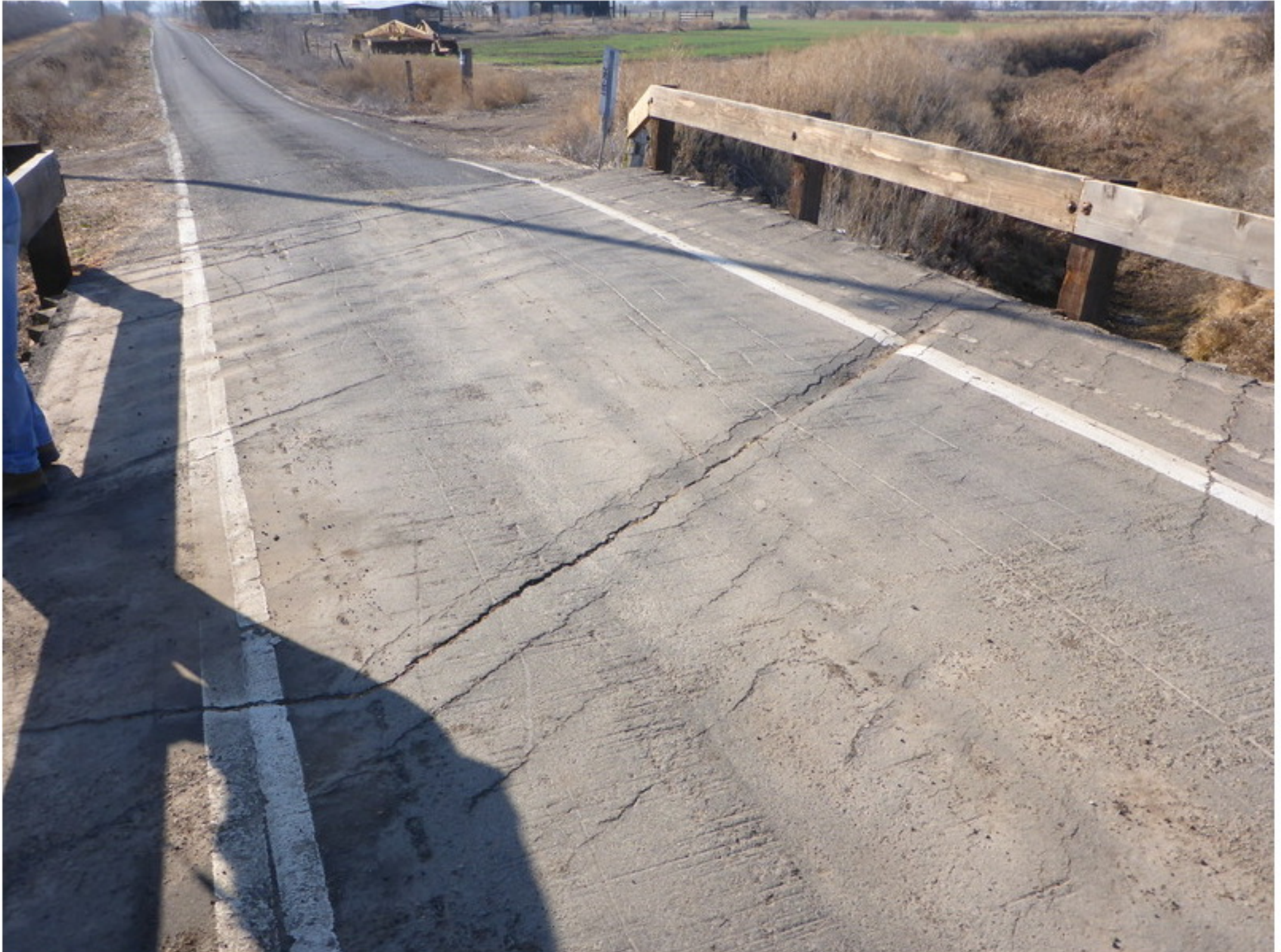
Photo No. 2 Rotten deck board in the middle of the bridge
