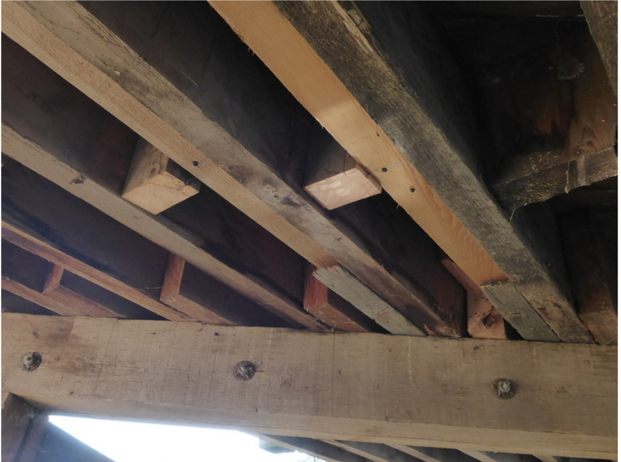
Photo No. 11 Supplemental girders (7 and 8) at Bent 3.
