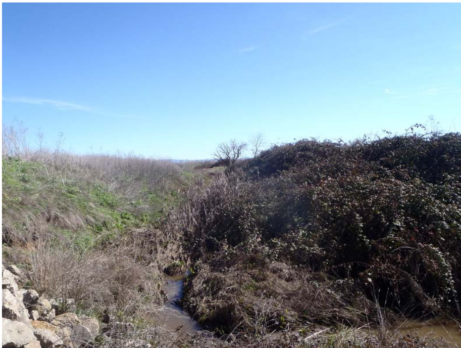
Buckman Road Bridge Replacement Project
