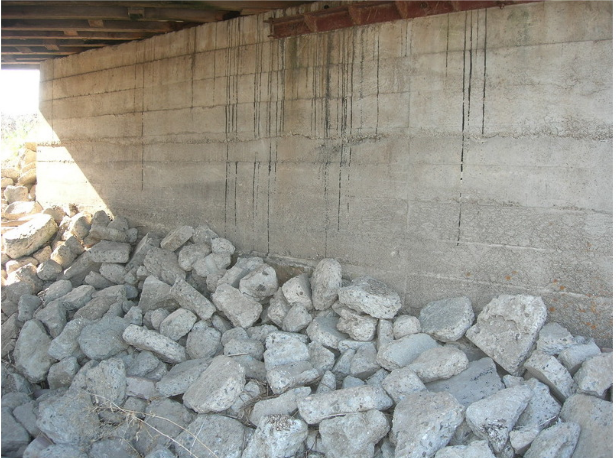
Photo No. 7 View of Abutment 4.
