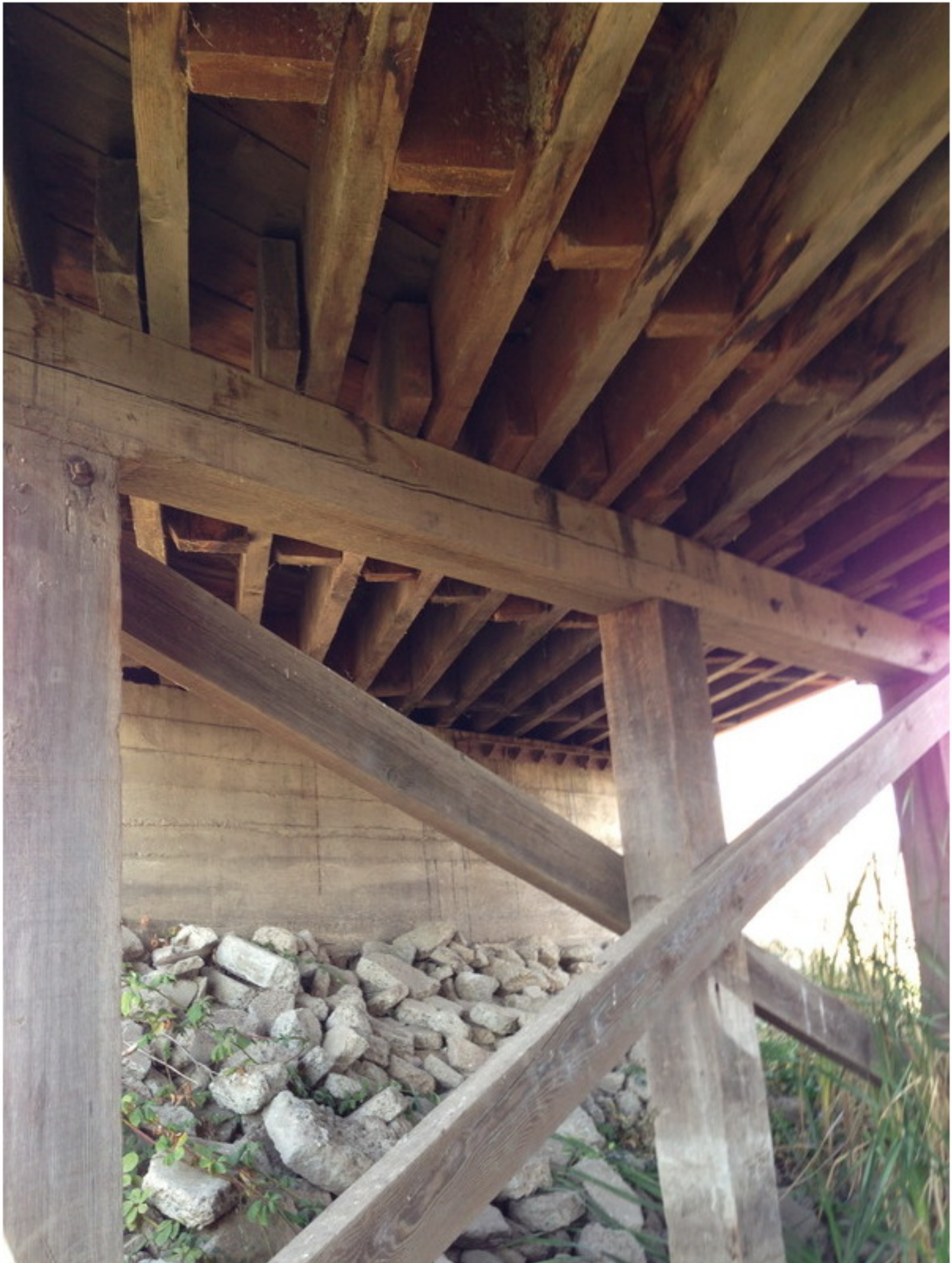
Photo No. 6 Pier 3 Timber Cap.
