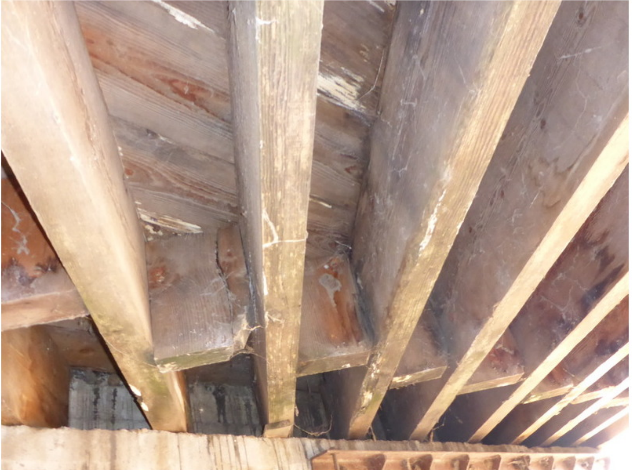
Photo No. 8 Soffit of deck below Abutment 4, left side
