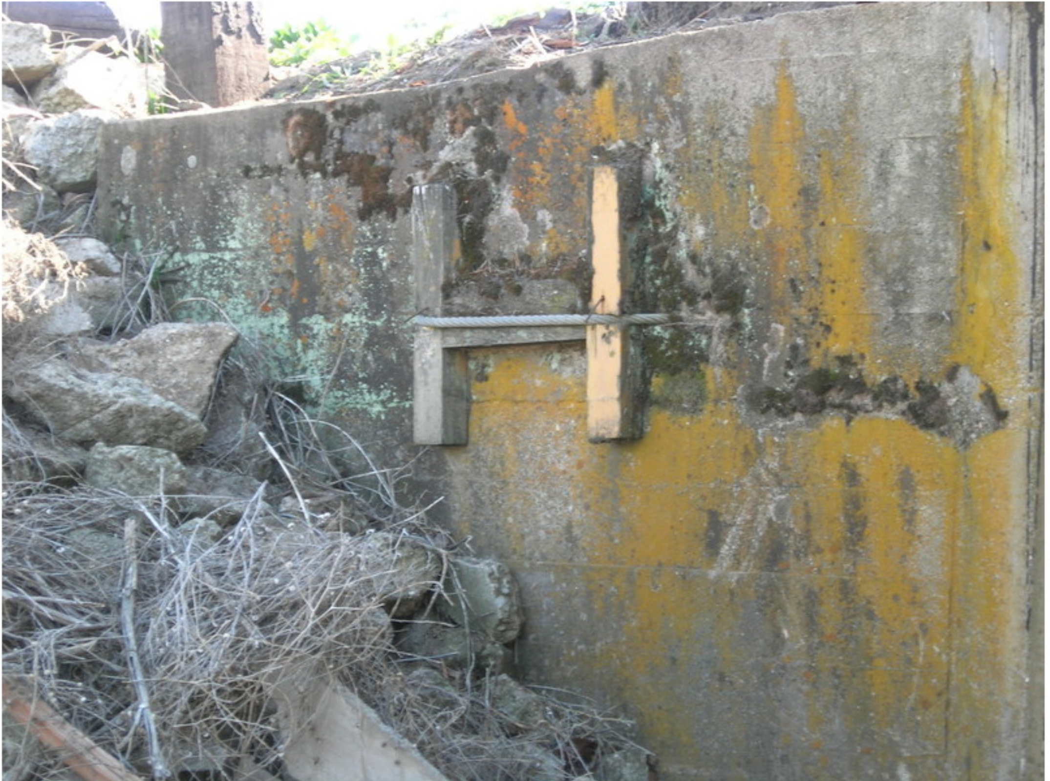
Photo No. 6 Left wingwall at Abutment 1.
