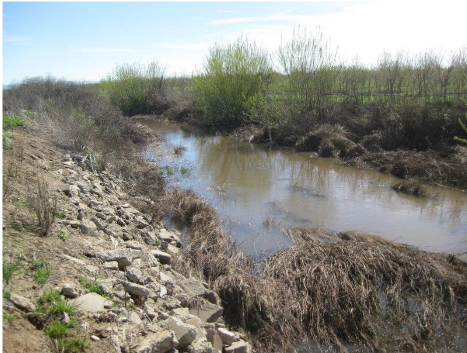
Buckman Road Bridge Replacement Project
