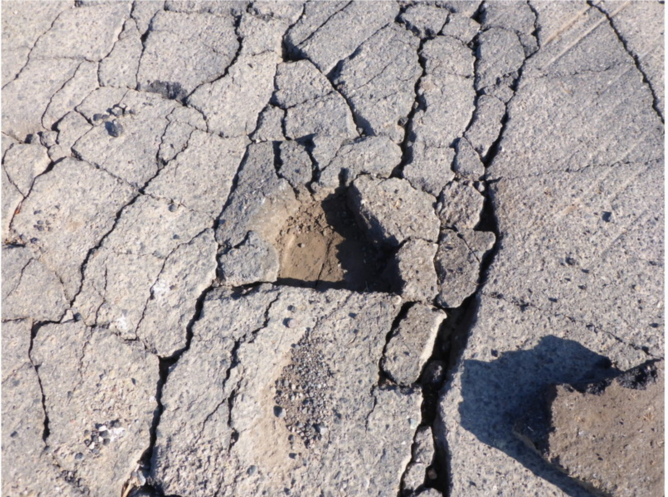
Photo No. 5 Bridge deck at Abutment 4, left side
