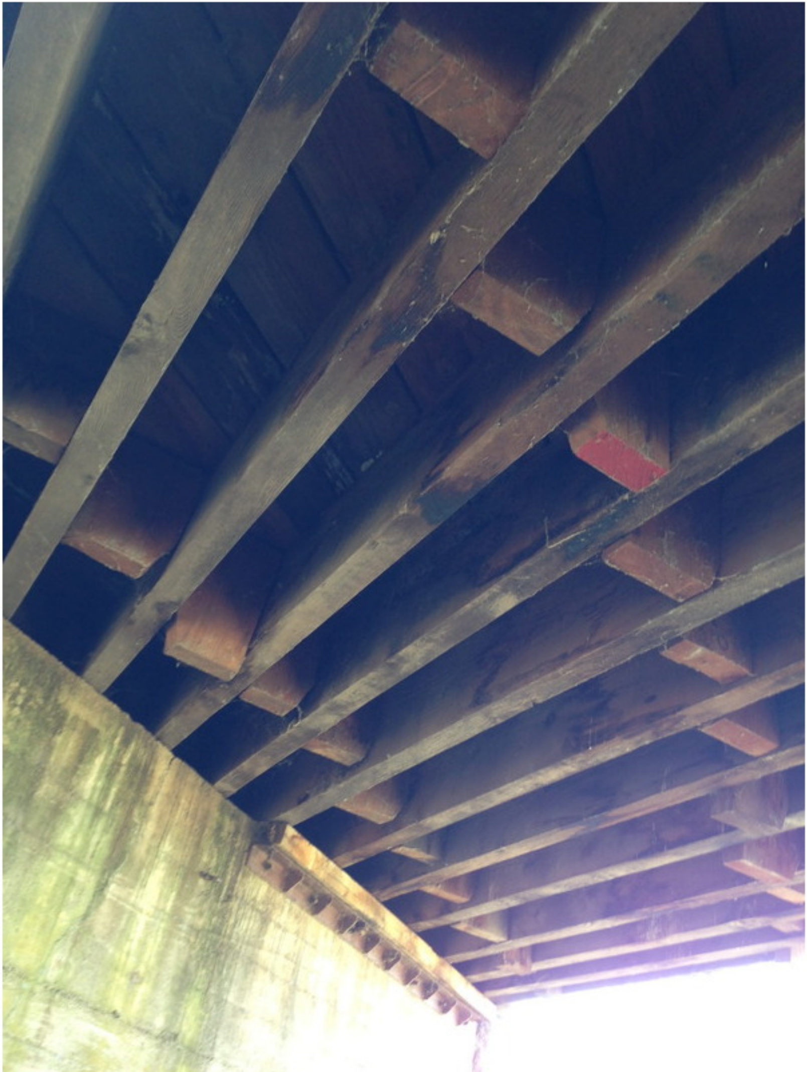
Photo No. 3 Underside Span 1.
