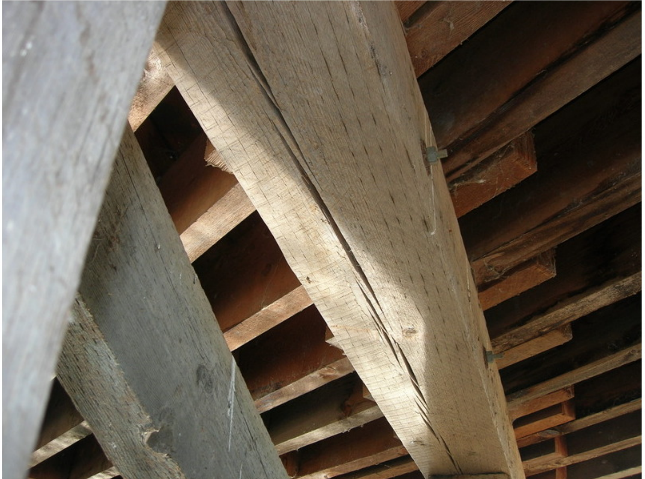
Photo No. 5 Timber cap at Bent 3.
