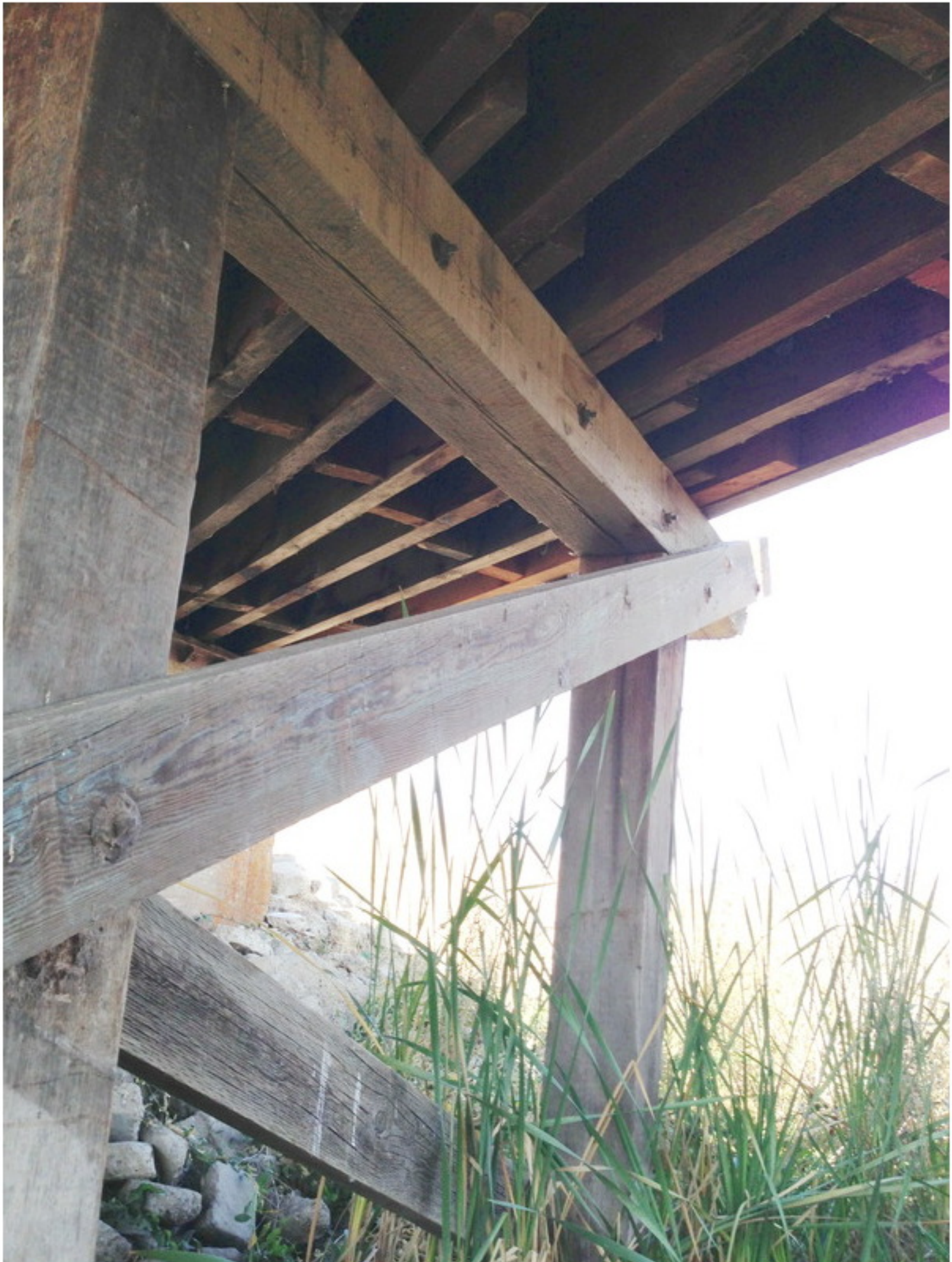
Photo No. 7 Pier 3 Timber Cap.
