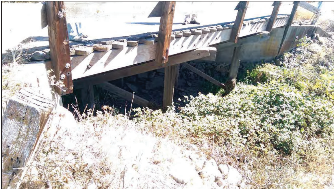
Photo 1. Existing Buckman Road Bridge, Upstream Face
