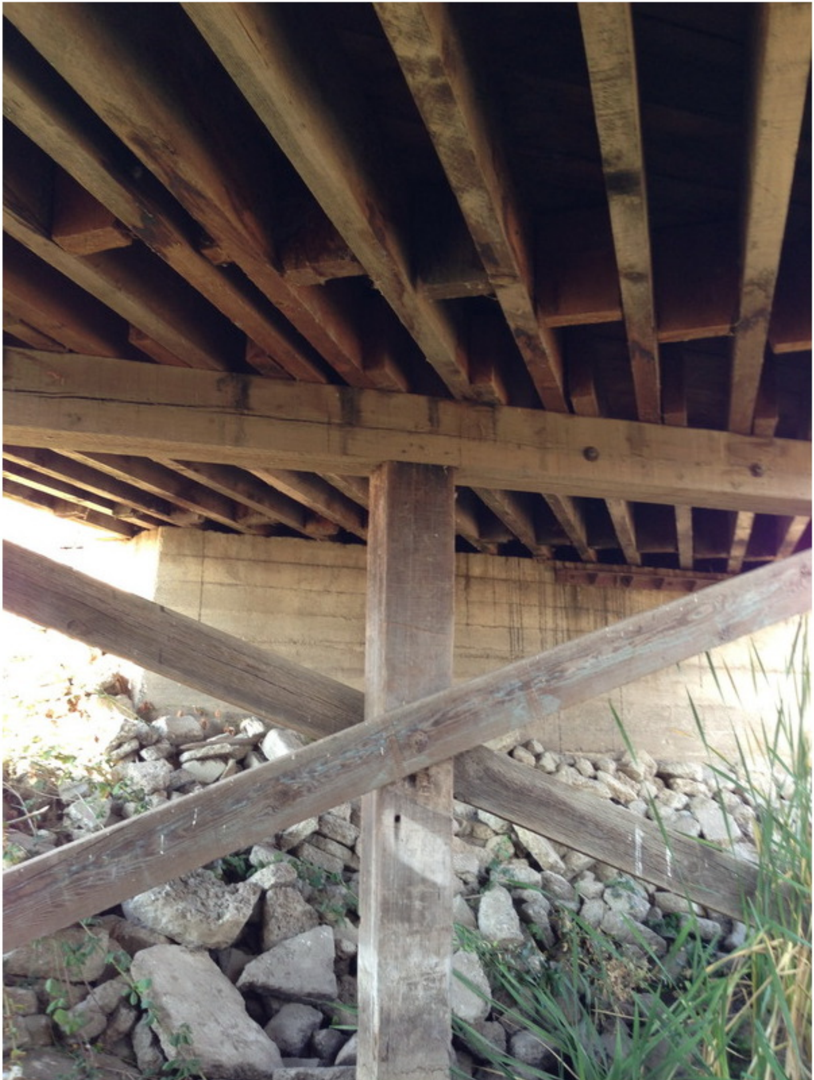
Photo No. 4 Underside Spans 2 and 3.
