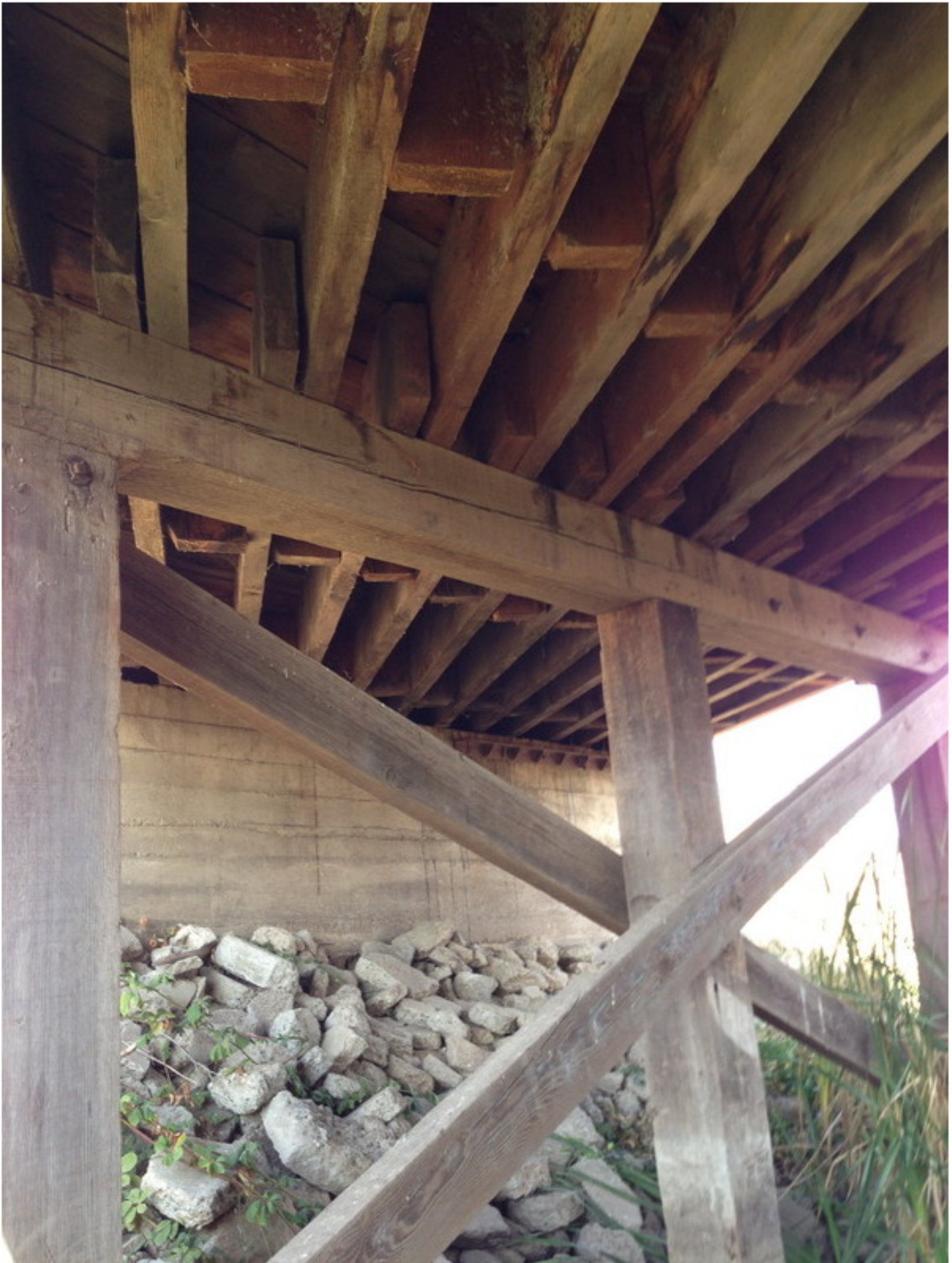
Photo No. 6 Pier 3 Timber Cap.
