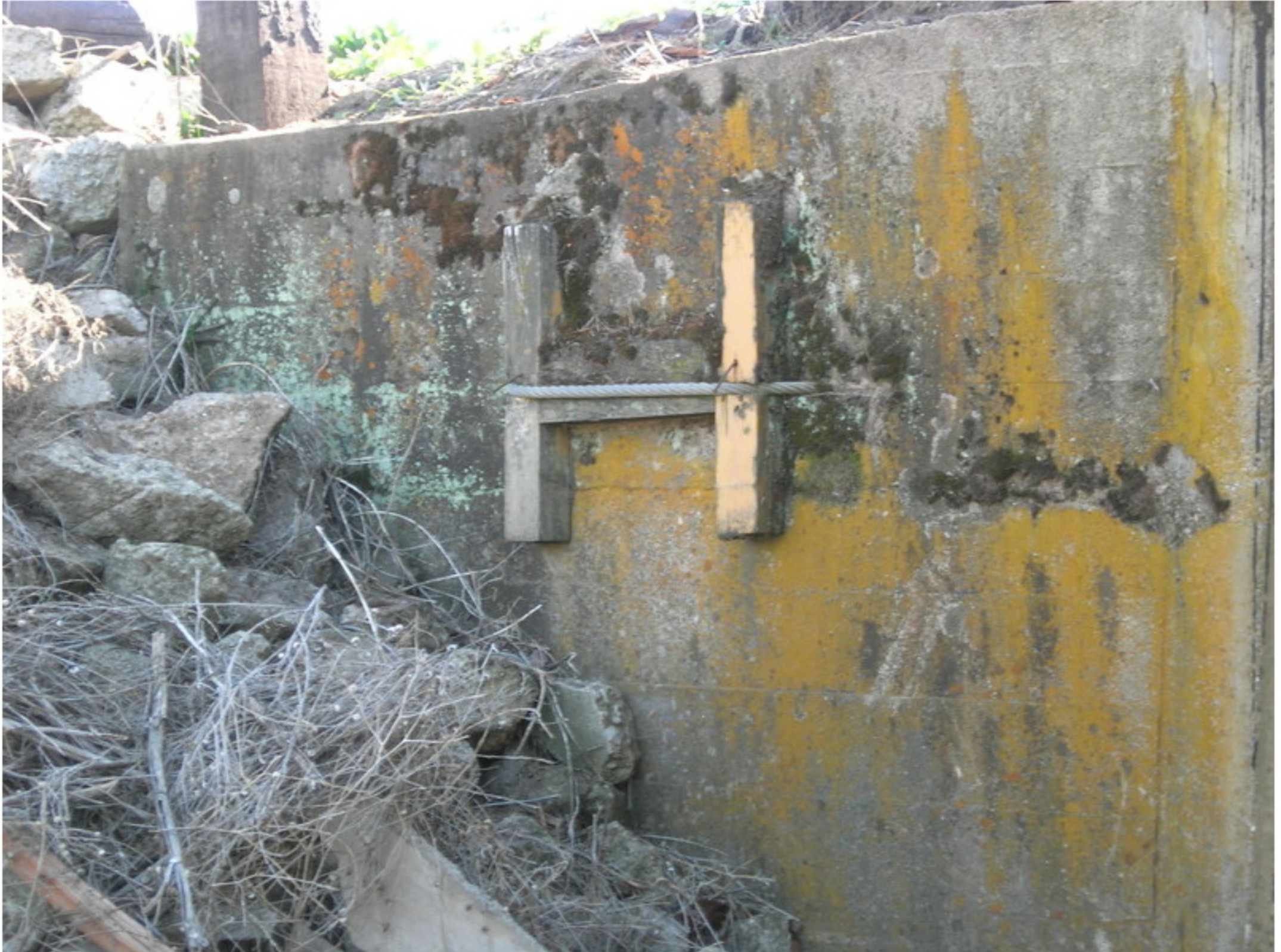
Photo No. 6 Left wingwall at Abutment 1.
