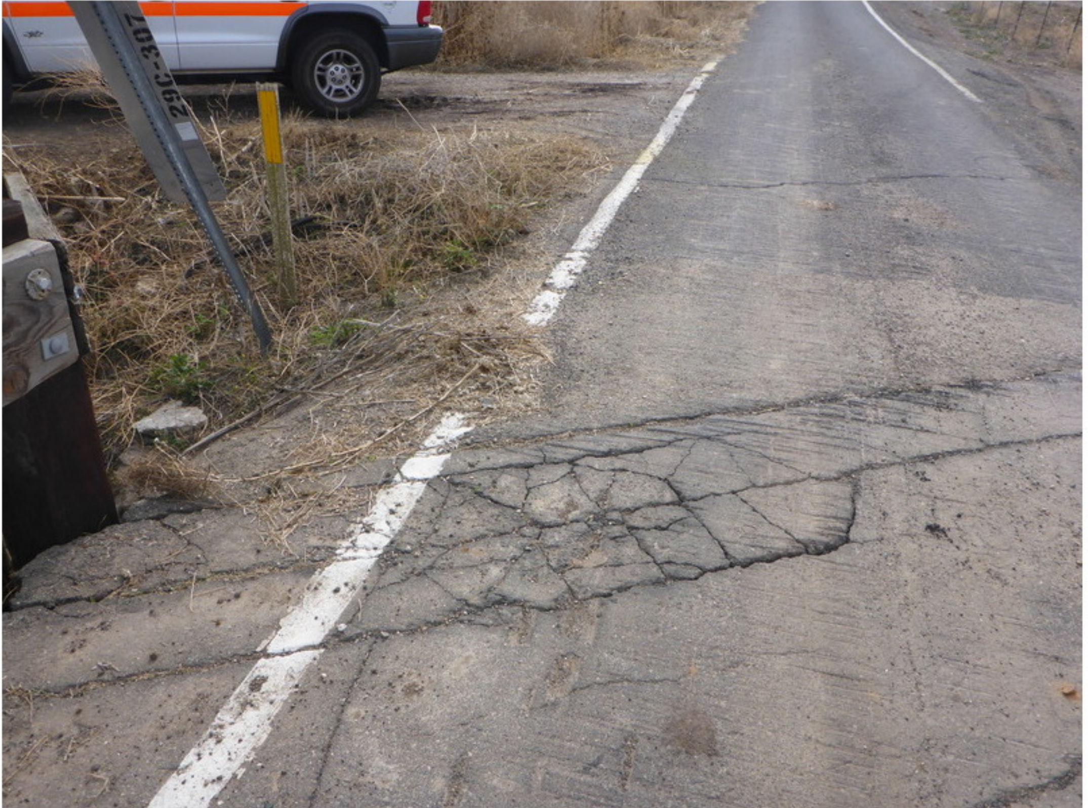
Photo No. 1 Broken up AC at Abutment 1 right.
