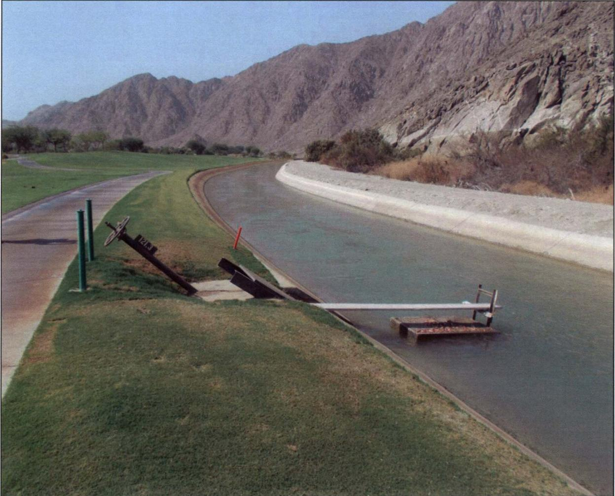
**Figure 2. The lateral at Sta. 6403 + 85.1 is a single-barrel turnout located on the east side of the canal, equipped with a single wheel-type manual gate control (photograph taken August 23, 2013, view to the south).**
