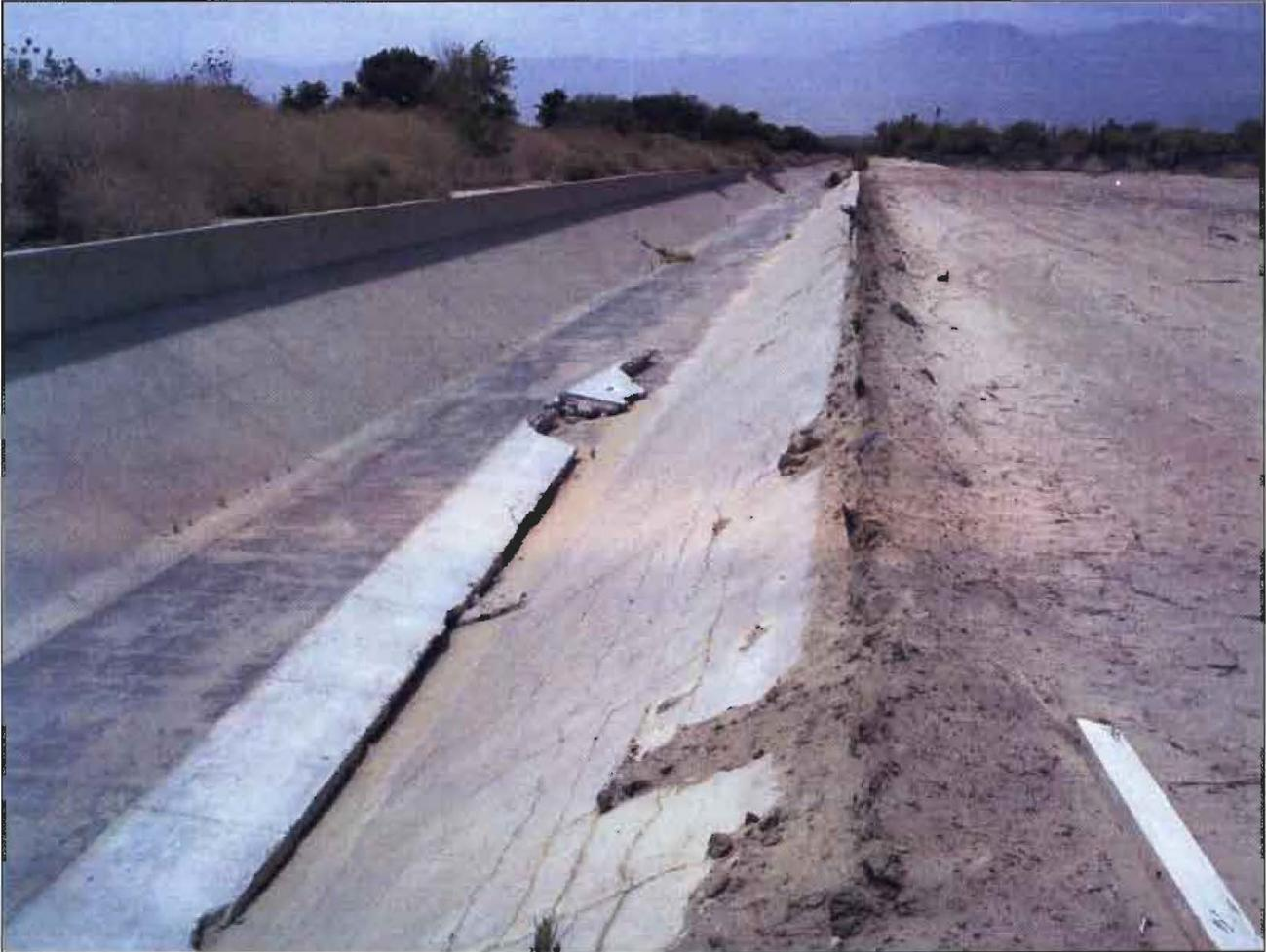
Figure 5. Segment of Wasteway No. 3 on Cabazon Indian Reservation (view to the southwest). Note the collapsed wall laying in the bottom of the wasteway.
