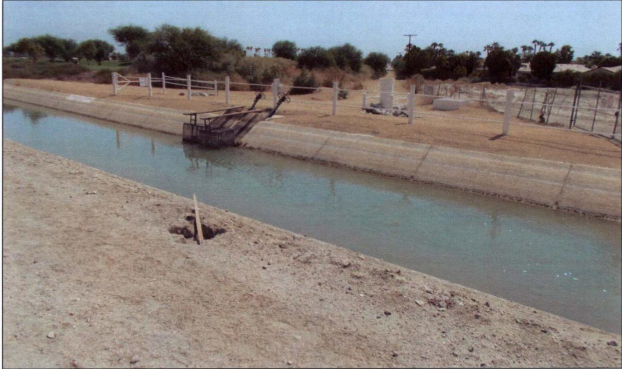
**Figure 3. The lateral at Sta. 6420 + 115 (Lateral 121.6) is a double-barrel turnout located on the east side of the canal. It is equipped with two wheel-type manual gate controls. An irrigation standpipe is visible in the distance (photograph taken August 23, 2013, view to the east toward the alignment of Avenue 54).**
