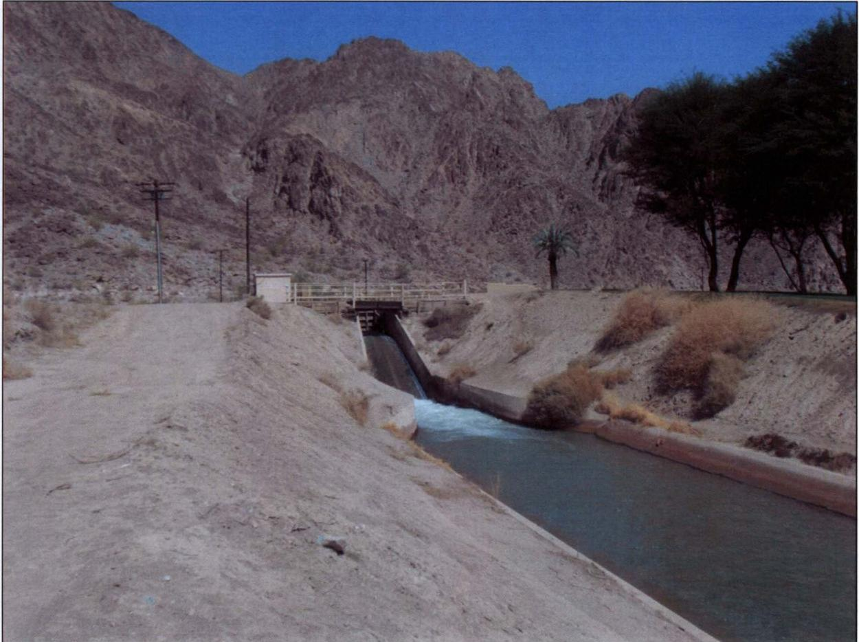
**Figure 4.** A large check dam/drop structure at Sta. 6426 + 40.1 (photograph taken August 23, 2013, view to the northwest). The drop structure at Sta. 6426 + 40.1 features a vehicle crossing bridge over the top of the spillway, supported at each end with concrete buttresses and with a deck of wood planks. A small concrete-block power supply and control room building sits on the west side of the canal at this location.
