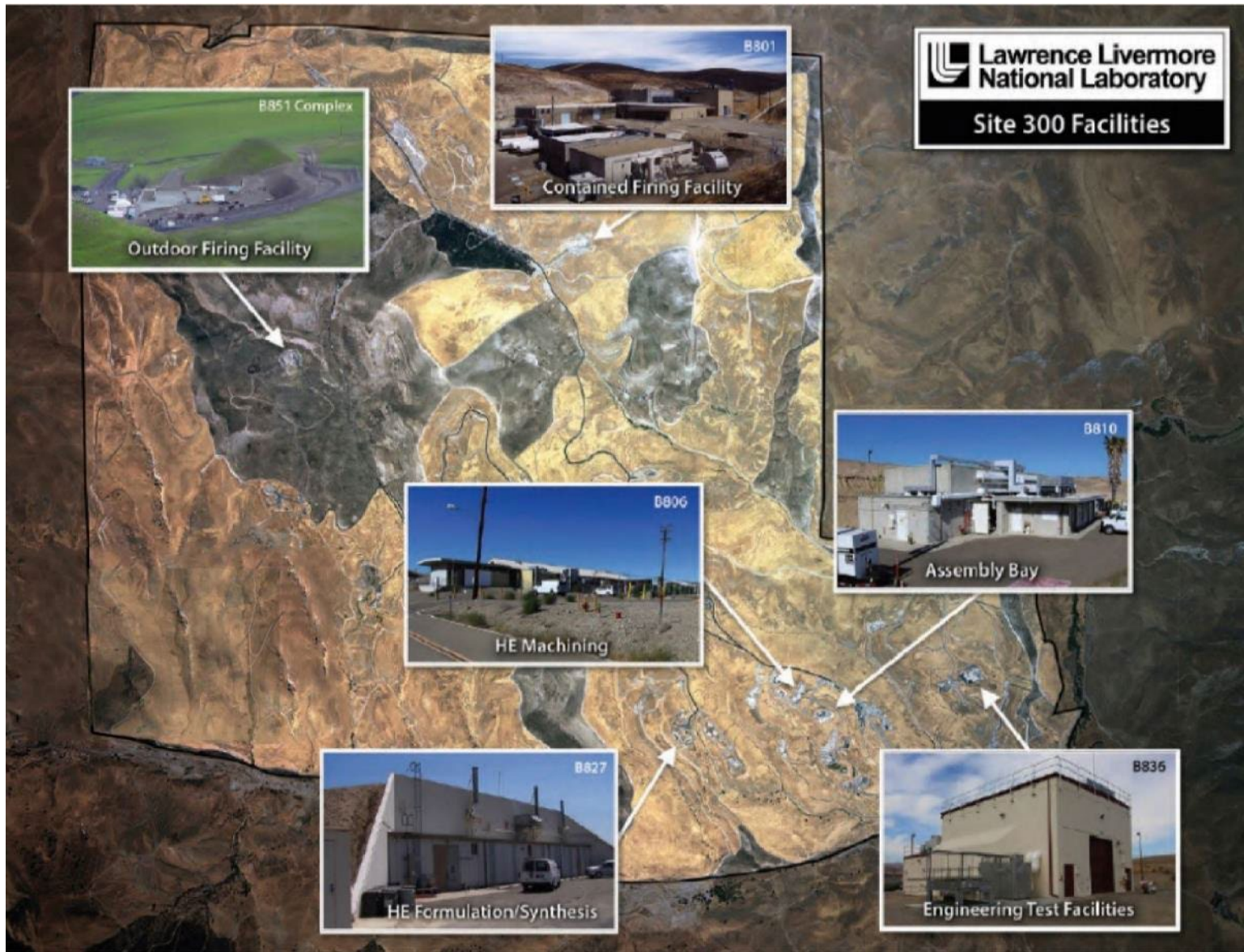
Figure S.2-4. Notable Facilities at Site 300
