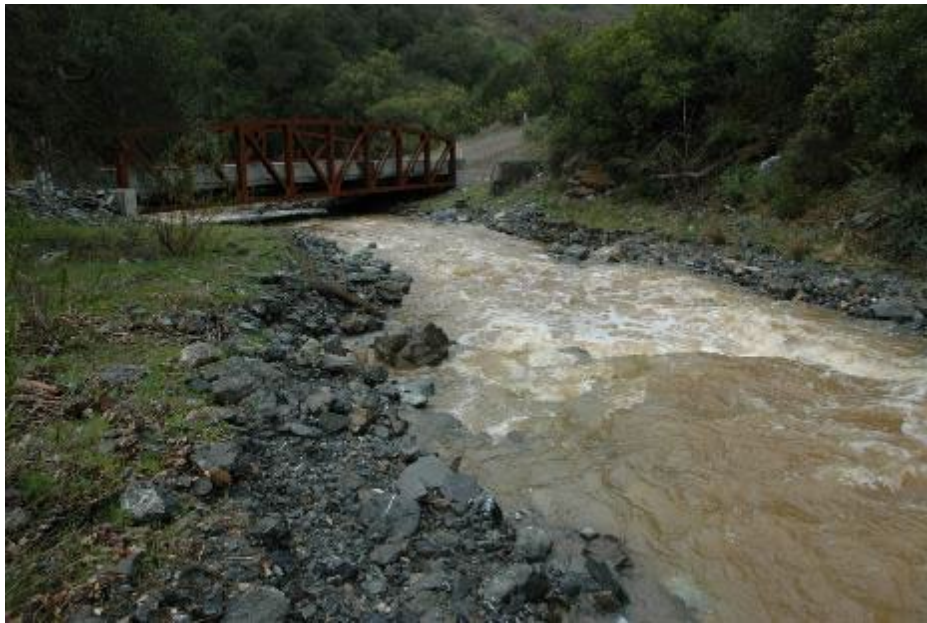
Figure E-9. Flooding Event at Arroyo Mocho
