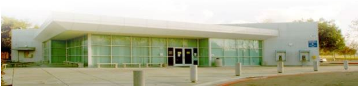
Figure 2-10. West Gate Badge Office
