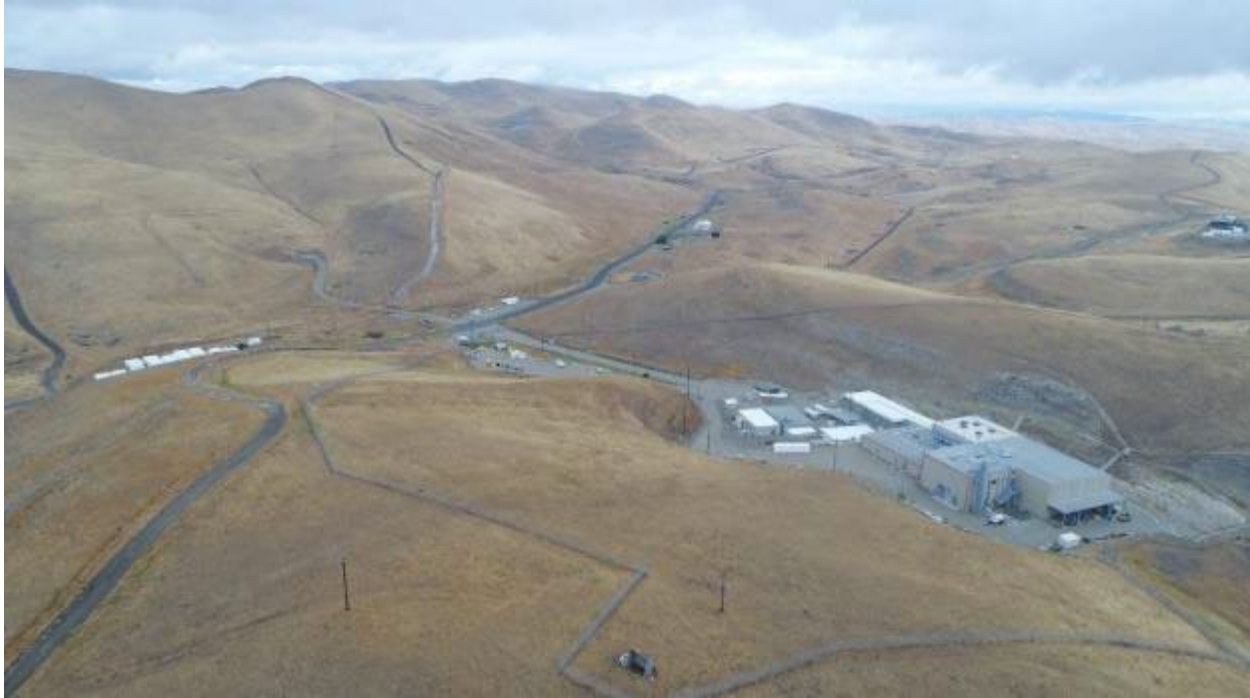
Figure 4-23. Typical Aerial View of Site 300 Area
