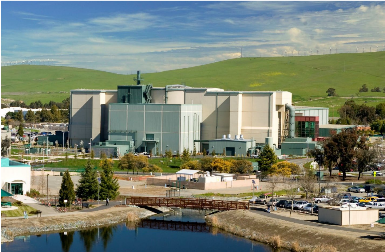
Figure 4-22. View of the NIF Looking Northeast
