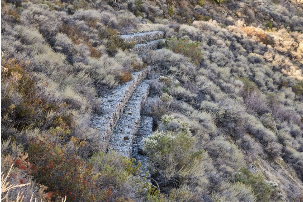
Figure 4-27. Gabion Retaining Walls
