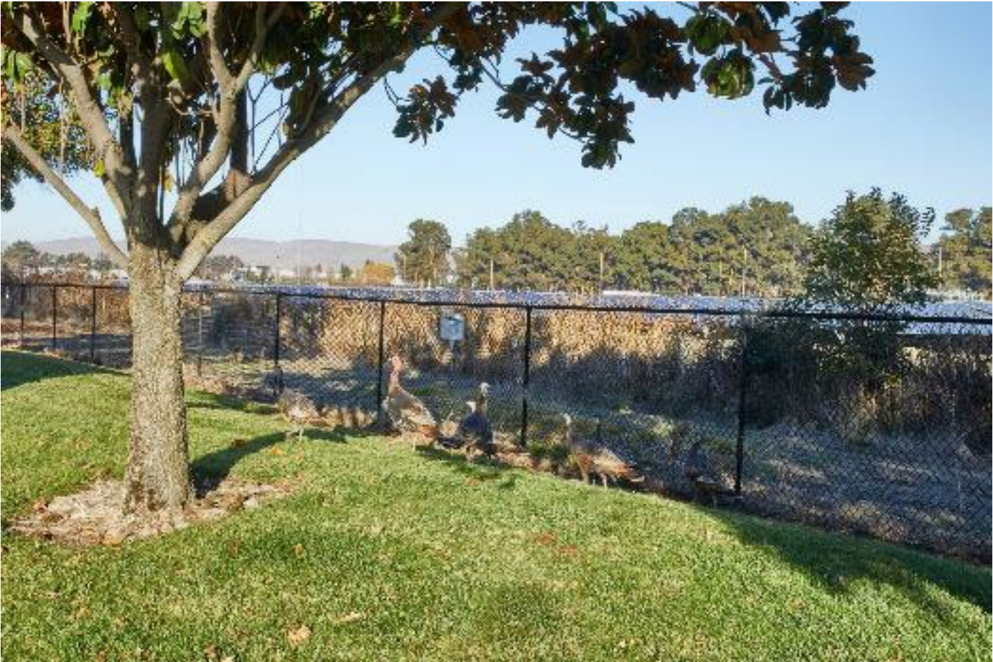
Figure 4-16. View of Solar Array from Outside Fence Line
