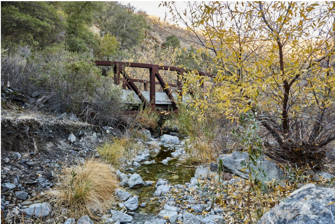
Figure 4-28. Steel Bridge to Arroyo Mocho Pump Station
