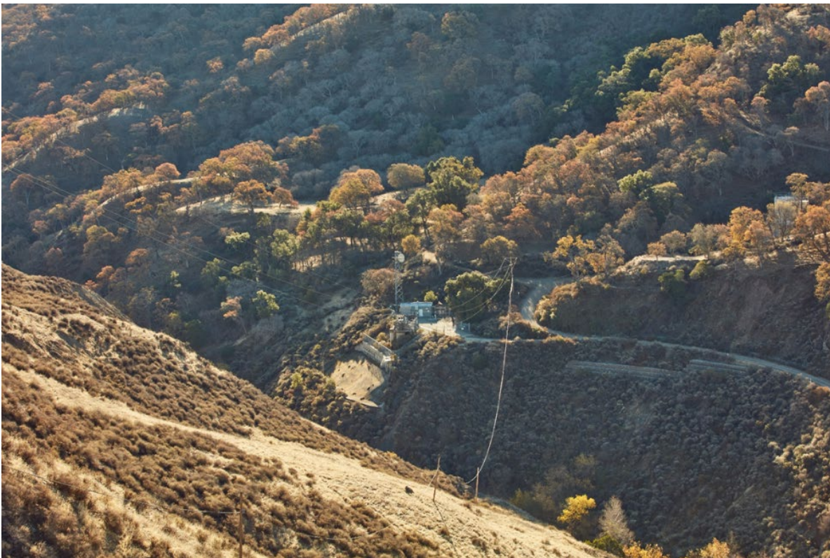
Figure 4-26. Arroyo Mocho Pump Station
