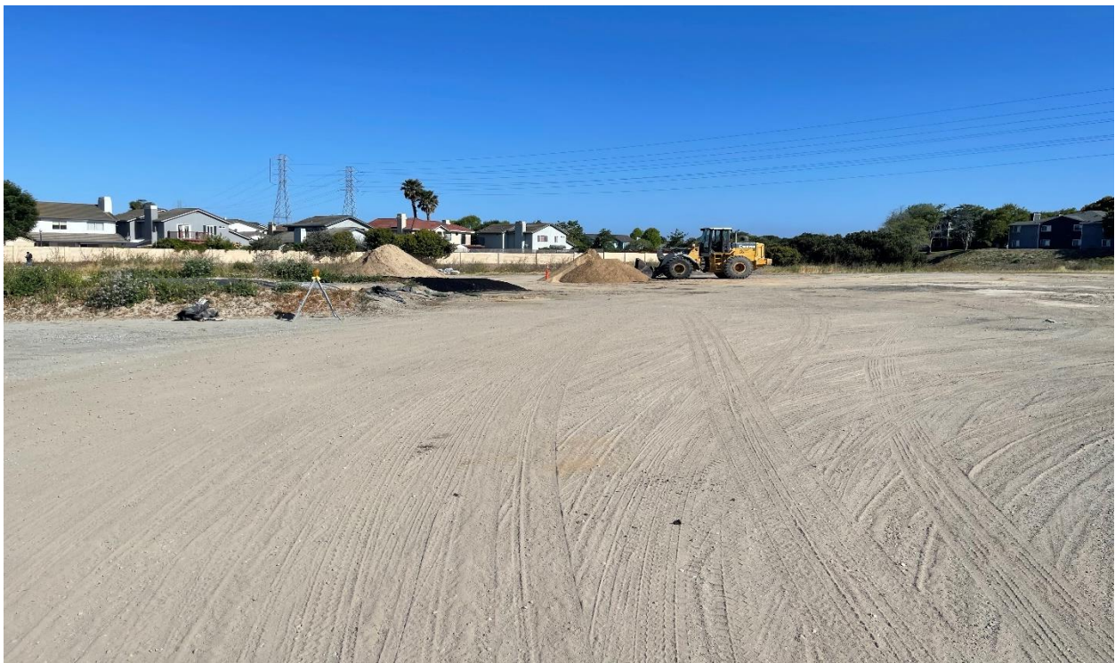
Photograph 2. The southwest corner of the study area, facing north. Soil stockpiles in the midground.
