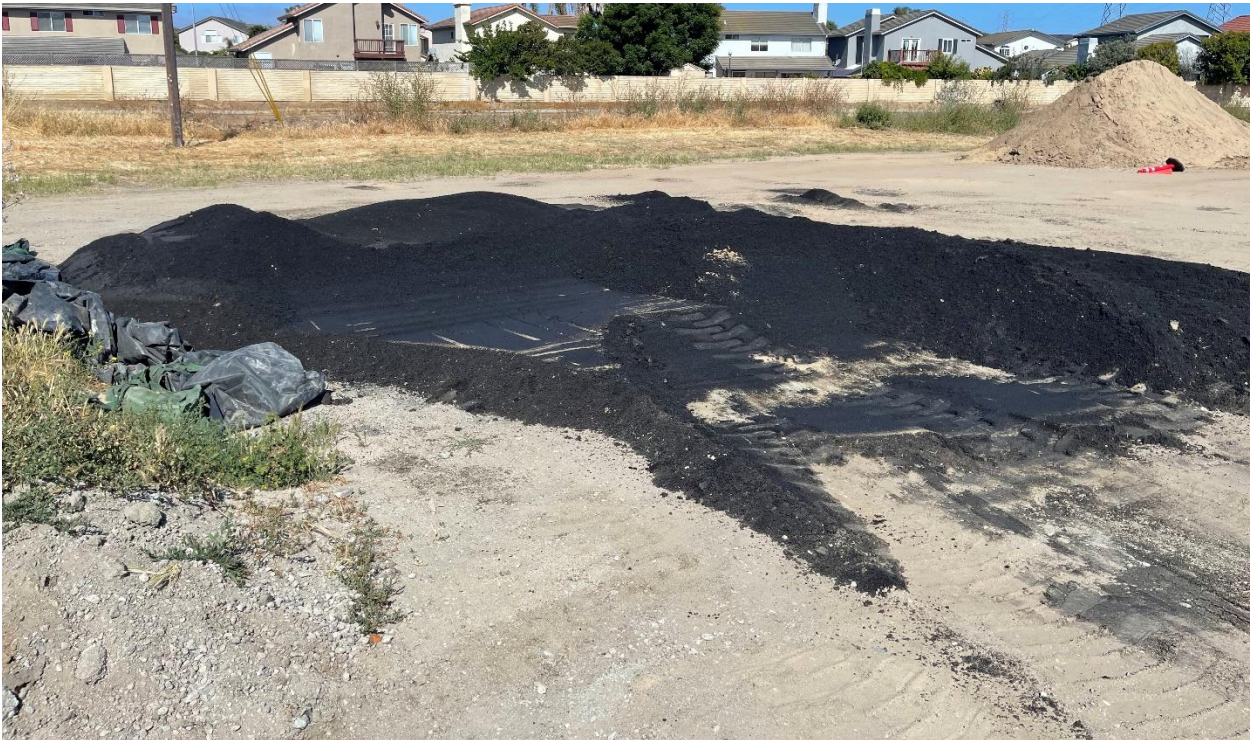
Photograph 6. Soil and gravel stockpiles along the western edge of the study area.
