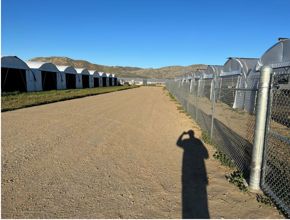
Photo 3 – Southeast corner of expansion area, west.
