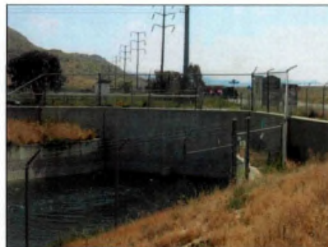
San Diego Canal siphon, facing southwest.
