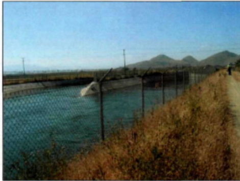
Casa Loma Canal divider, facing southeast.
