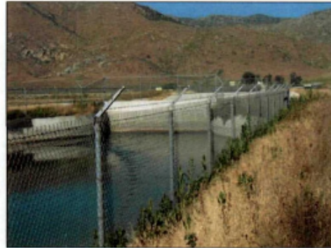
Casa Loma Canal siphon, facing west.
