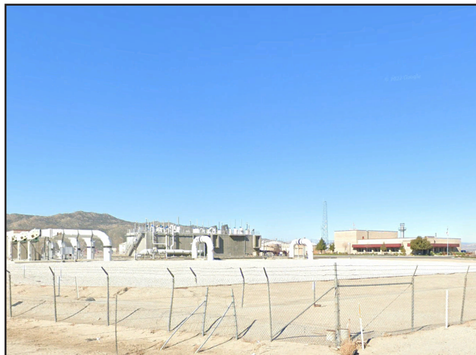
View 5: Looking northwest towards the San Jacinto Valley Regional Water Reclamation Facility.
