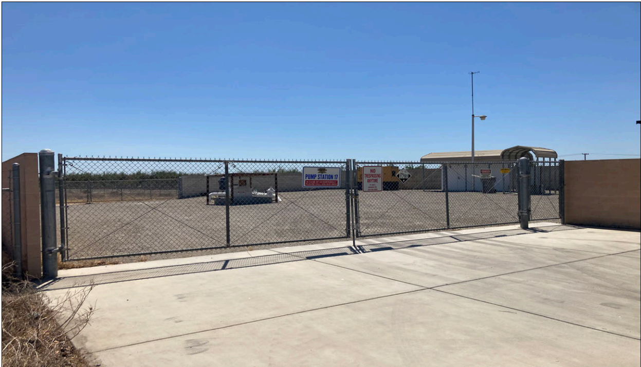
Figure 11. Photograph of the Lift Station Number 17 site, looking southeast from South Goldenrod Avenue.
