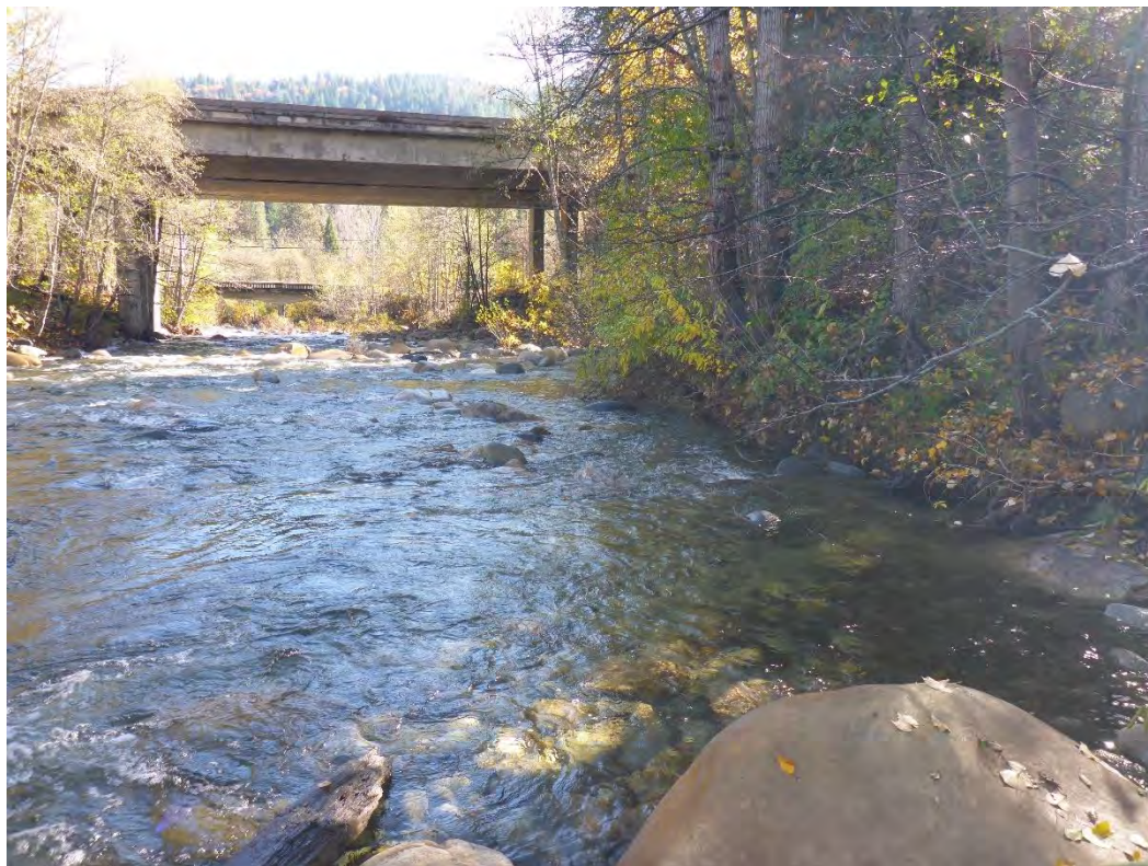
Castle Creek (1:PS), view to the east toward Interstate 5 overpass.
