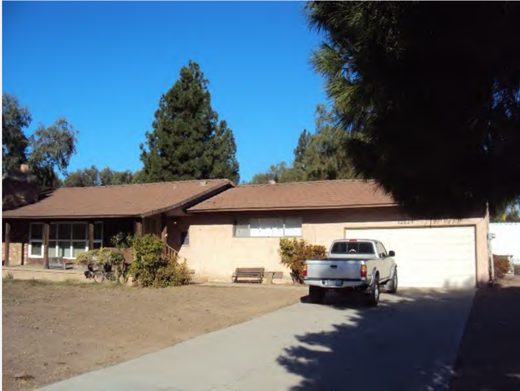
Exhibit D. 12624 Oak Knoll Road. Primary (south) elevation, looking northwest.
