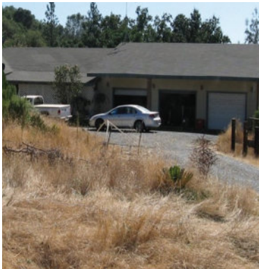
DEFENSIBLE SPACE NONCOMPLIANT
