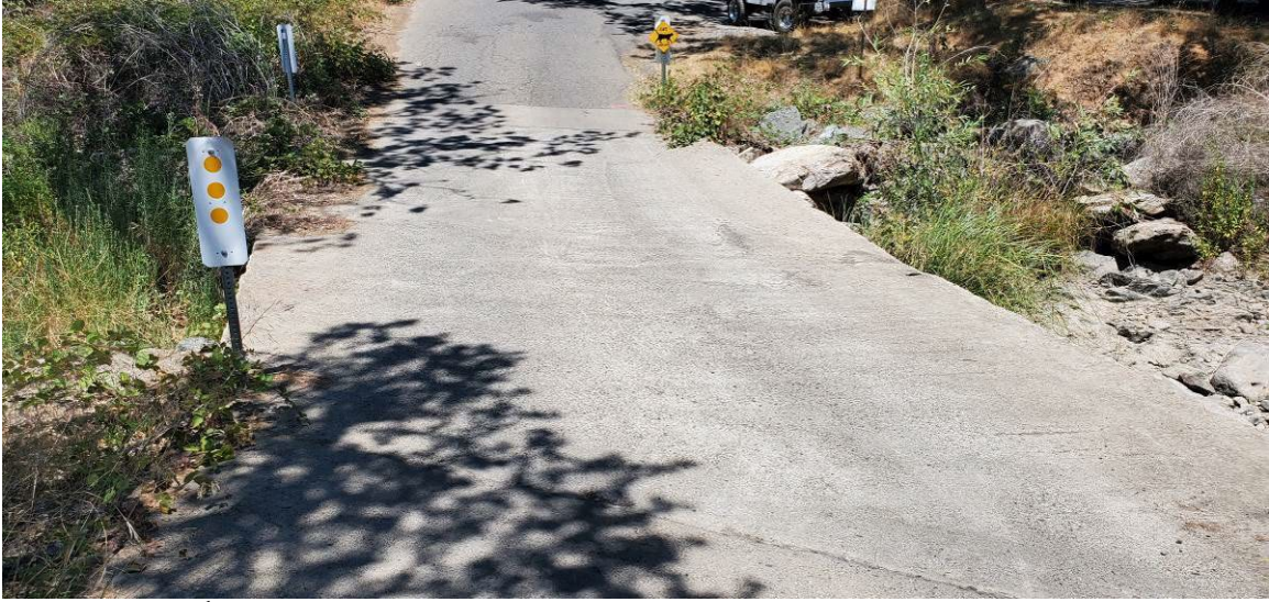
Photo 7: 8 th Street crossing of Mariposa Creek channel. Photo direction: northeast.
