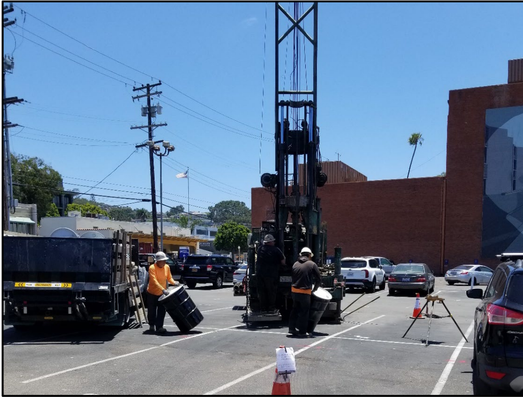
Figure 3-2. Drilling Operations, June 18, 2020
