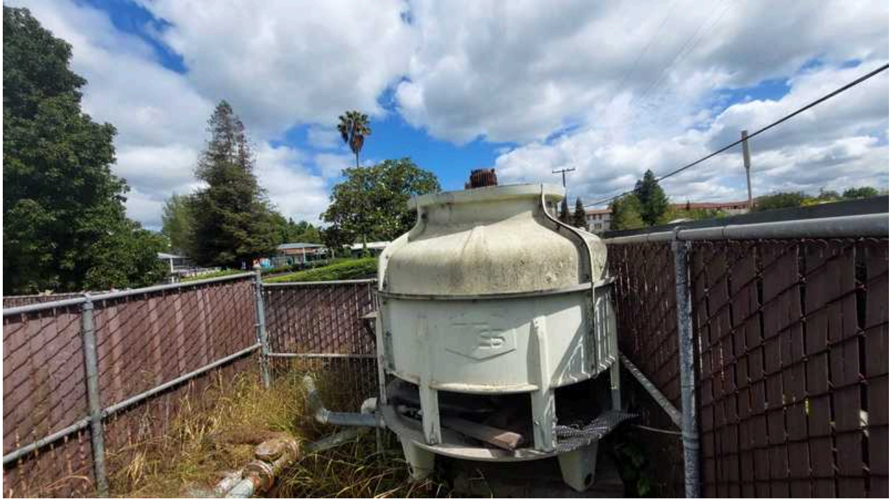
9. View of water cistern, not in use
