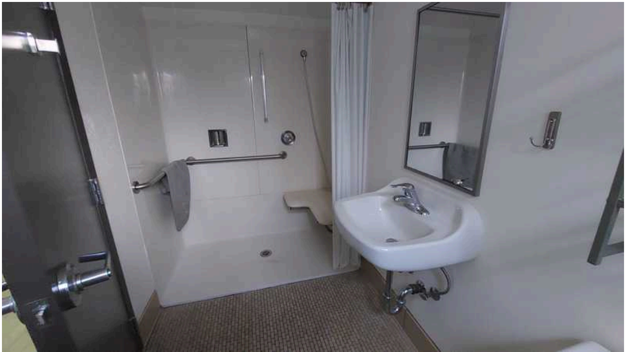
20. View of typical attached shower and sink
