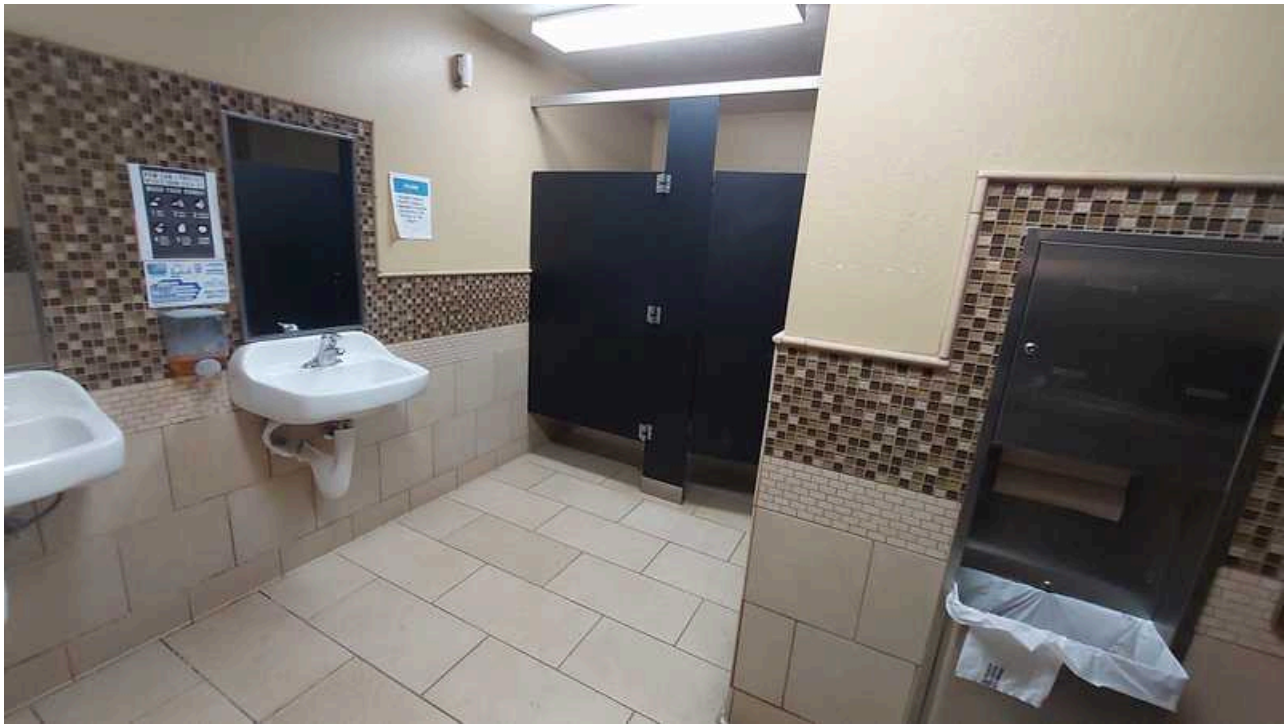
14. View of a restroom inside the subject property building
