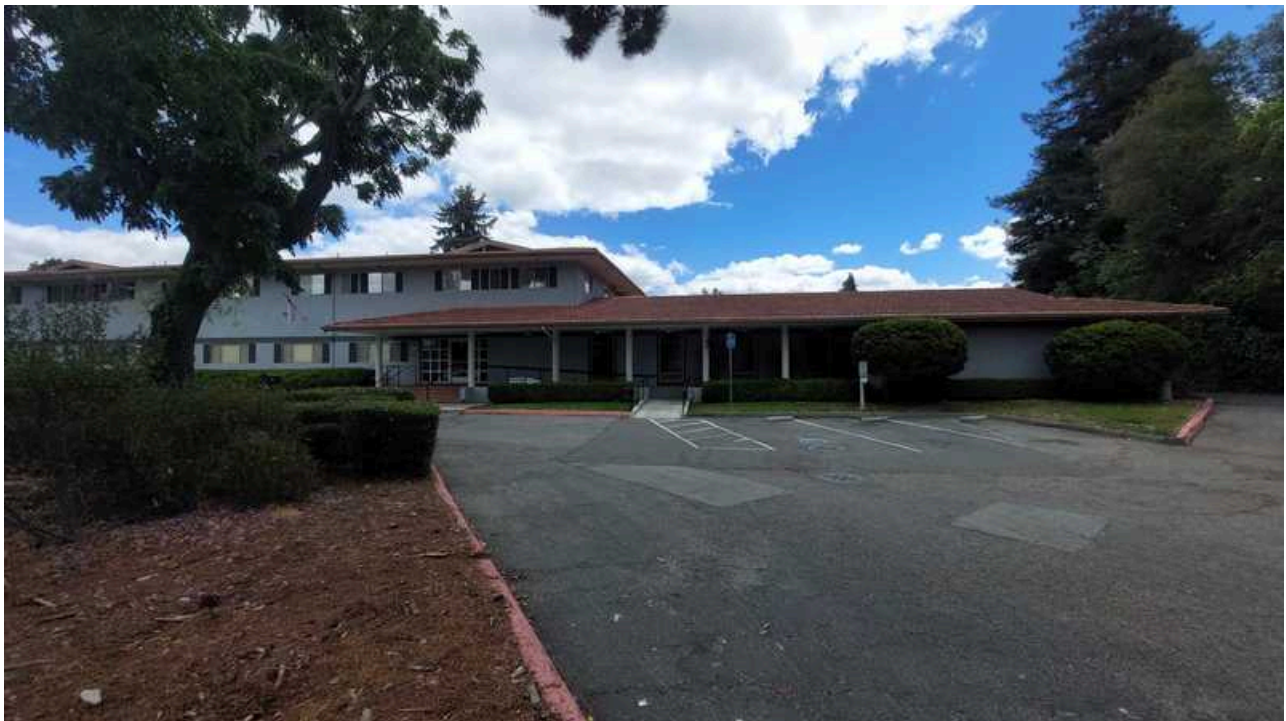
2. View of the subject property building, facing east
