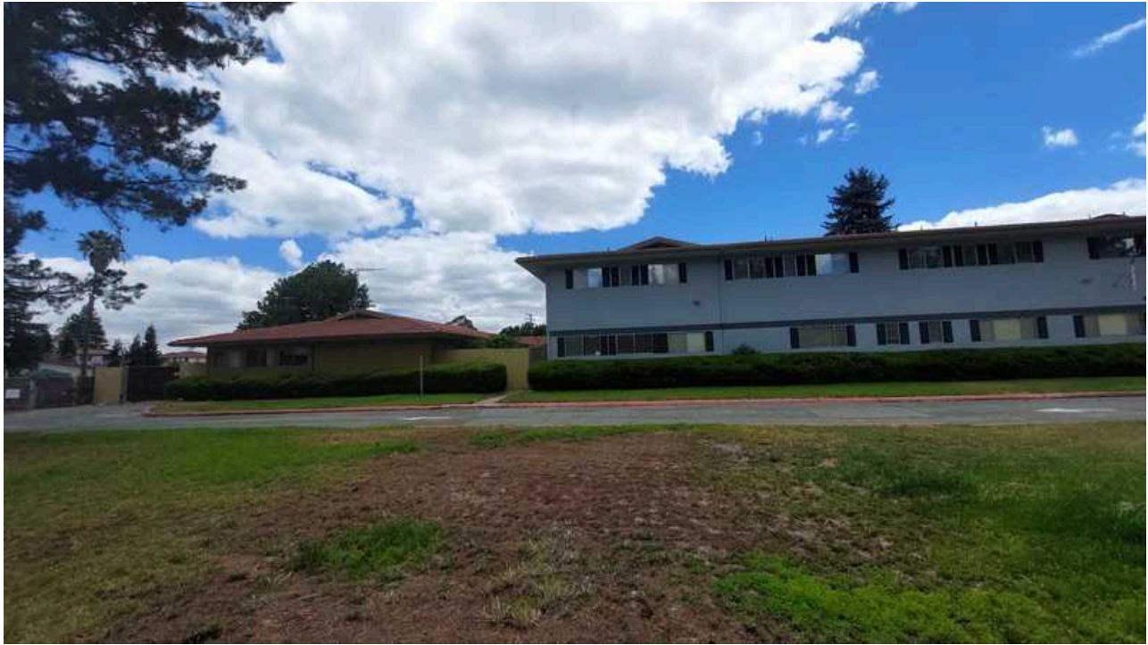
3. Additional view of the subject property facing east
