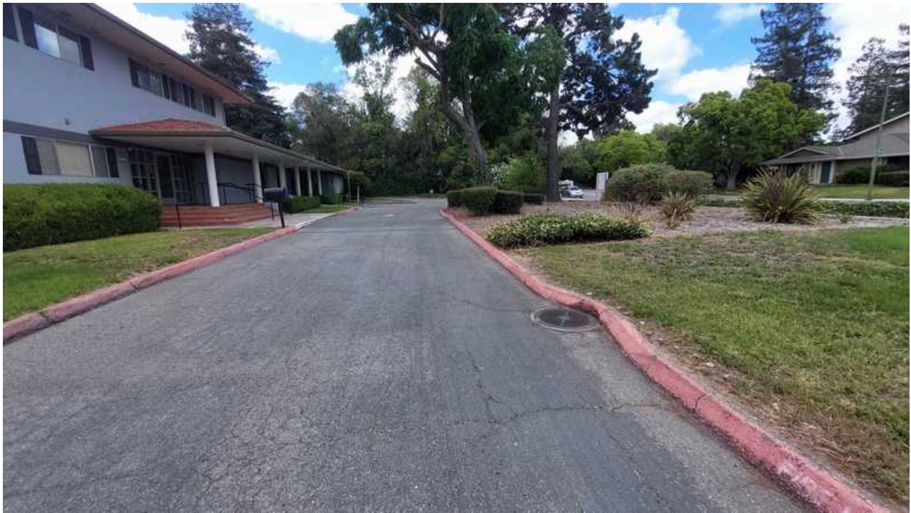
8. View of the eastern side of the subject property facing south
