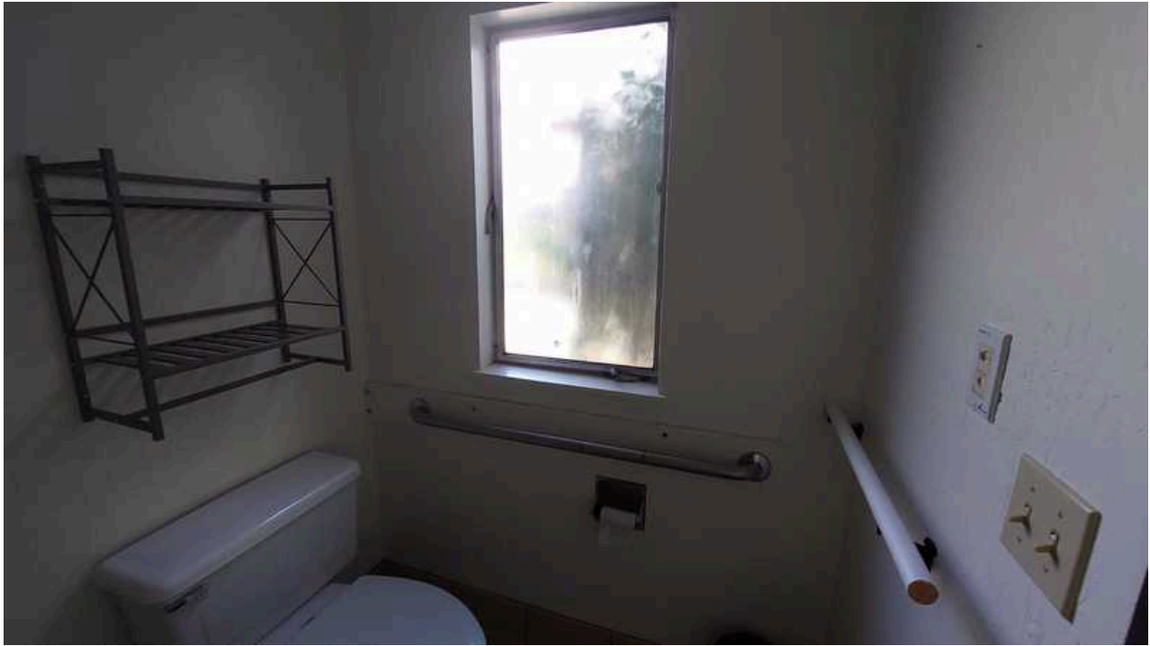
19. View of a typical attached bathroom
