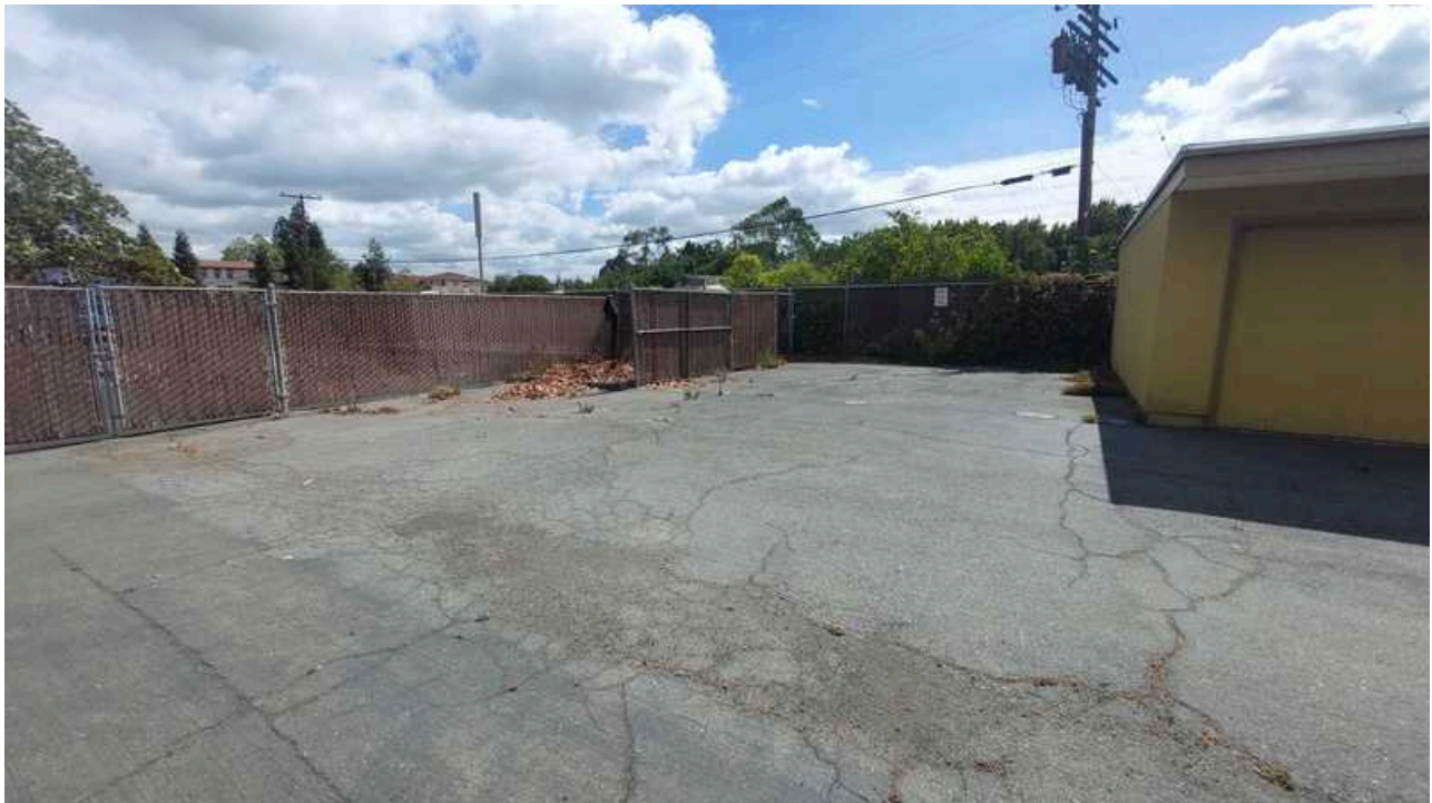
6. View of the parking lot of subject property, facing northeast
