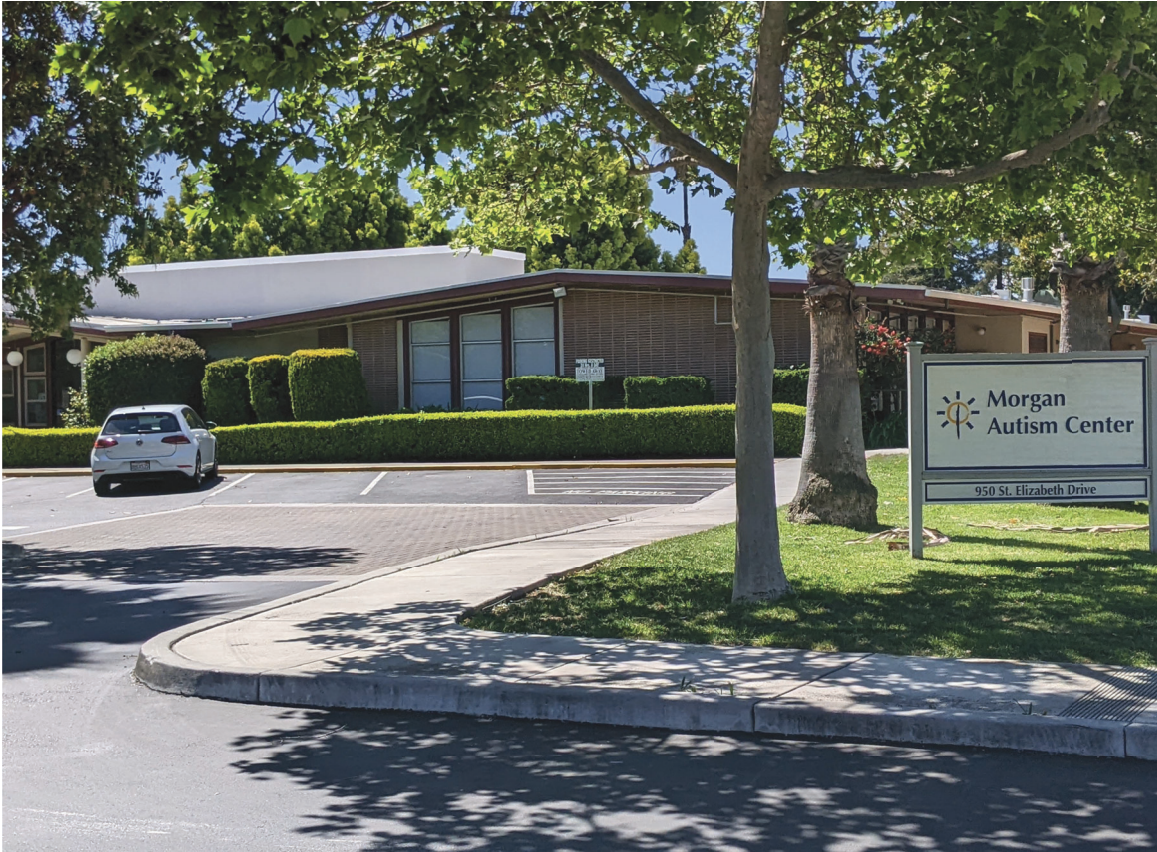
Photo 2: Adjacent One-Story School to the North.
