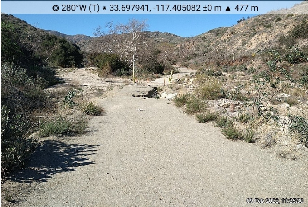
Image 1: View of the dirt access road and washed out creek crossing on the east end of the project site. RAFSS within floodplain and riparian forest on opposite side of the creek.
