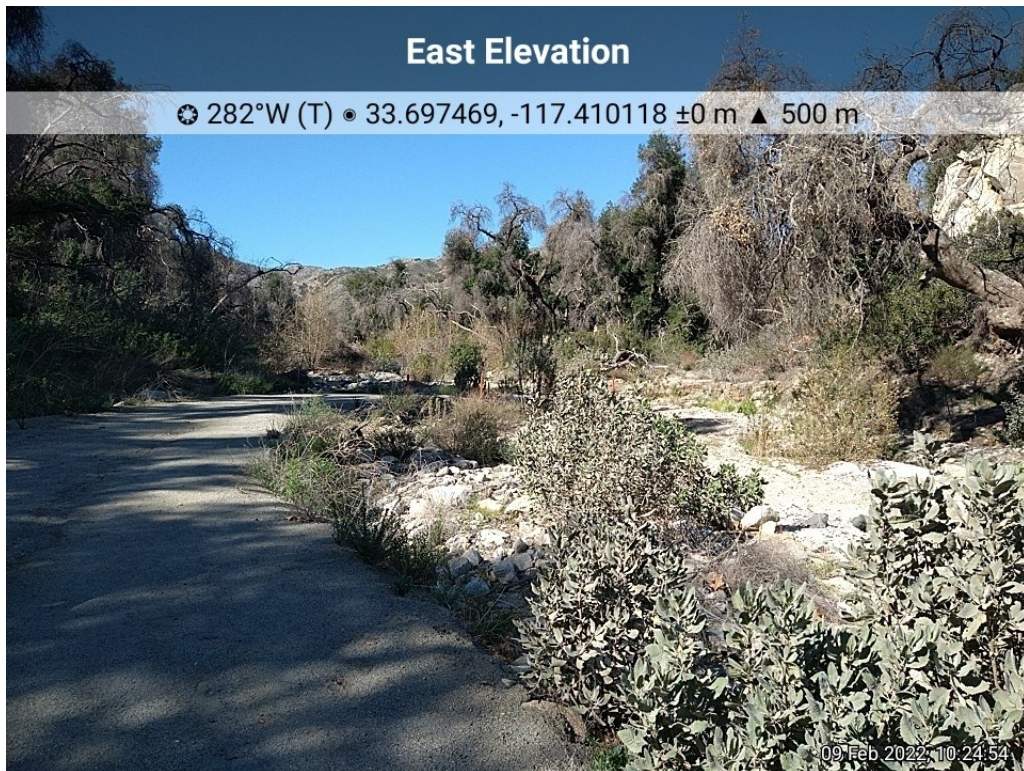
Photo 6. Depicts the third project crossing through Rice Canyon Creek on the west end of the project site.
